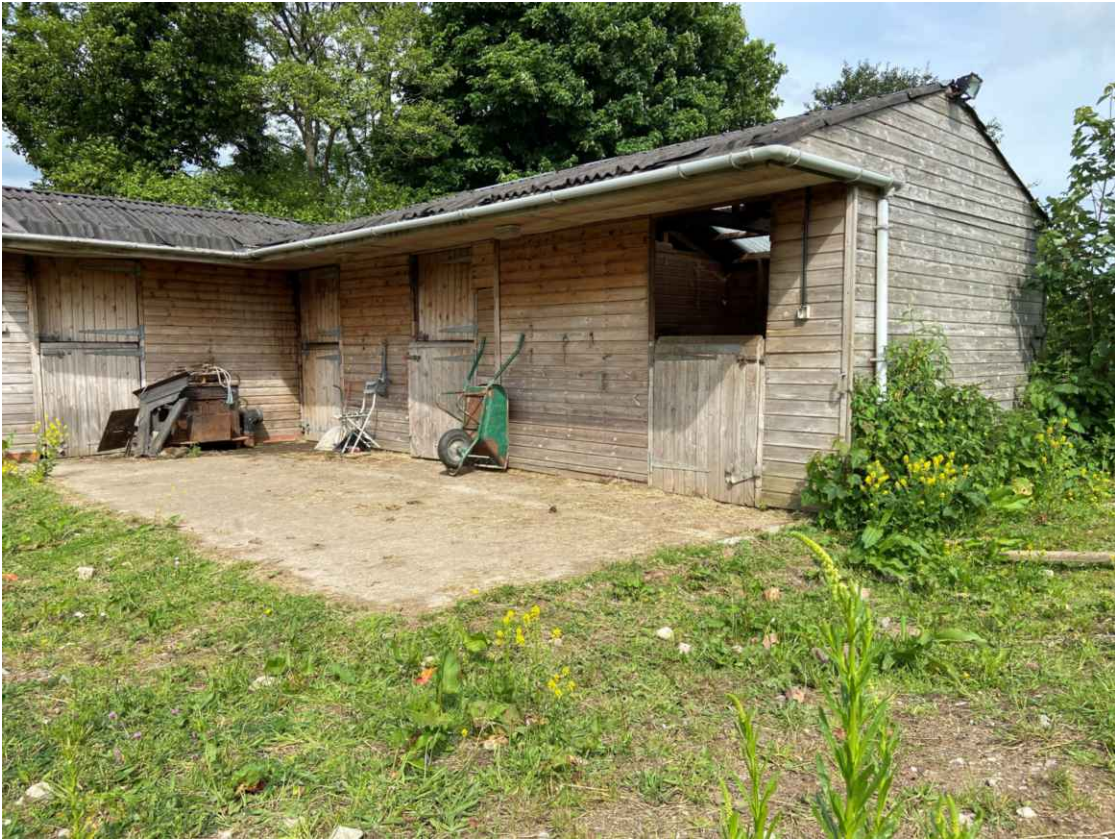
View 7 - View of existing stables to be utilised for bicycle storage.
