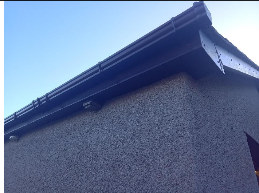
B1 – northern elevation – intact soffits/barge boards
