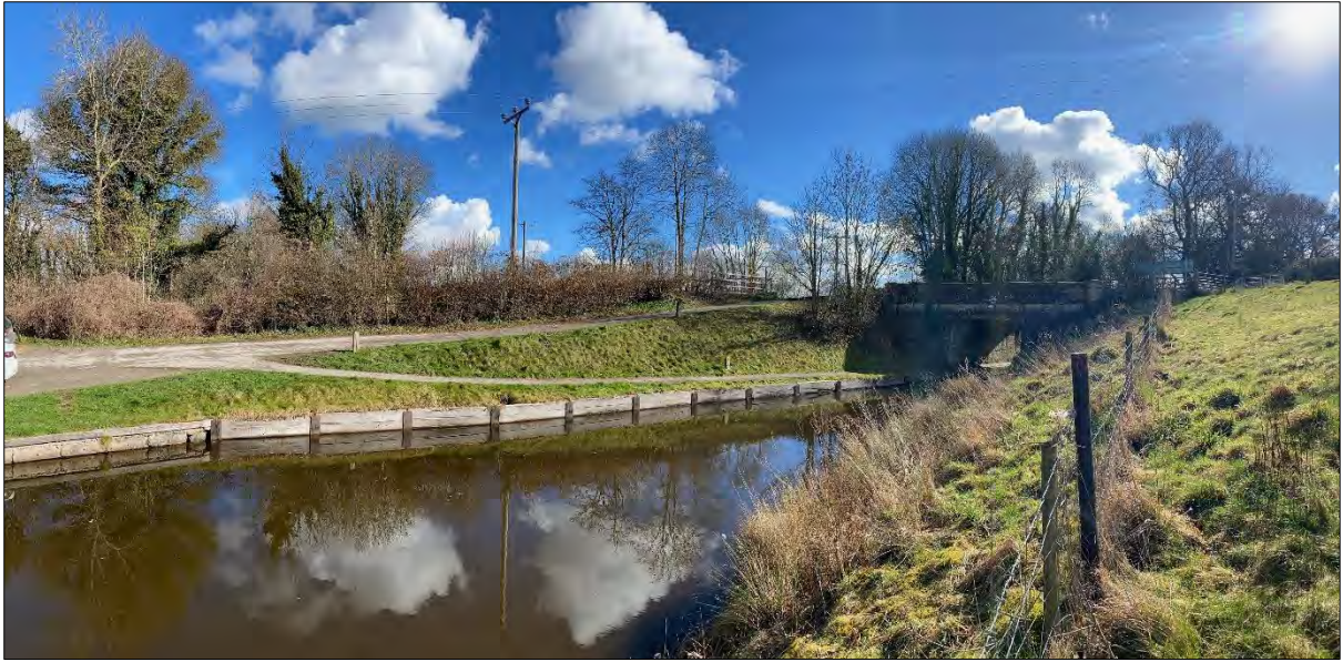
Plate 9. Irishman's Bridge (LB20214) and the Llangollen Canal (DE175). View to the east.
