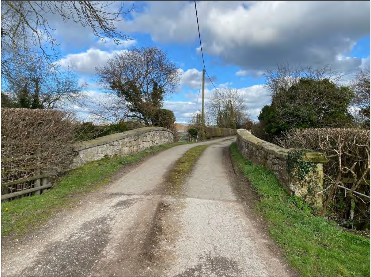
Plate 7. Whitehouse Bridge (LB87548). View to the east.
