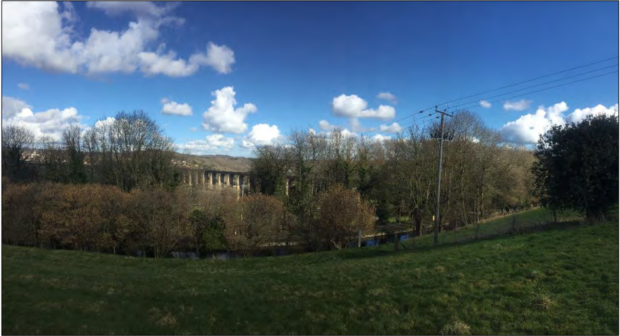
Plate 17. The course of DE138 running down to the Llangollen Canal (right) and DE140 beyond (left).
