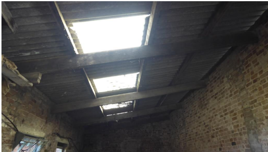
Figure 4.9. Internal view of building 3
