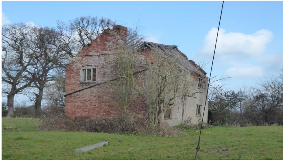
Figure 4.3. Building 1 from south in 2020
