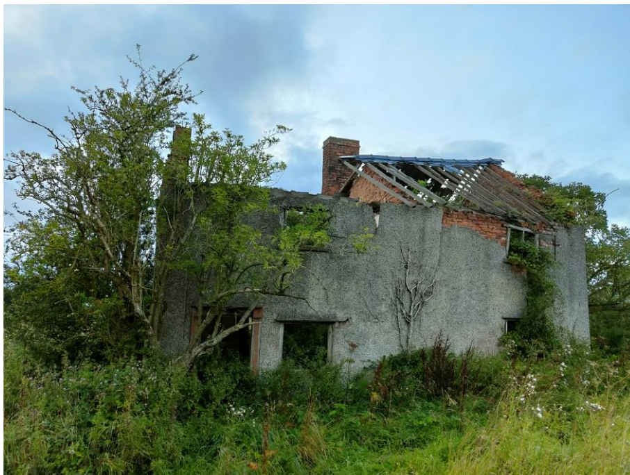
Figure 4.4. Building 1 from east in 2021
