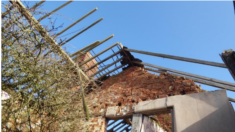
Figure 4.5. Internal view of building 1
