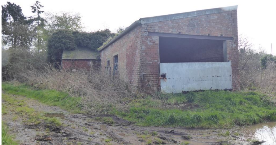
Figure 4.8. View of building 3 from northwest
