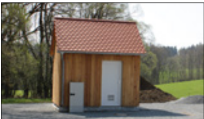
Example: Installation in a machine house
