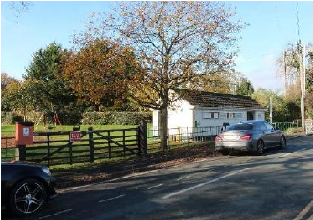
Image 1. Existing Toilet Block
