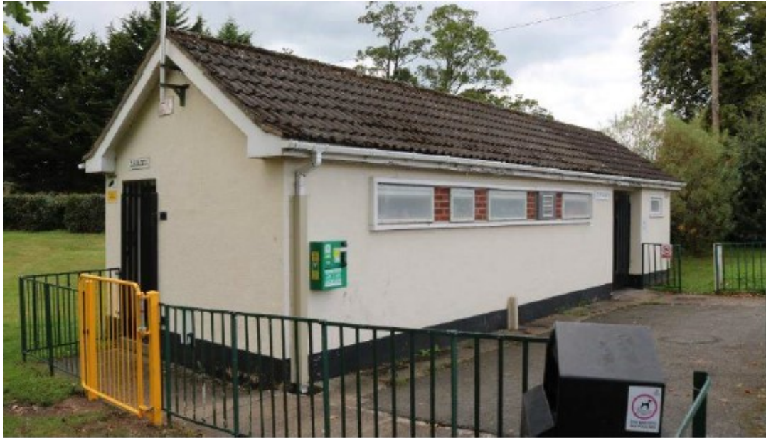
Image 2. Existing Toilet Block
