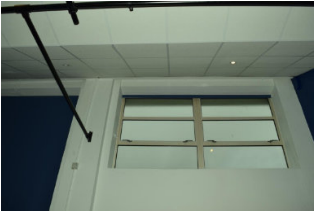
Figure 246 SU R28 NE elevation, southern end High level window above emergency exit.
