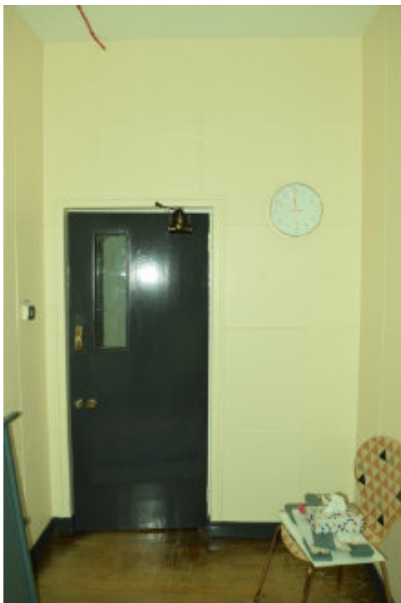
Figure 213 Passage, original door to R7.
