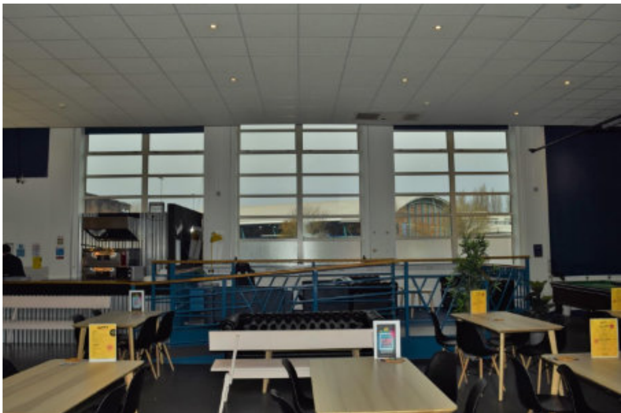
Figure 245 R28 NE elevation windows.
