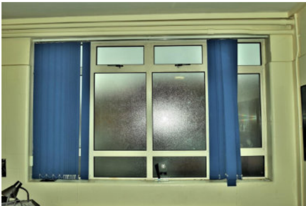
Figure 191 SU R2 SW elevation window (over-painted tiled wall surround).
