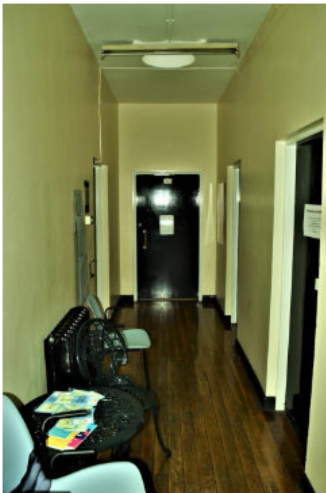
Figure 205 SU Access passageway to R8 - R11 (door to R11 at far end) View SE.
