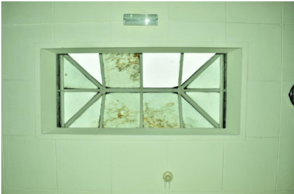
Figure 204 SU R7 Rooflight.
