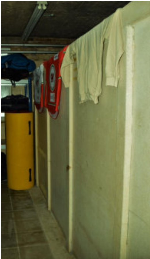
Figure 228 SU R17 Central partition with doorways at both ends.
