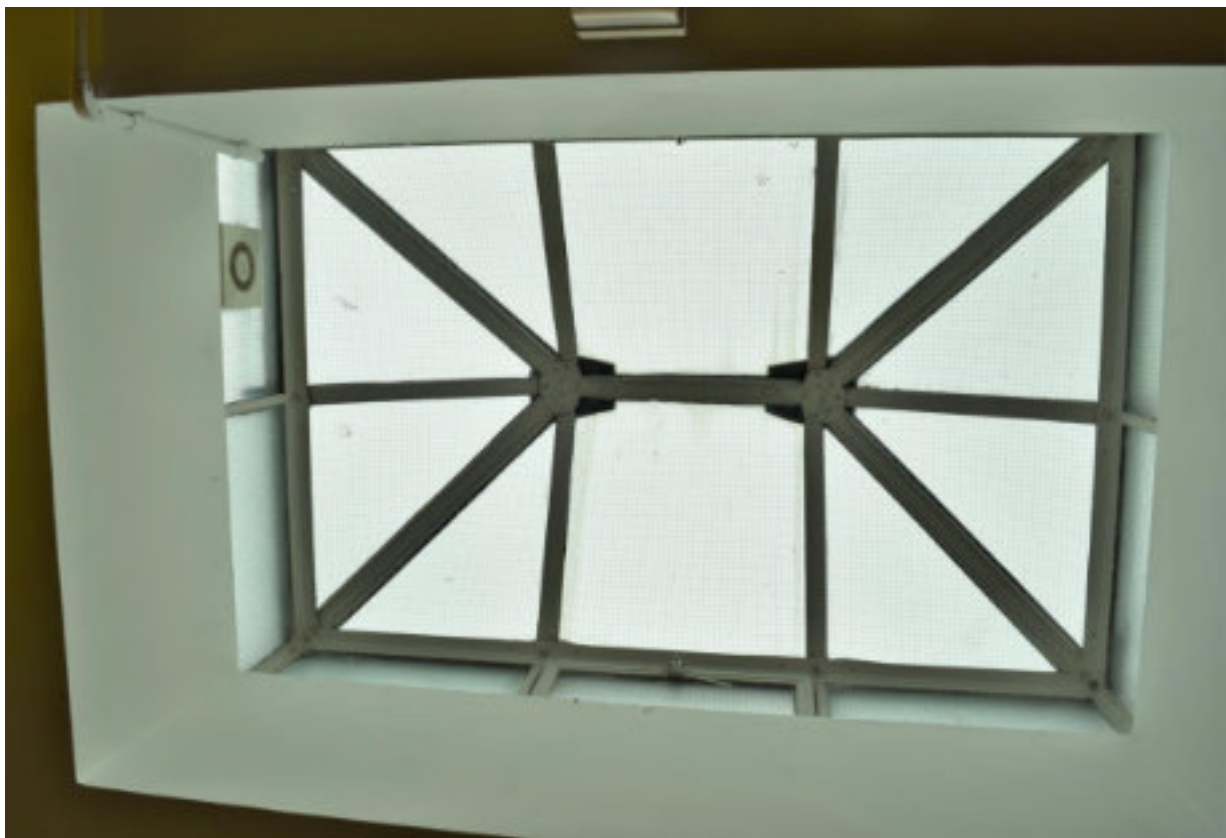
Figure 187 SU R1 Skylight.
