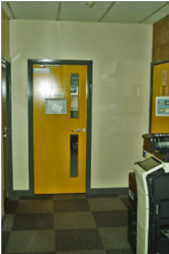
Figure 144 R 16NE elevation with door to R 16b.
