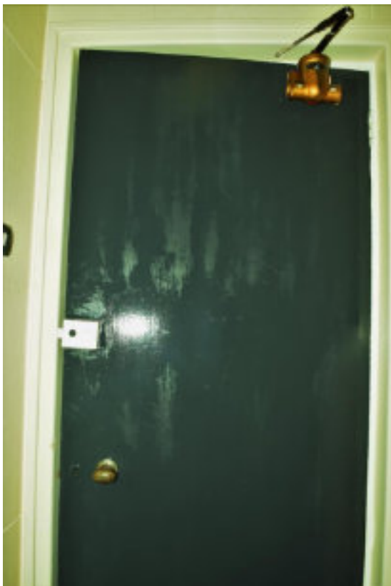
Figure 211 SU Rooms typical door furniture detail with closer, copper alloy door knob, mortice lock keyhole and modern lock.
