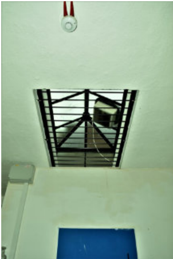
Figure 224 SU R16 Rooflight.
