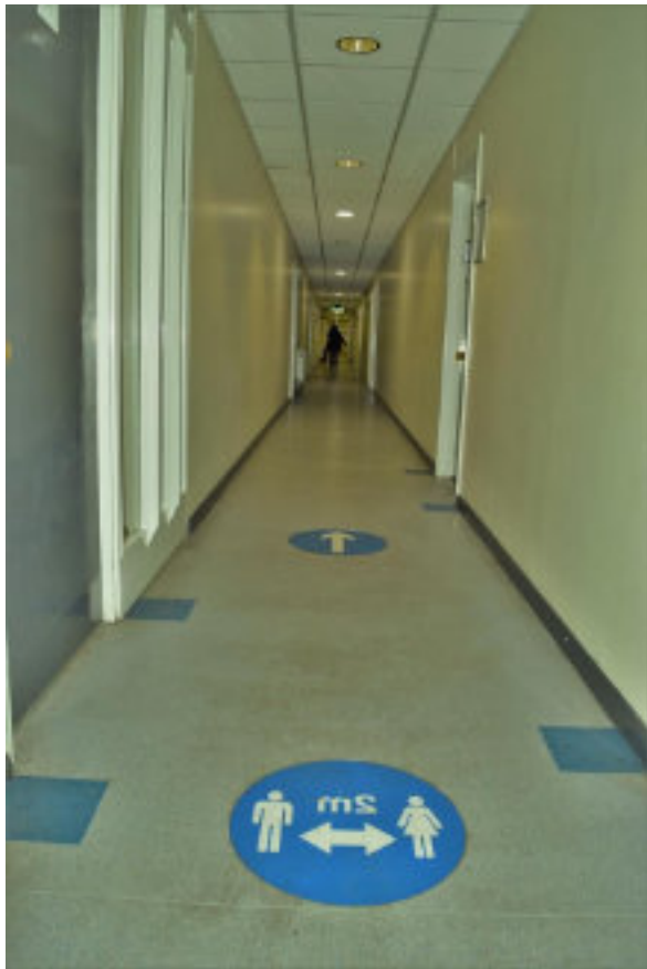
Figure 156 D block View SE down main corridor.
