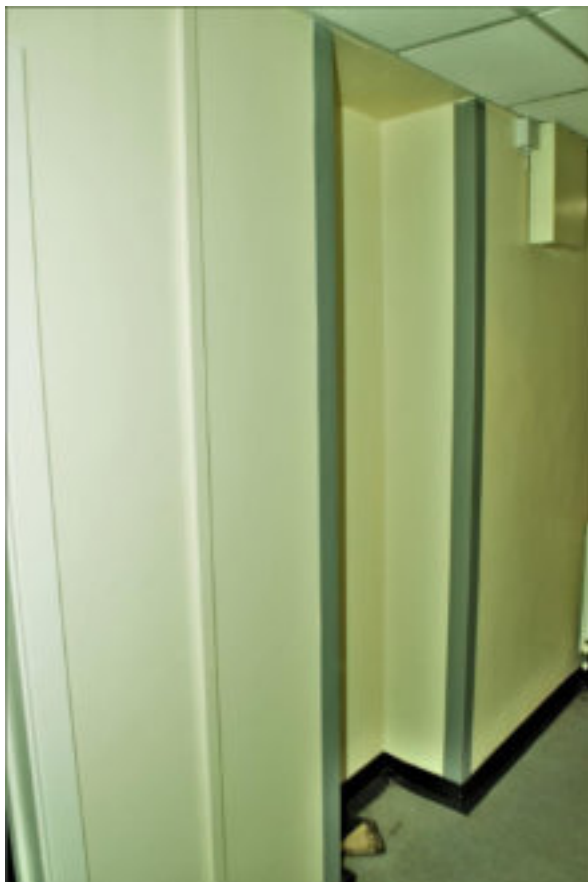
Figure 182 Vertical recess SW side of corridor, S end of exterior of R 15
