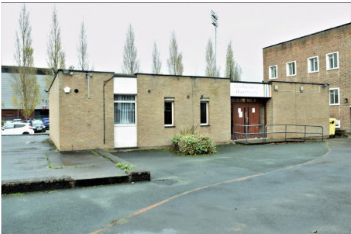
Figure 253 Building 3 on Fig.6 Medical Centre NW elevation.
