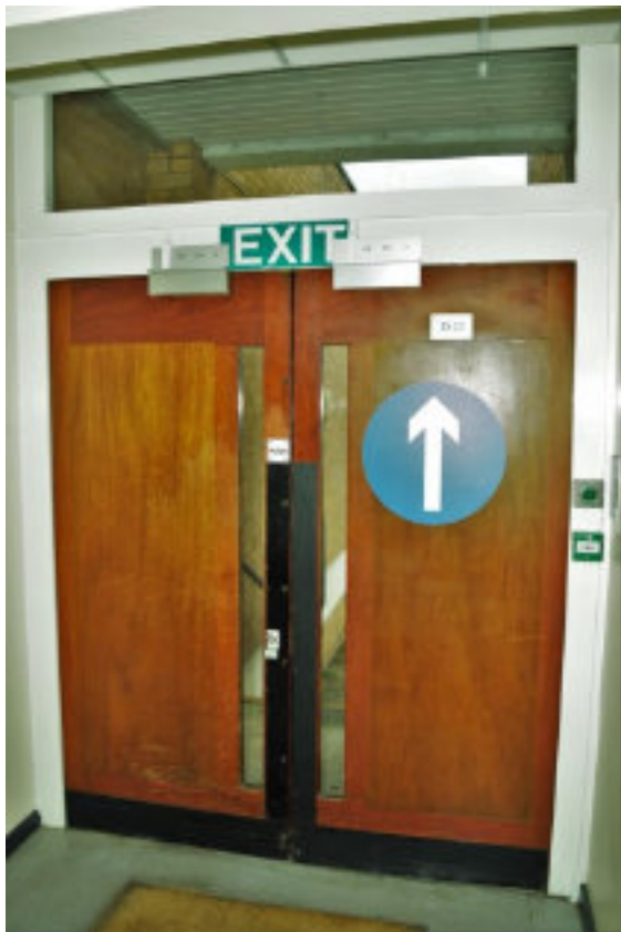
Figure 152 Corridor NE elevation outside R 26, recess in wall.
