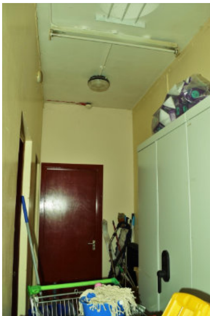
Figure 203 Passage between R7 and R3 from R7 (view to NW).
