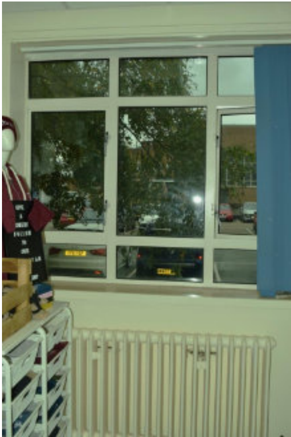
Figure 194 SU Reception and shop SW elevation window.
