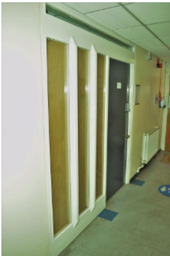
Figure 159 R 29 Door and glass panels in wall looking into corridor, from E.
