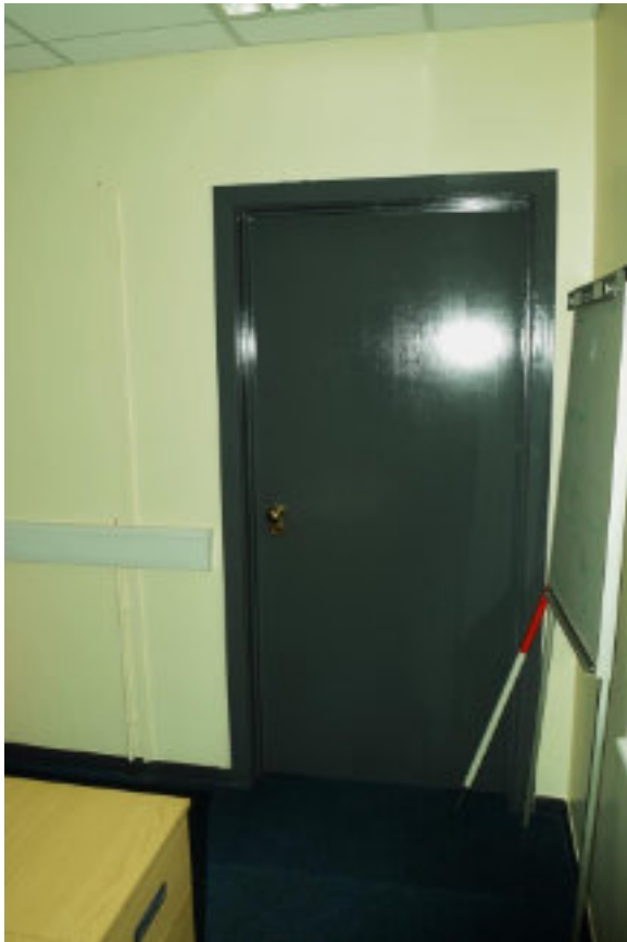
Figure 129 R 12 NW elevation Door to R 14.
