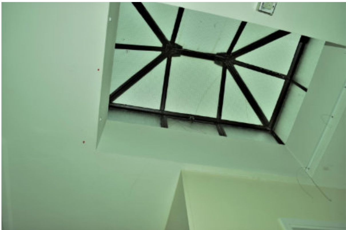
Figure 239 SU R22 Rooflight.
