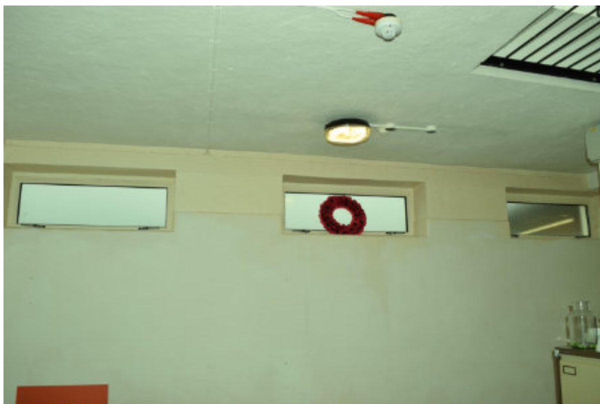
Figure 223 SU R16 Windows in NE elevation.
