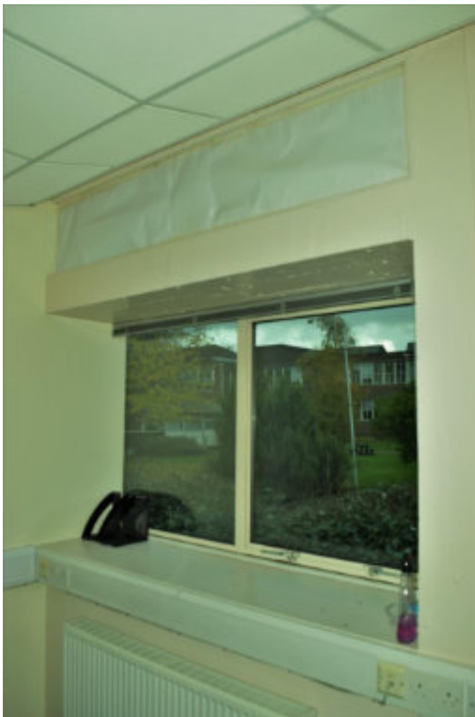
Figure 180 R 15a SW elevation window detail, oblique view, note covered horizontal strip window above main window.
