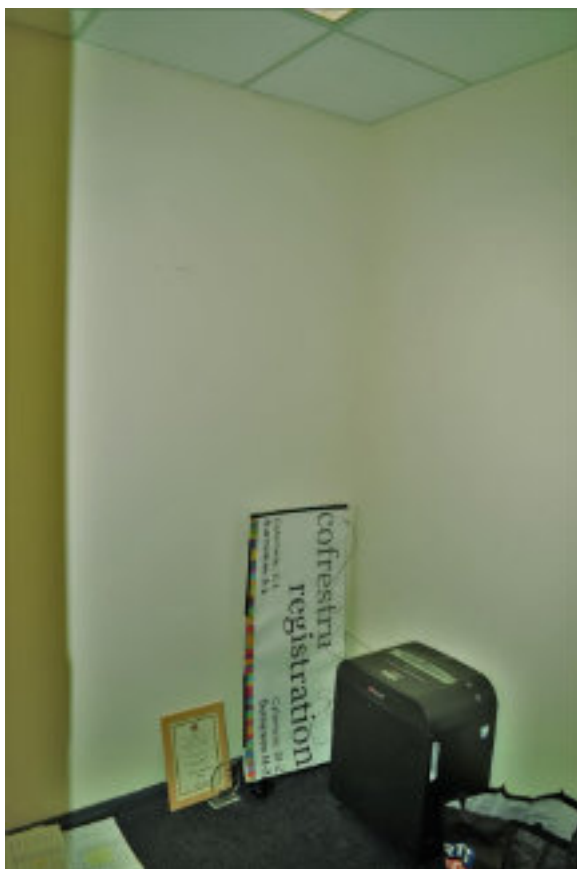
Figure 153 Small sample of equipment and materials found in stores and corners of offices.
