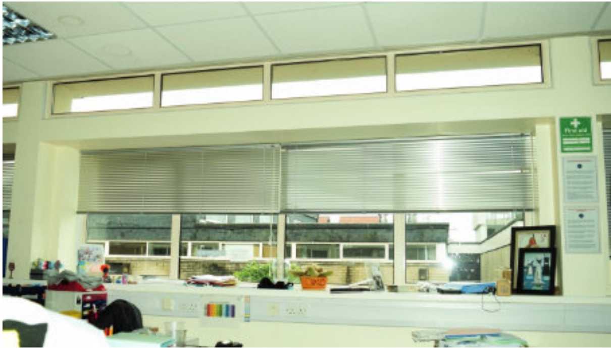
Figure 138 R 14 NE elevation window detail.
