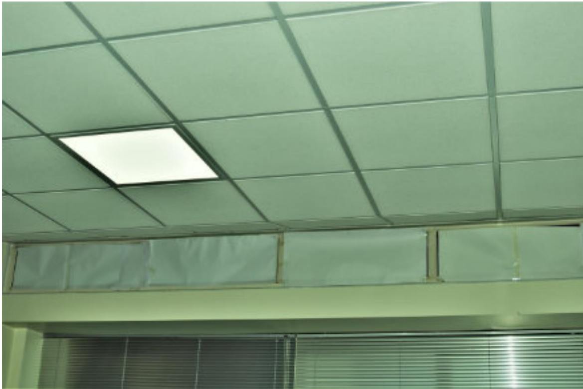
Figure 125 R 11 SW elevation wall top windows (covered) and ceiling with light fitting detail.
