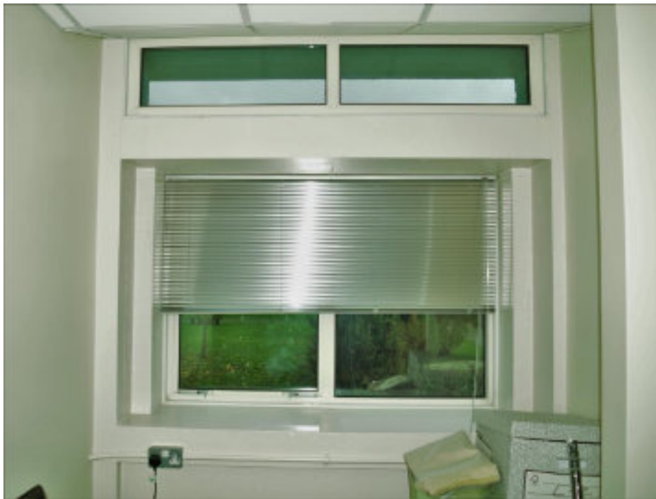
Figure 131 R 13 SW elevation window. Strip window panes at top is a regular design feature.
