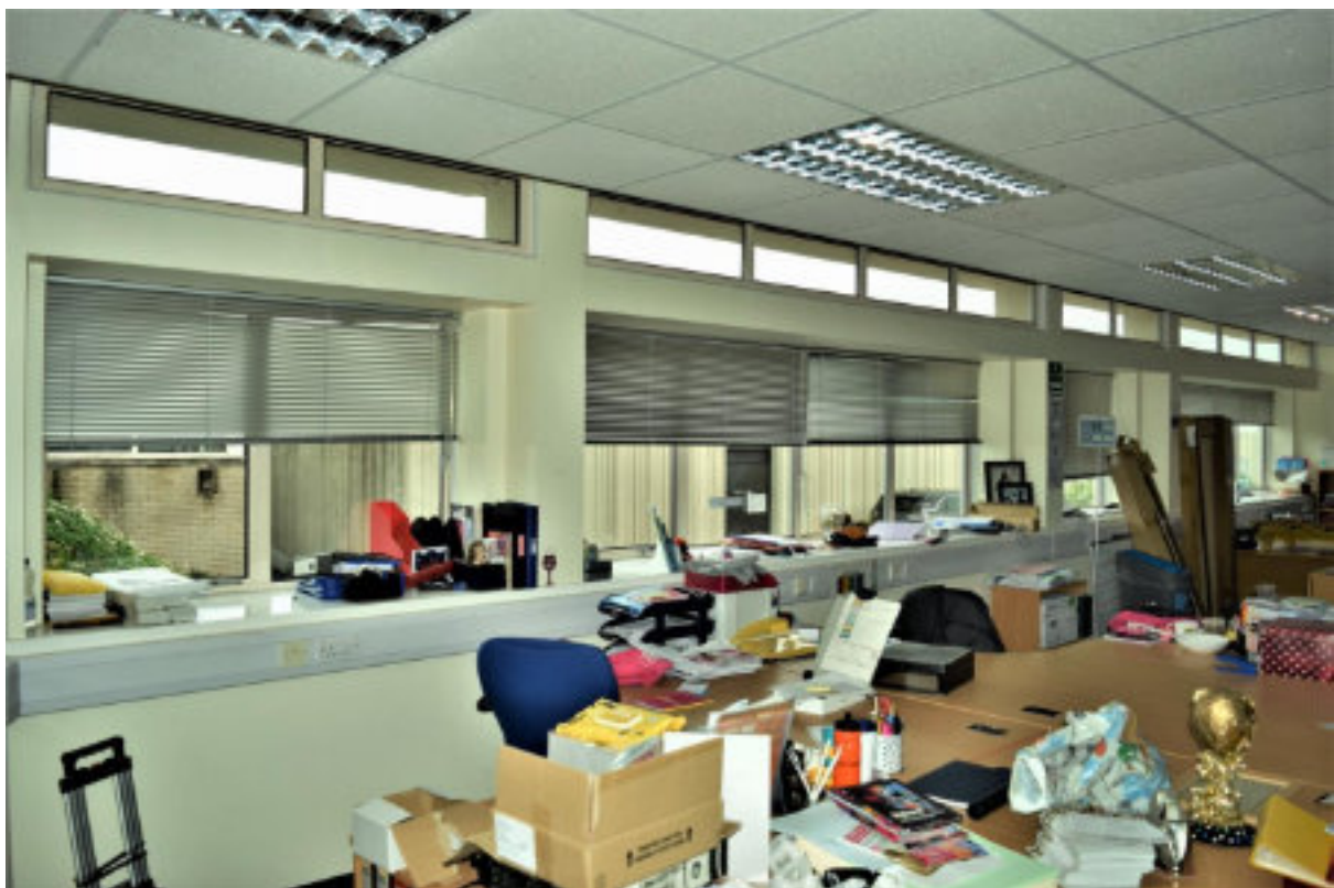
Figure 137 R 14 view along NE elevation from NW.
