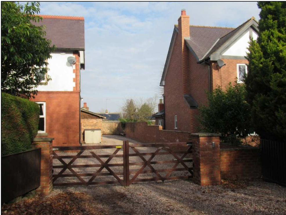
Plate 6 – View through the conservation area where solar panels are visible.
