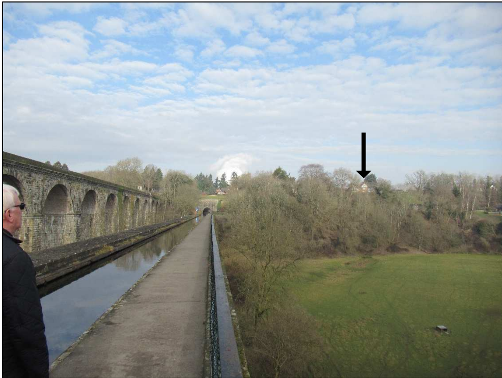
Plate D – View north along canal across the aqueduct; Glyn Wylfa house just visible to the right of centre above the tree line of the wooded valley side
