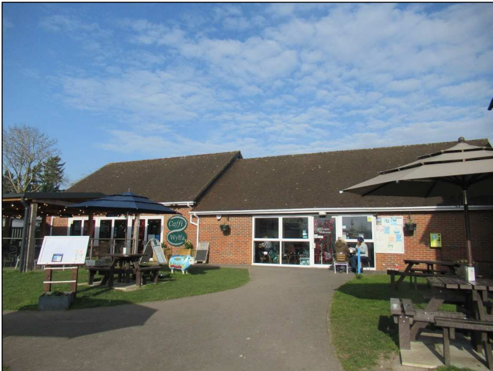
Plate 8 – South elevation of Caffi Wylfa
