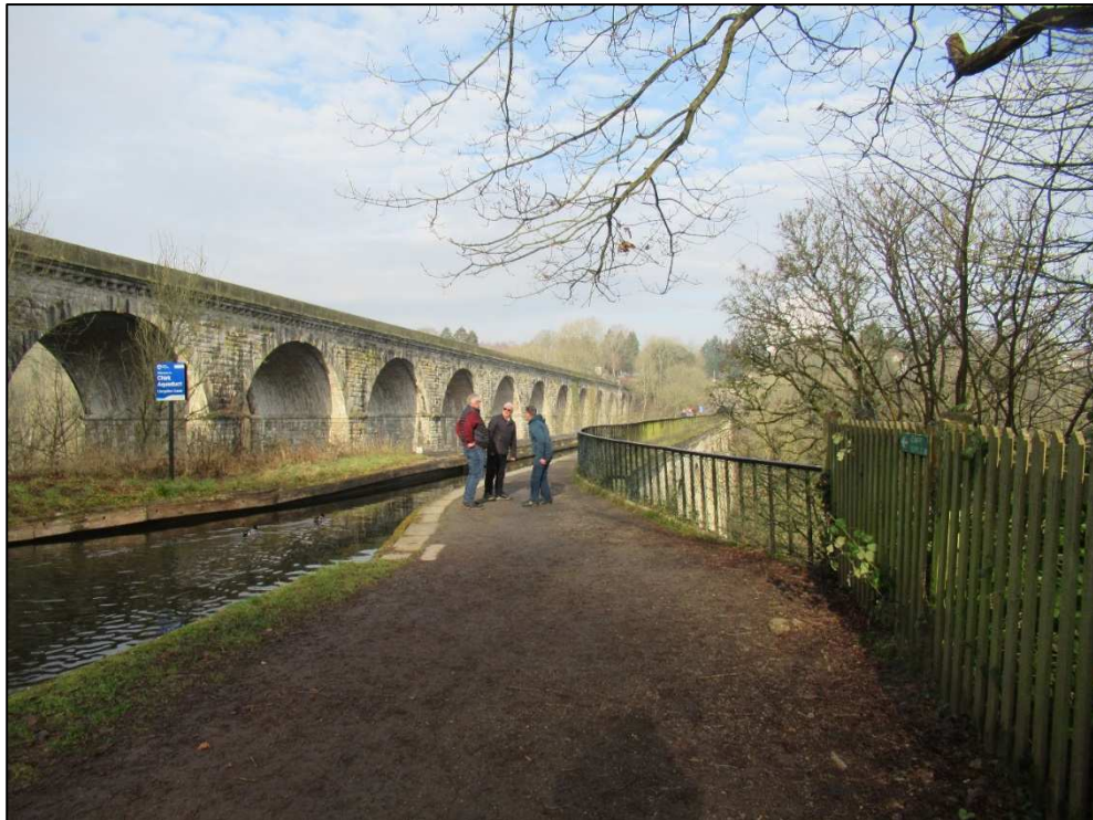
Plate 3 – View along the canal from Chirk Bank; Caffi Wylfa not visible
