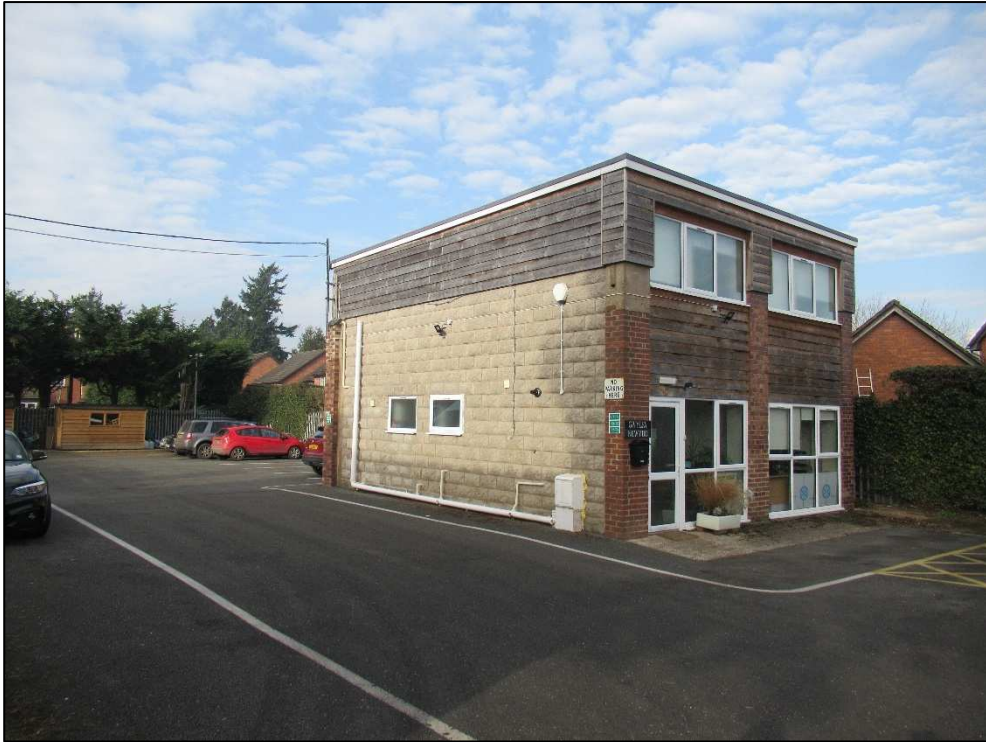
Plate 11 – Altered, modern outbuilding to the north of the Glyn Wylfa site.
