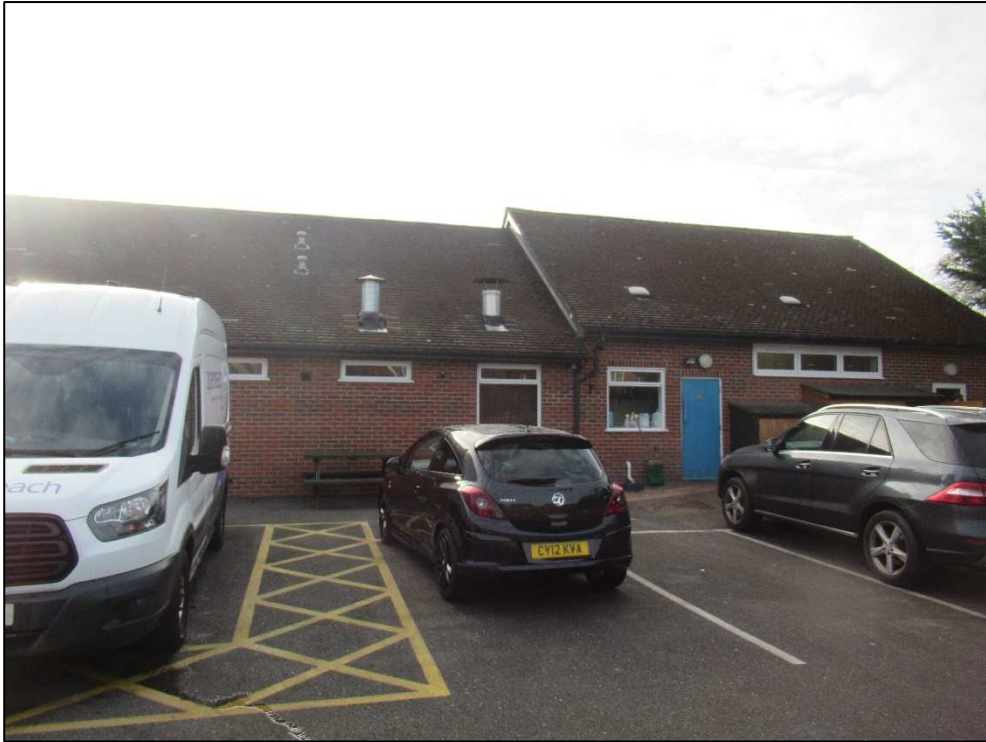
Plate 9 – North elevation of Caffi Wylfa
