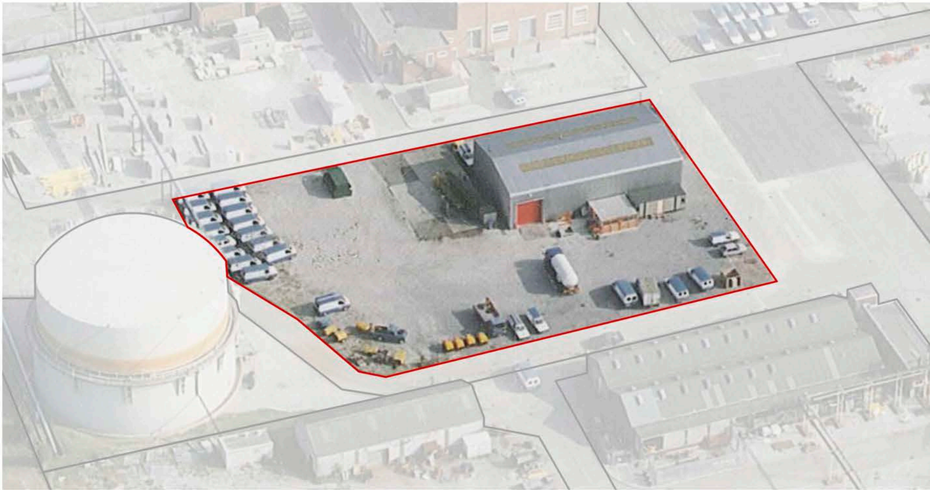
Garage - highlighted aerial image
