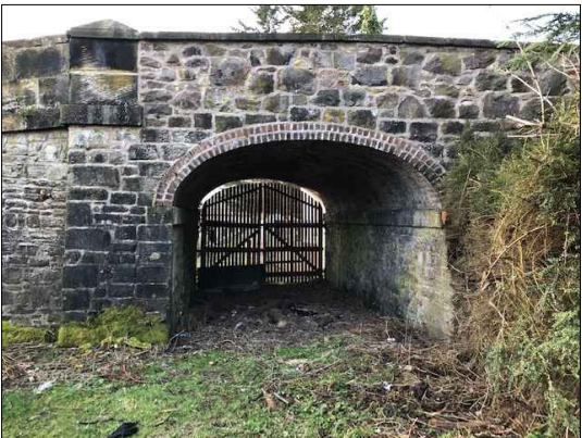
Above; photograph of existing north facing elevation, note that the proposed gate is within the west arch of the north side of Scotch Hall Bridge only.
