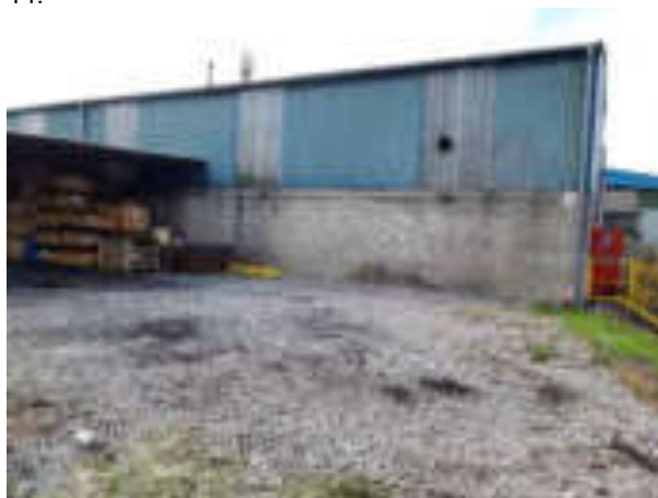
13.09.22 – View west from northeast corner
