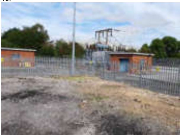
13.09.22 – Northeast corner with off-site substation
