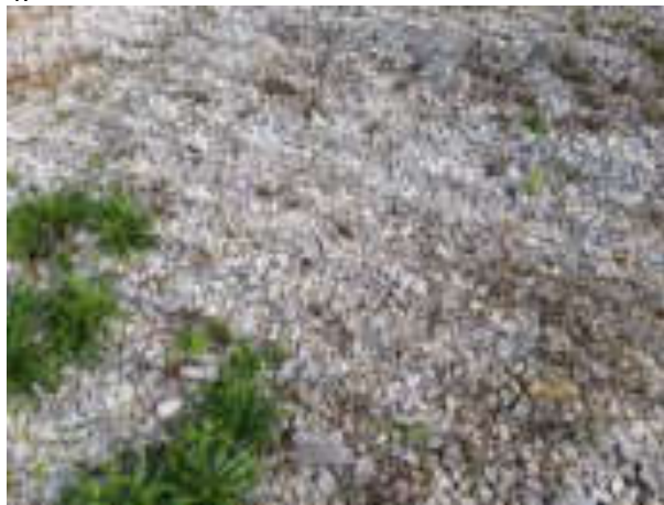
13.09.22 – Southern half of the site surface
