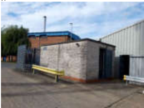
13.09.22 – View of small brick office.
