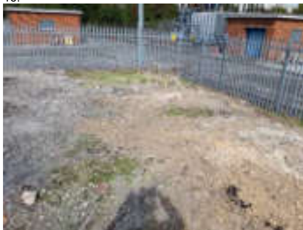
13.09.22 – Northeast corner surface
