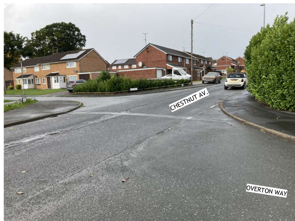
VIEW FROM OVERTON WAY LOOKING NORTH UP CHESTNUT AV.
