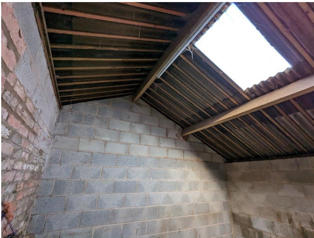
Plate 6 – Interior of the stables block adjacent to the application site
