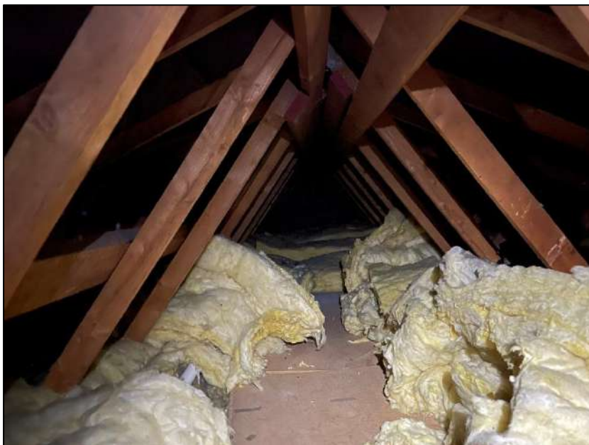
Photograph 14 showing the roof void above the single-storey part of the dwelling
