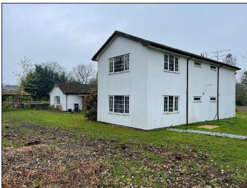
Photograph 10 showing the front of the dwelling
