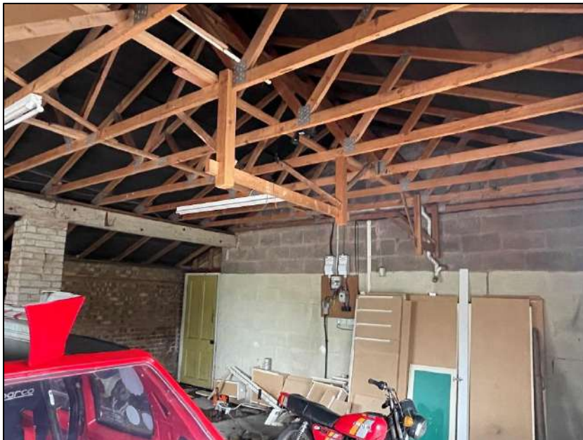
Photograph 16 showing the interior roof of the garaging
