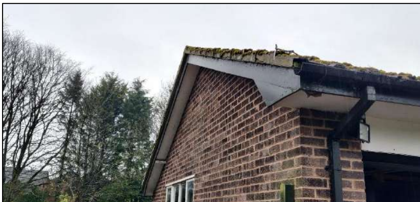
Photograph 12 showing the roof edge at the garage
