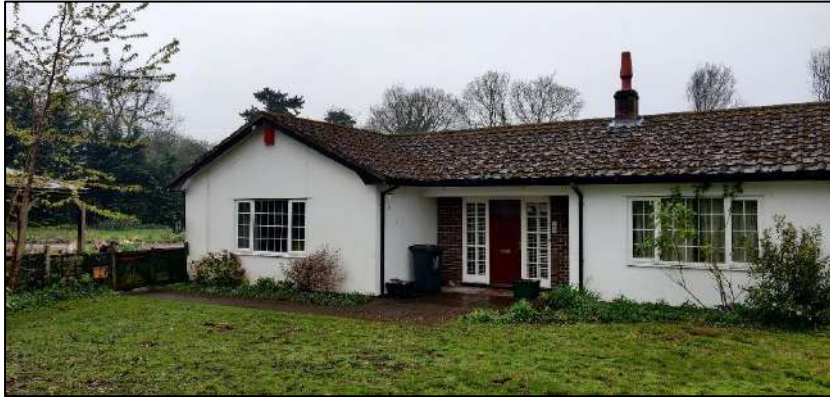
Photograph 10 showing the roof at the front of the dwelling
