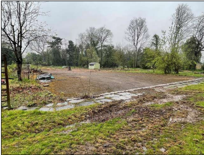
Photograph 1 showing the hardstanding at the tennis court
