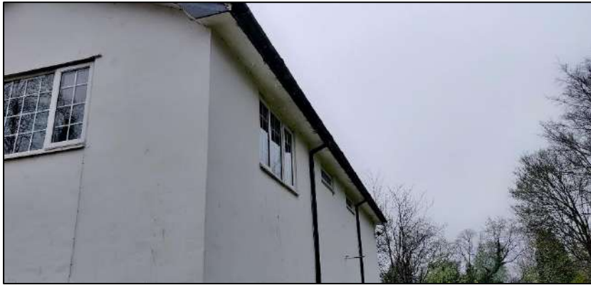
Photograph 13 showing the soffits at the two-storey section
