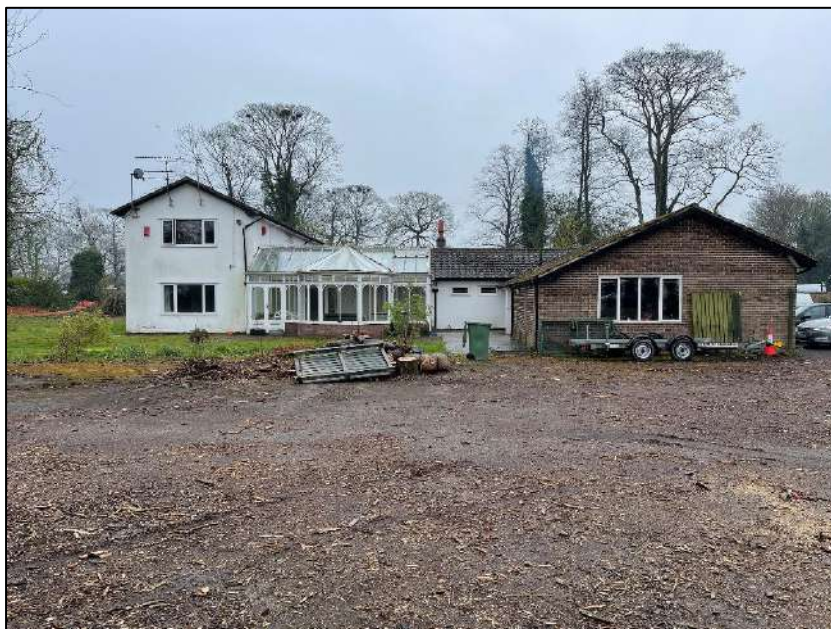
Photograph 8 showing the exterior of the dwelling at the rear
