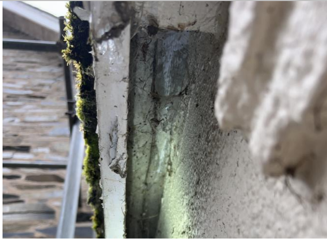
1970's lean to eaves
