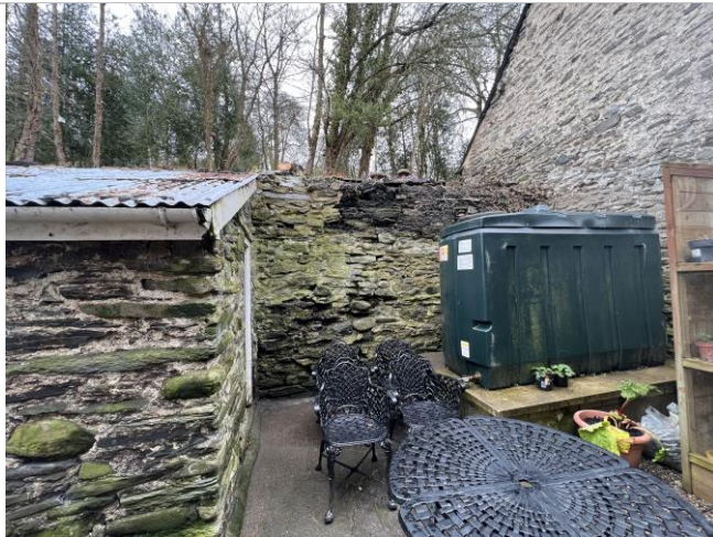
Stone retaining wall
