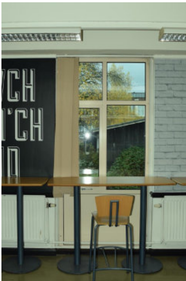
Figure 69 Restaurant NW area SW elevation window detail.
