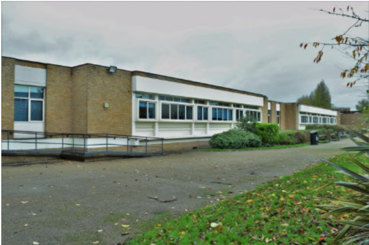
Figure 26 D Block SW elevation from NW.
