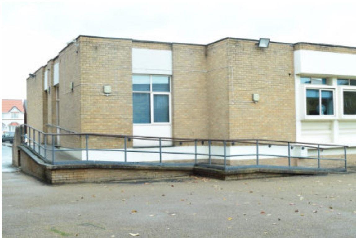
Figure 25 D Block SW elevation ramp to entrance door in NW elevation.
