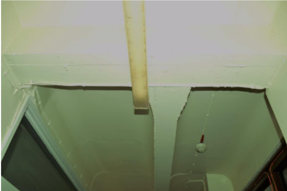
Figure 96 Service corridor NW end ceiling detail view to SE.
