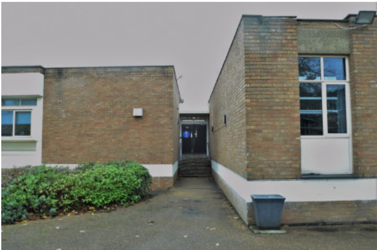
Figure 35 Door to link between Refectory (R) and D Block (L).
