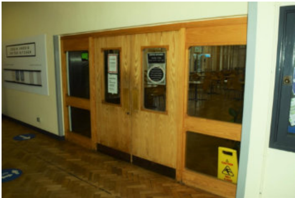
Figure 55 Refectory Entrance from main corridor.
