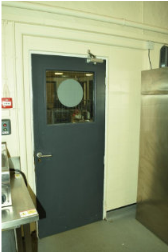
Figure 106 Kitchen, SW elevation Door to north end of servery area.
