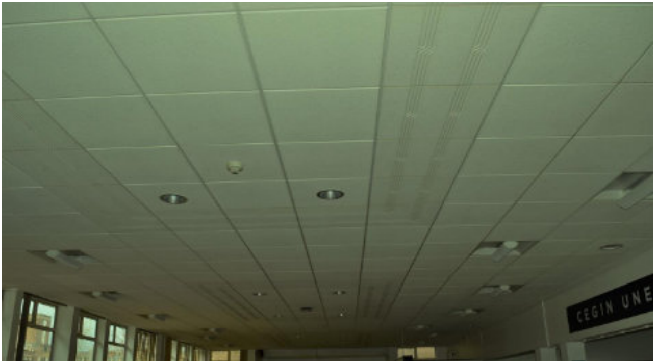
Figure 84 Restaurant SE section, ceiling with grooved decorative details in tiles, from SE.
