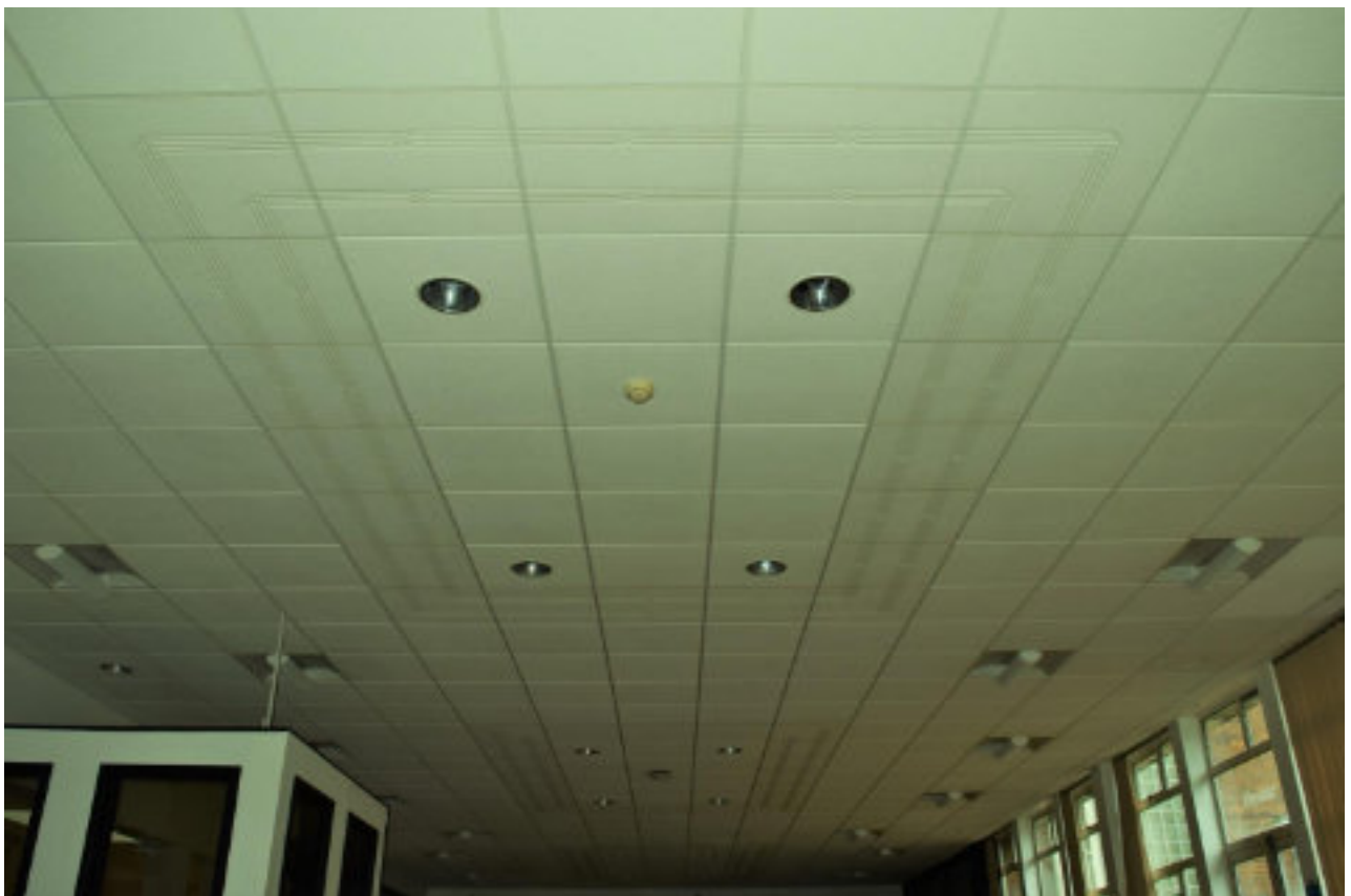
Figure 85 Restaurant SE section ceiling with grooved decorative detailing, from NW.
