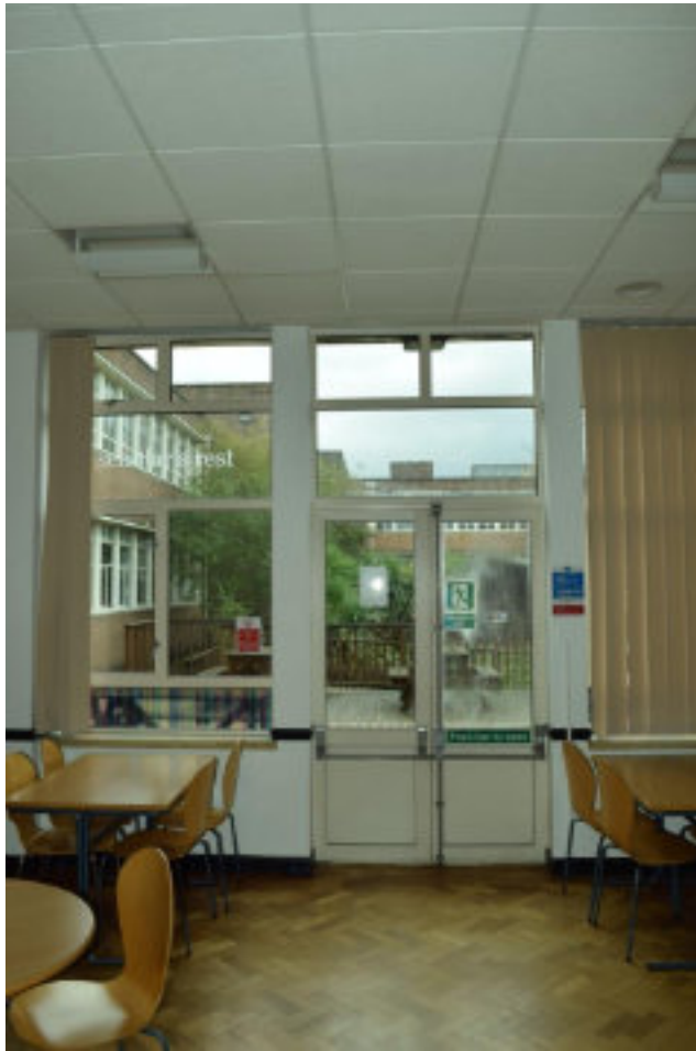
Figure 82 Restaurant windows on SW elevation of SE section. Note window on R, on stub that divides parts of restaurant.
