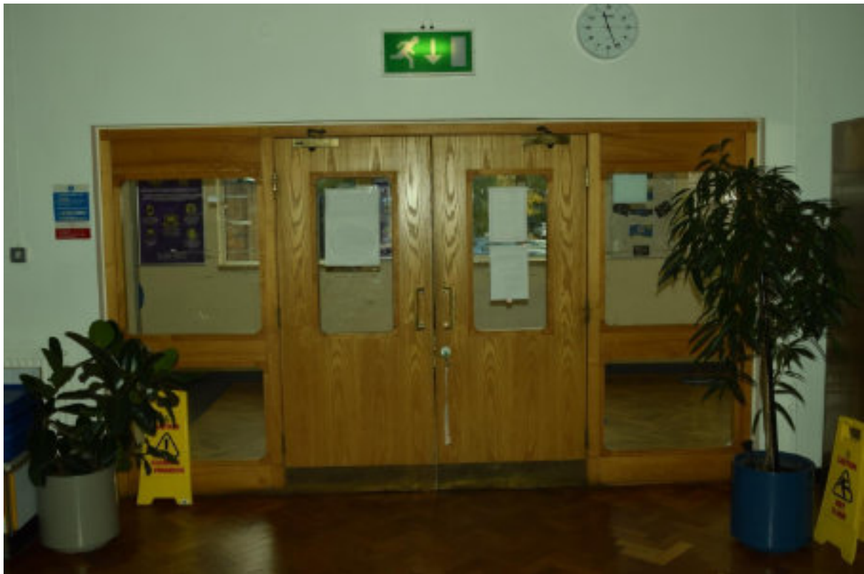
Figure 76 Main entrance doors, detail.
