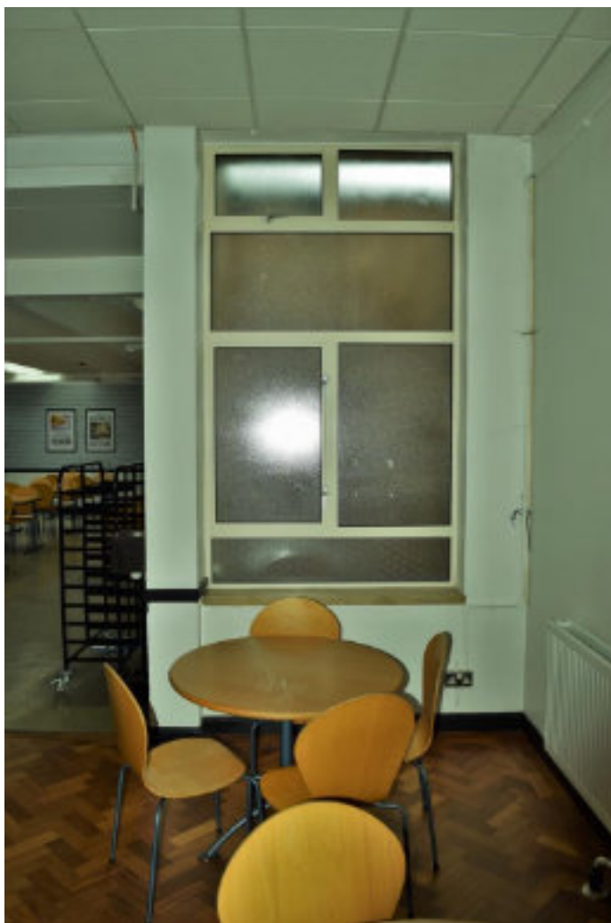
Figure 73 SW stub dividing areas of restaurant, window in SE elevation.
