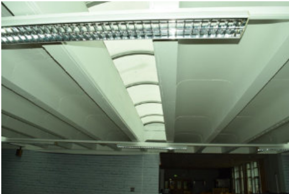
Figure 62 Refectory restaurant, NW section skylight details view SE.
