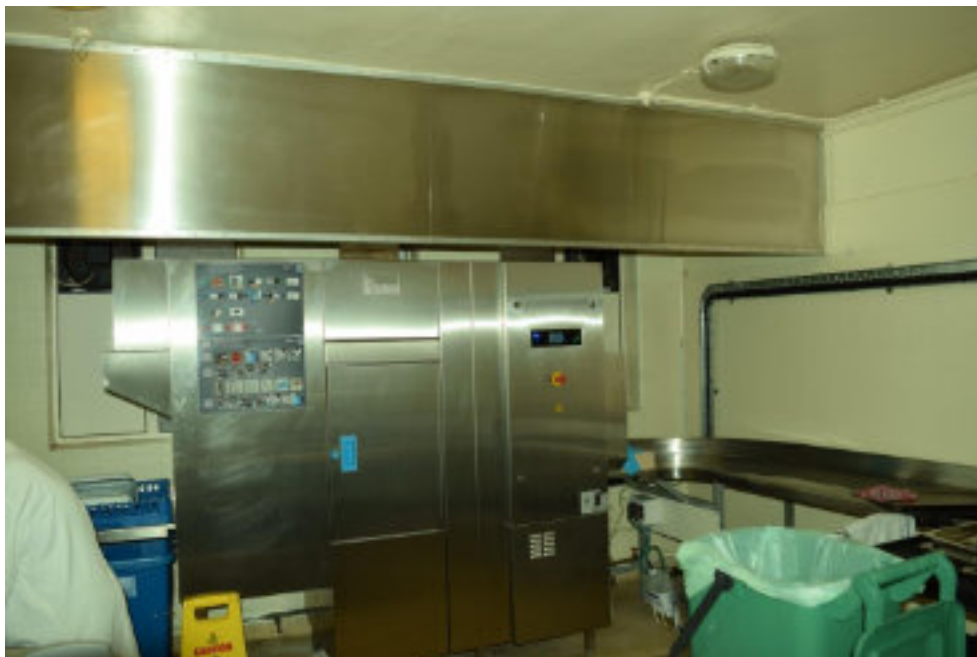
Figure 91 NW elevation of wash up.
