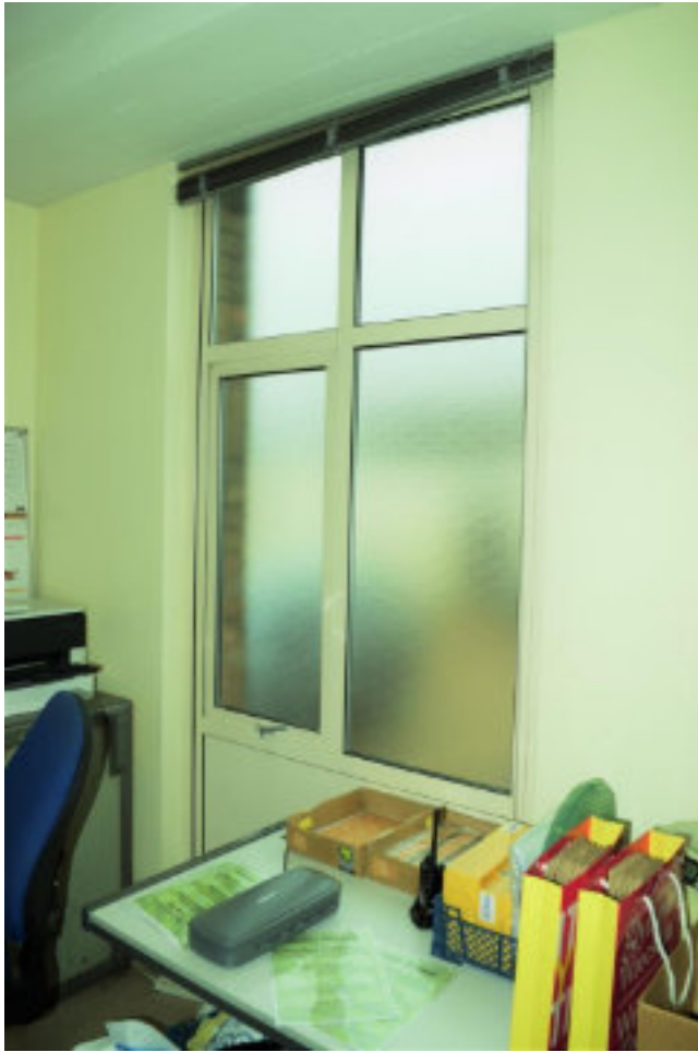
Figure 112 Service corridor, Managers office, N end of corridor, NE elevation.
