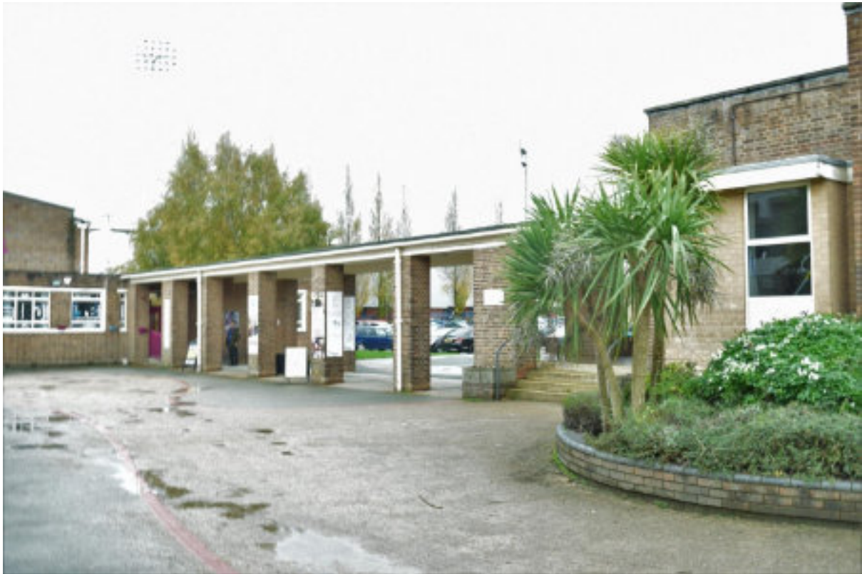
Figure 39 Walkway between Refectory (R) and SU building (L).
