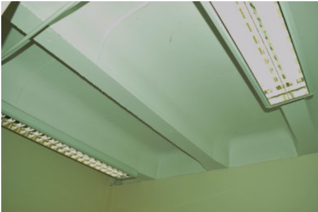
Figure 113 Service corridor, NE side Manager's office, N end of NE side of corridor, ceiling detail.
