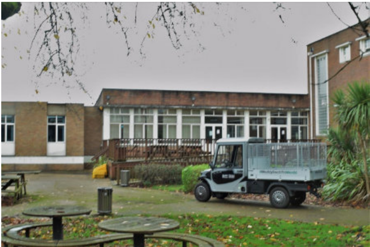
Figure 33 Refectory dining room, SW elevation.
