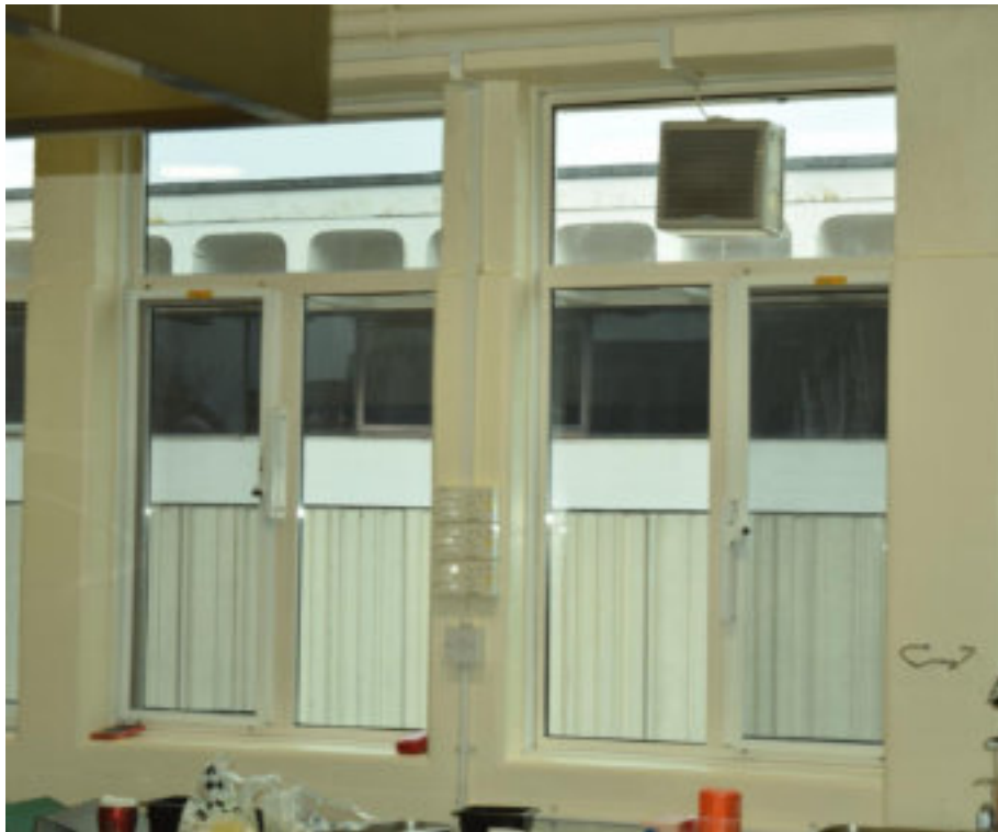
Figure 104 Kitchen SE elevation window detail, alternate top panes have extractor fans.
