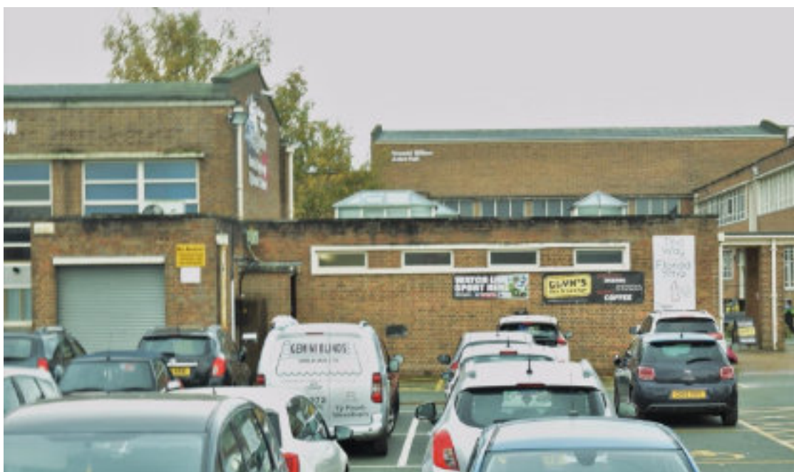
Figure 52 SU NE elevation Northern goods loading bay and northern section of elevation.
