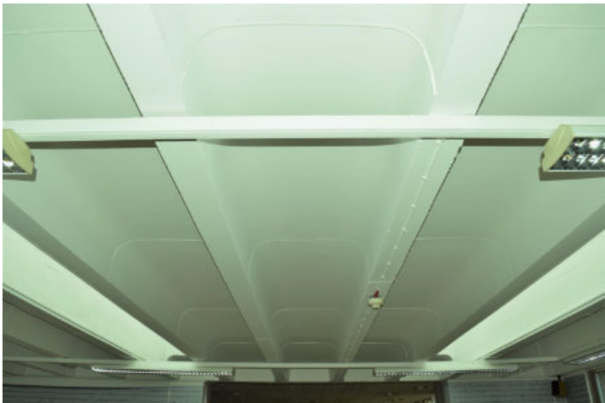
Figure 61 Refectory restaurant, NW section roof beam details, view SE.
