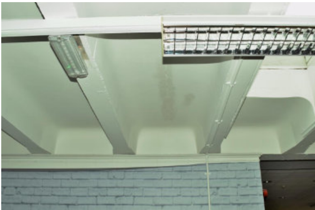
Figure 65 Ceiling beam end details, view SE.
