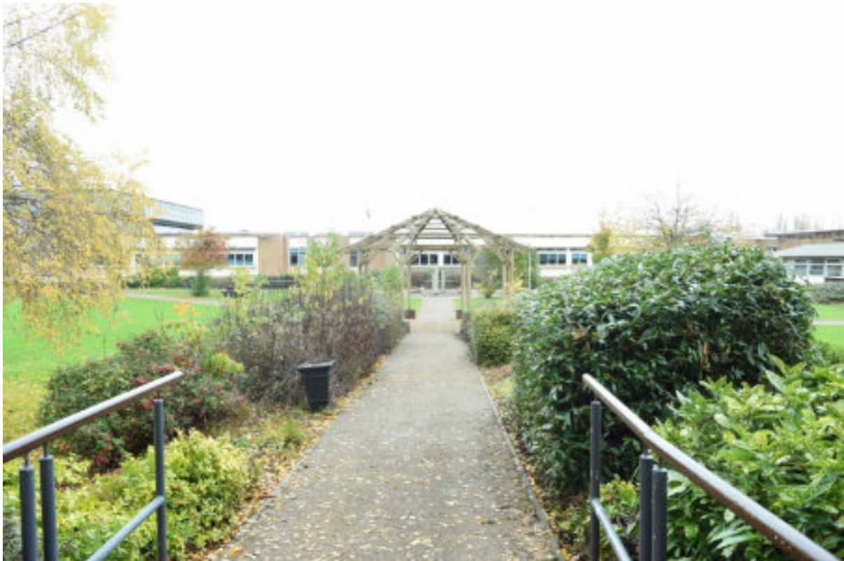
Figure 31 D Block from central doorway in NE elevation of front (SW) range of main building.
