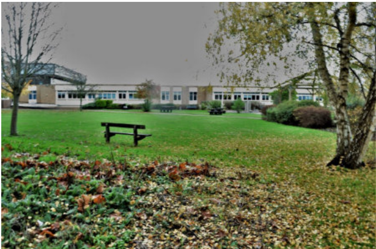
Figure 29 D Block from SW across quadrangle.
