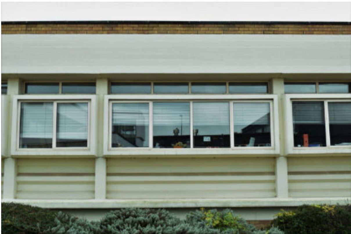
Figure 15 NE elevation D Block window and concrete panel detail.
