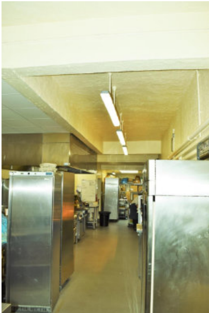
Figure 98 Kitchen, view up kitchen passage, cooking and preparation on L, prep and hatch to servery on R.
