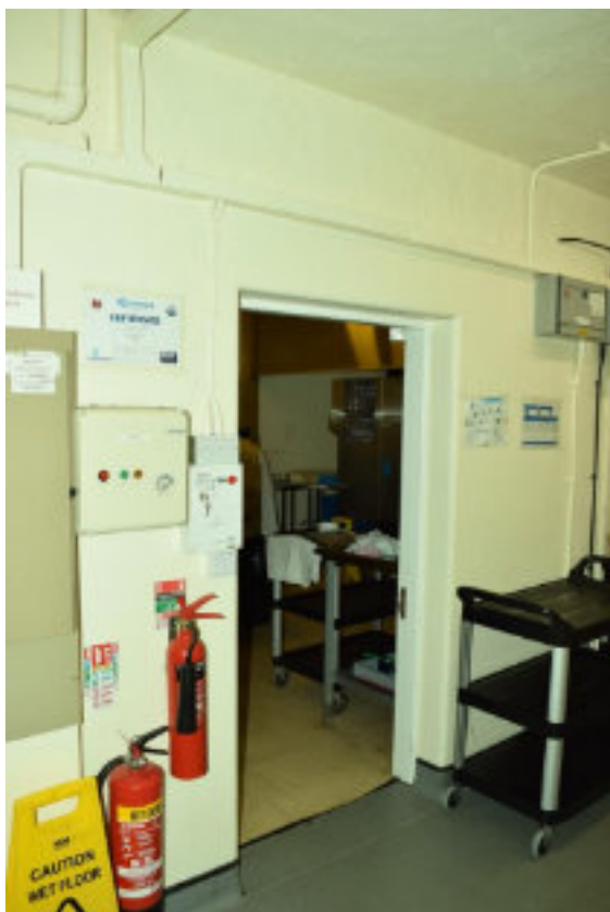
Figure 107 Kitchen SW elevation, door to wash up room.
