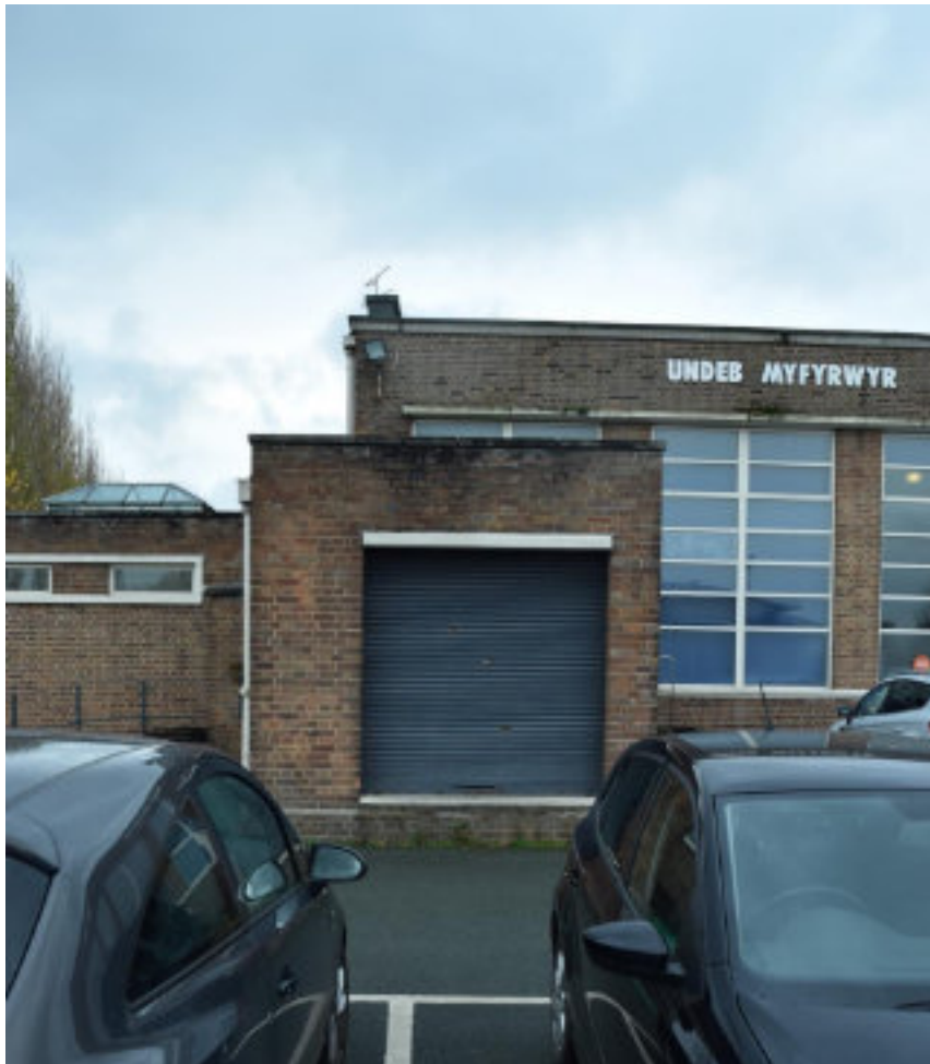
Figure 51 SU NE elevation, southern goods loading bay.
