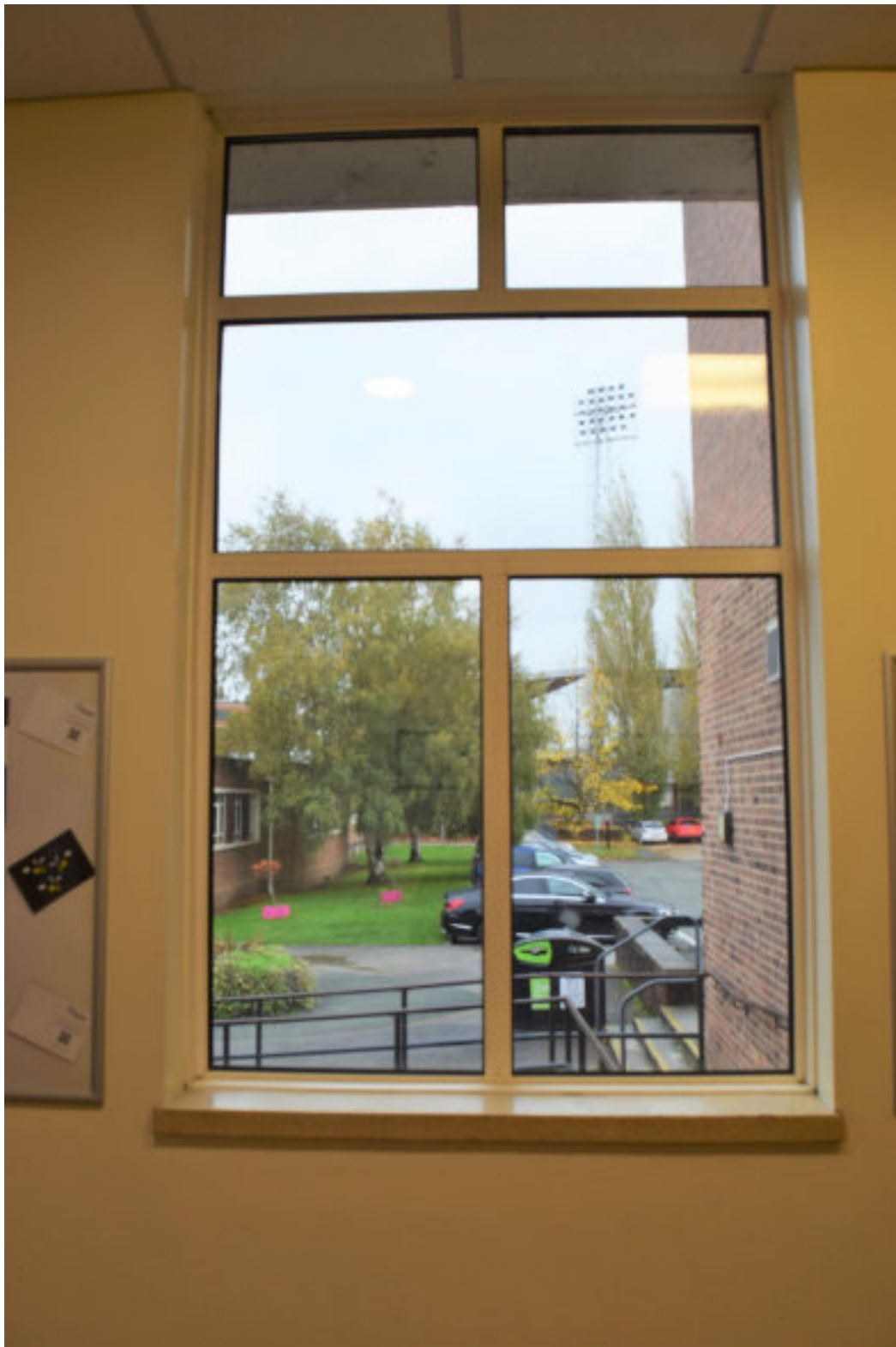
Figure 57 Main corridor, window opposite Refectory main entrance, detail.
