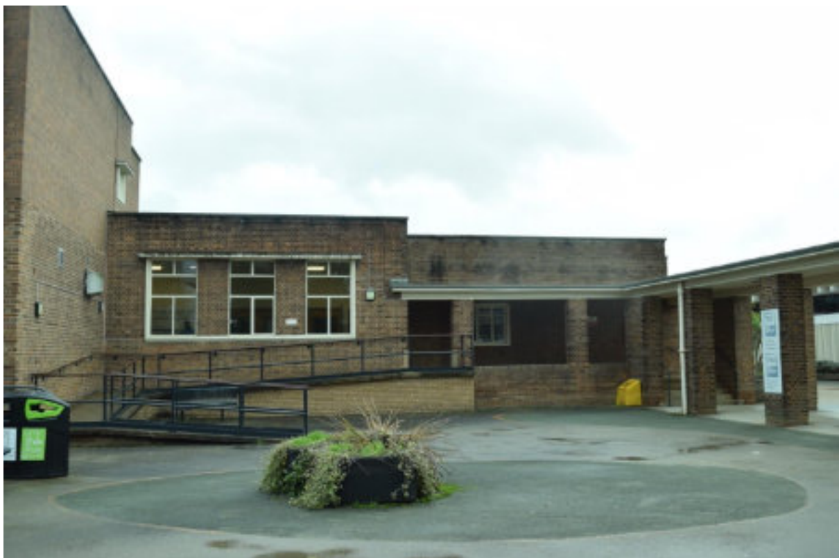
Figure 37 SE elevation of Refectory, covered walkway to Students Union Building on right.
