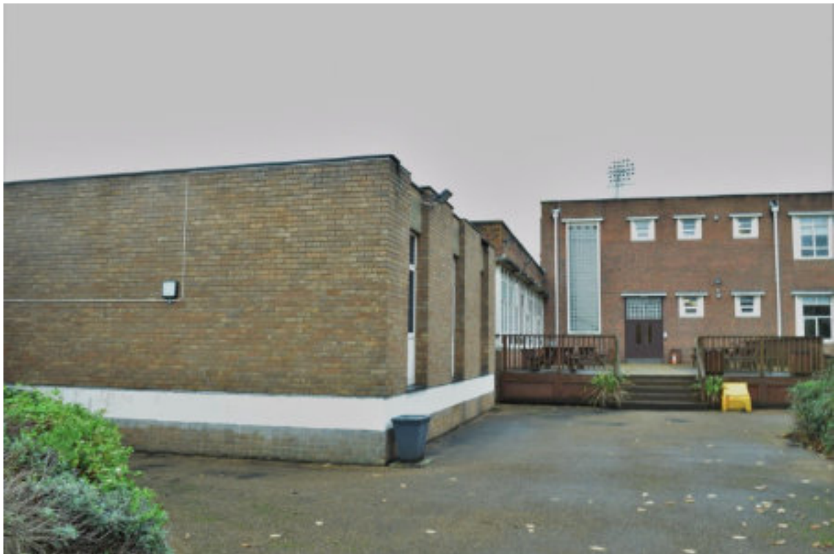
Figure 36 Refectory block and patio from NW, the tall, multipane, stair windows, as shown centre, are a feature of the first phase buildings on the campus.
