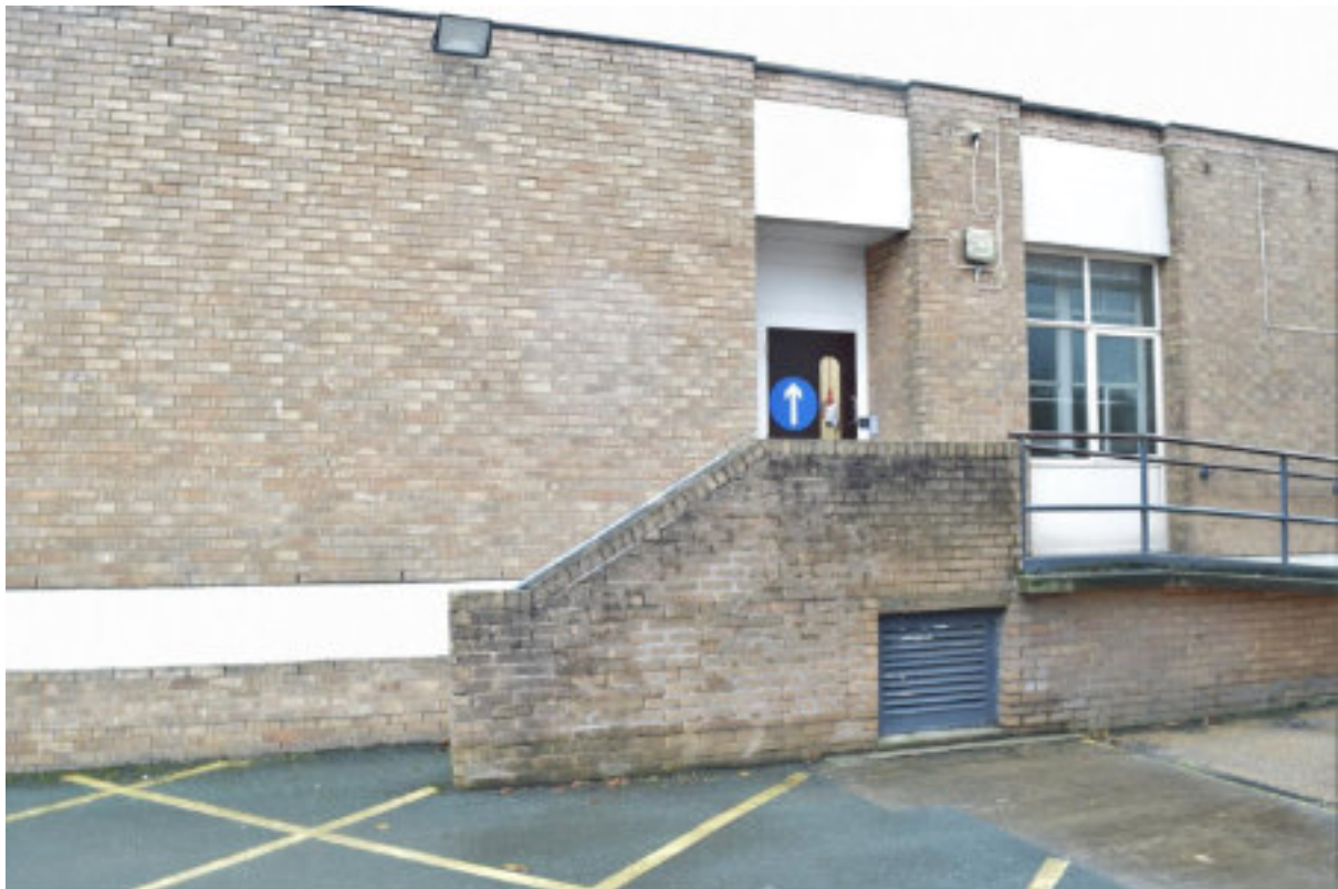
Figure 24 D Block NW elevation steps and ramp to entrance door.
