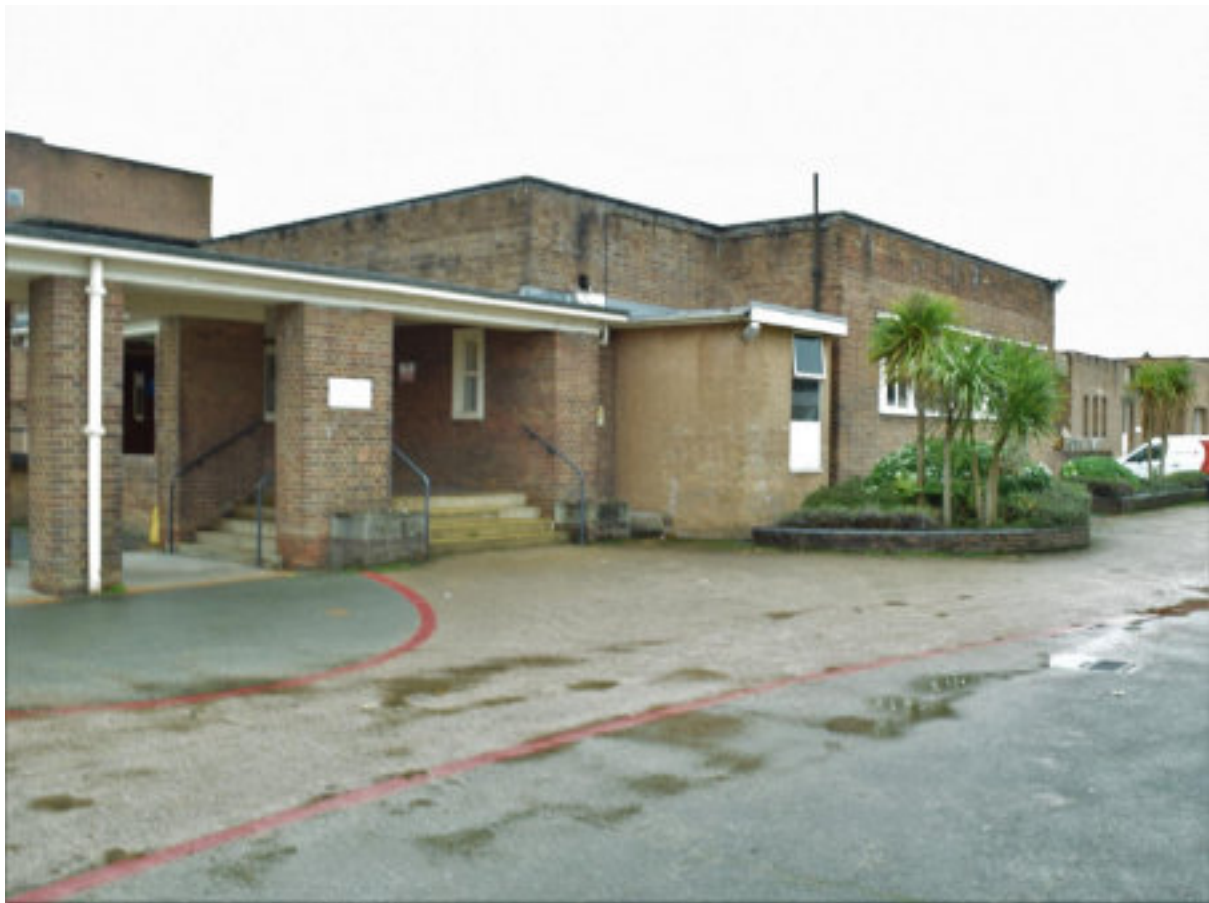
Figure 7 Refectory North-eastern elevation from E.
