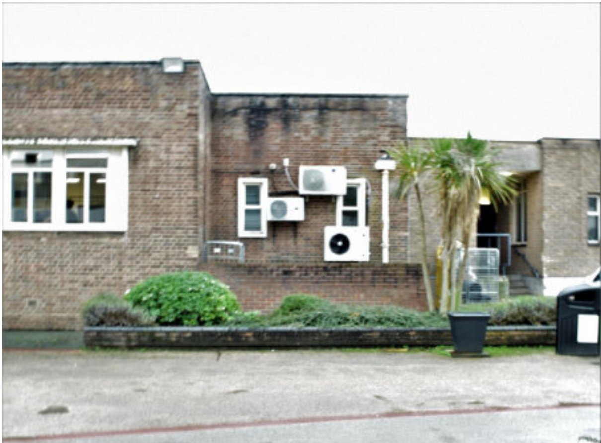
Figure 10 NE elevation Kitchen cold stores.
