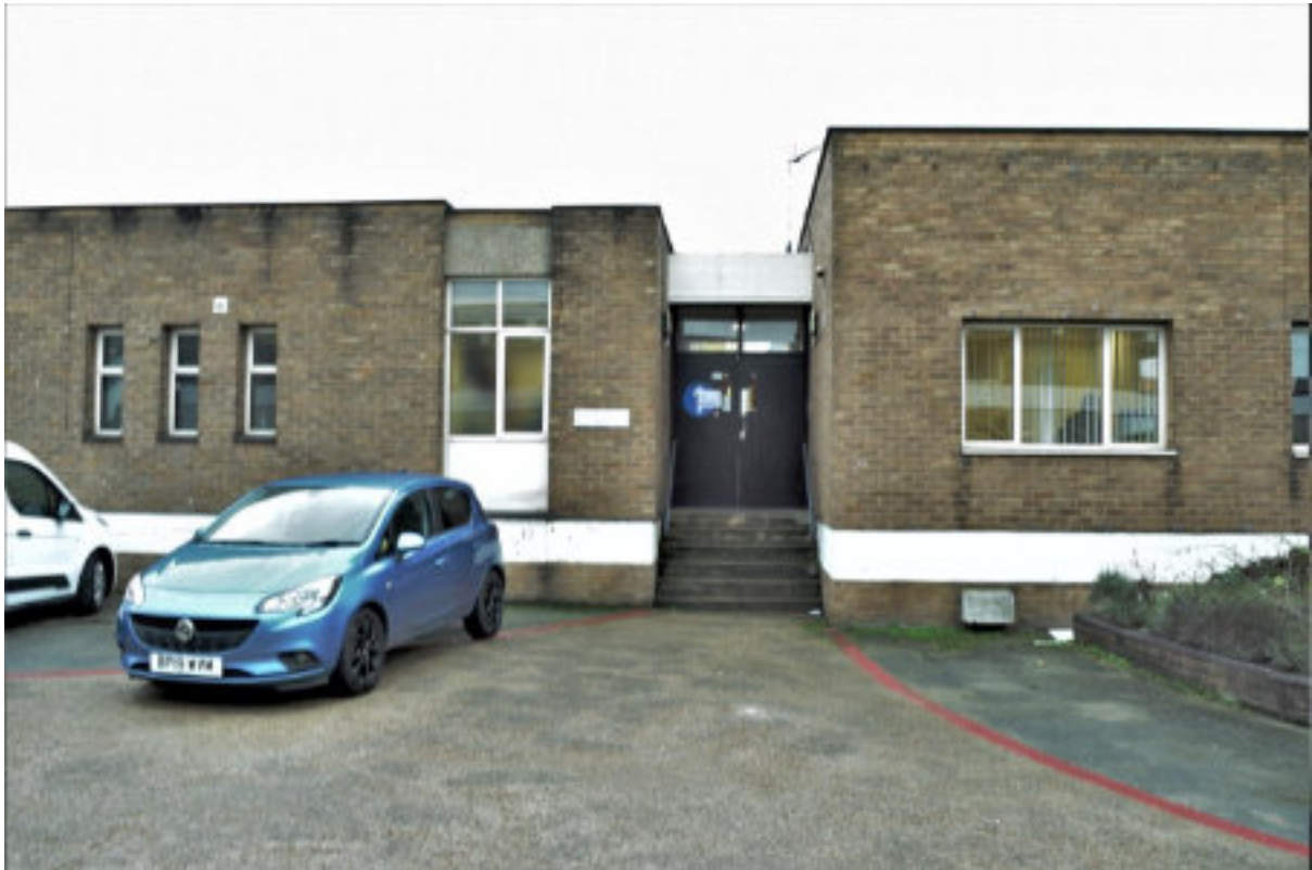
Figure 12 Link entrance between Refectory on L and D Block on R.
