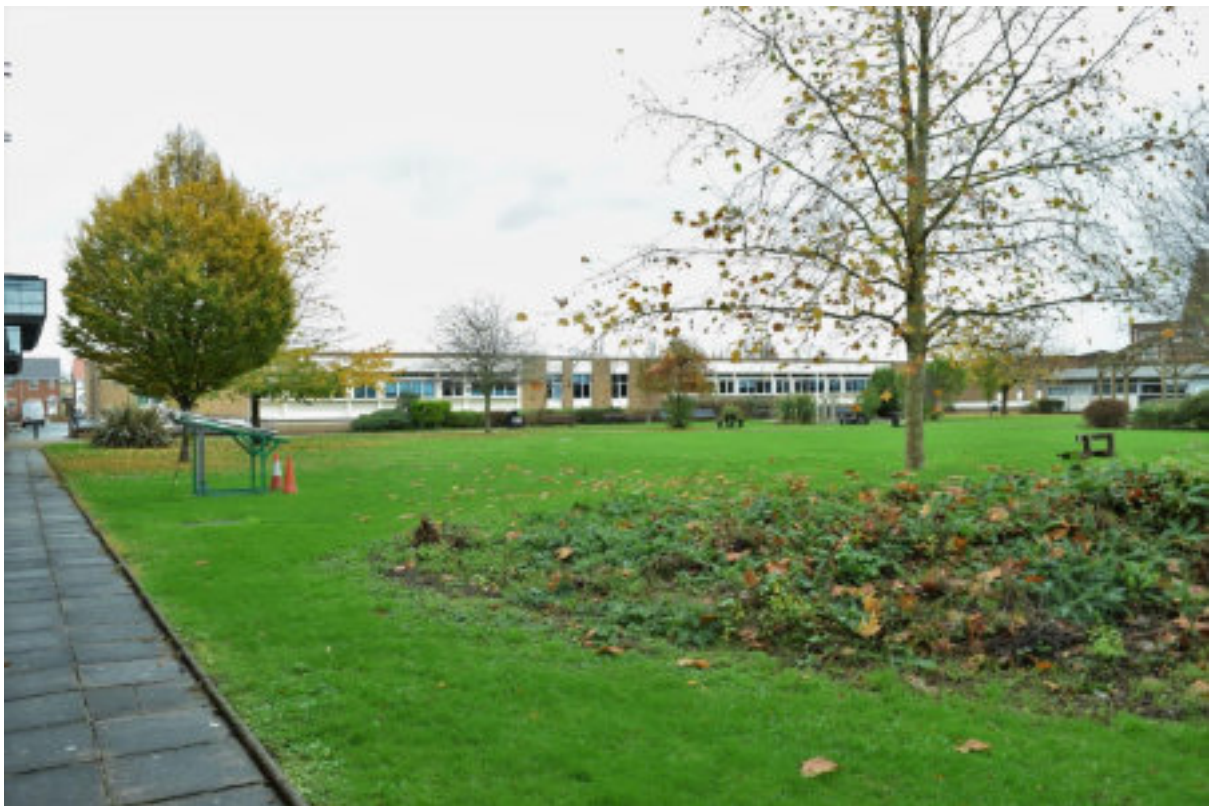
Figure 27 D Block SW elevation from W across quadrangle.
