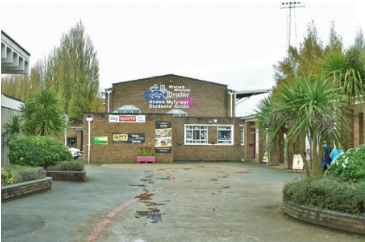
Figure 40 SU NW elevation from NW.
