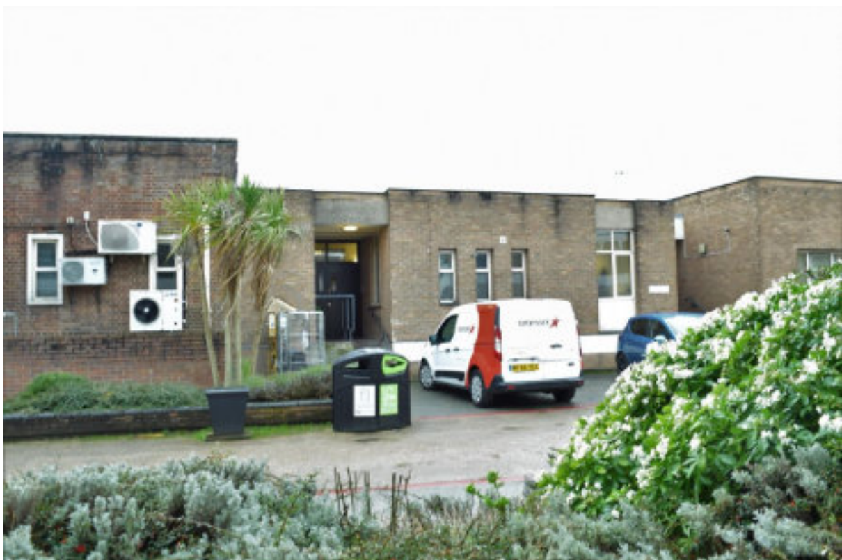
Figure 11 NE elevation Kitchen cold stores and storerooms.
