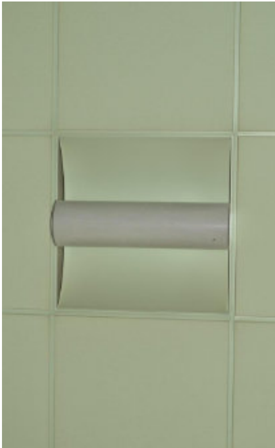
Figure 87 Restaurant SE section light fitting detail.
