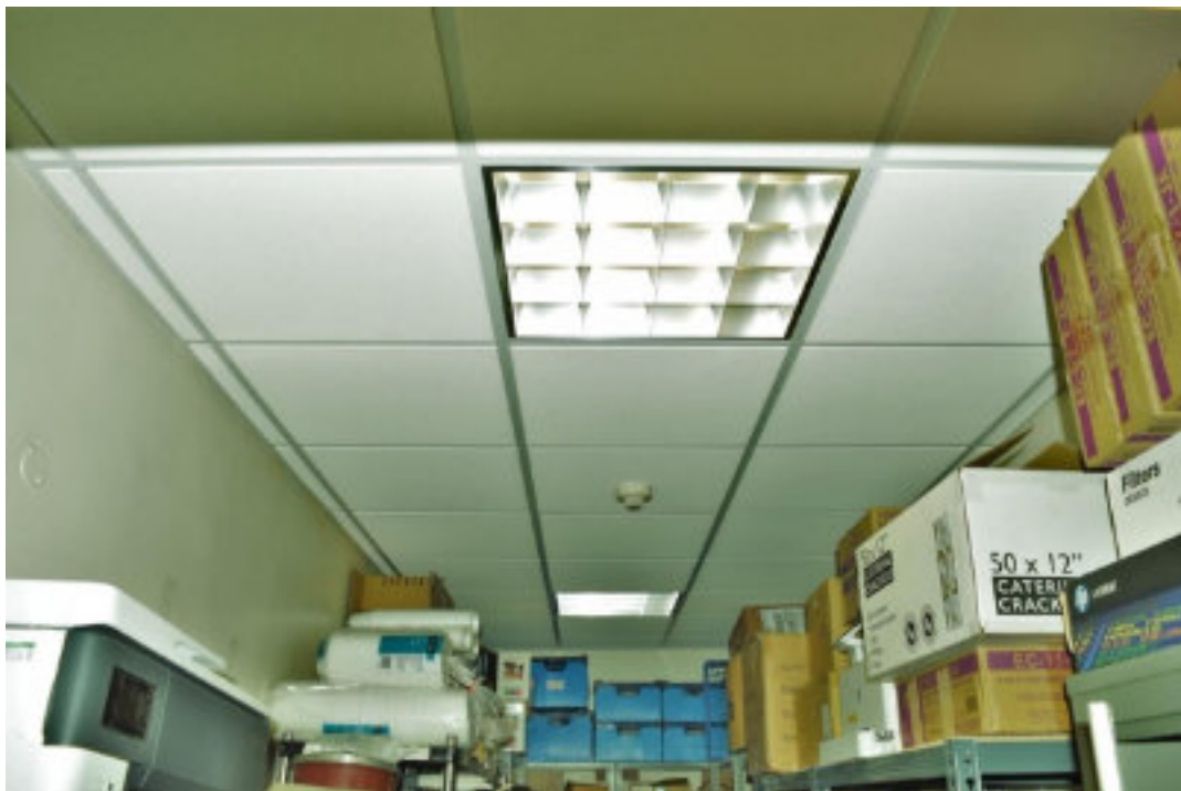
Figure 111 Service Corridor store room, suspended ceiling and light fittings detail.
