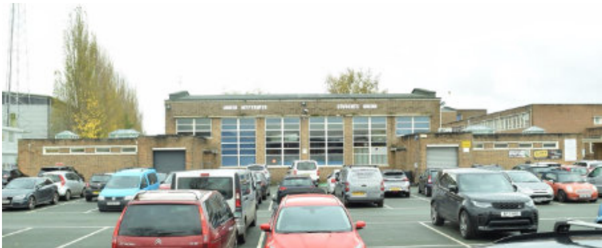
Figure 49 SU NE Elevation view from NE.
