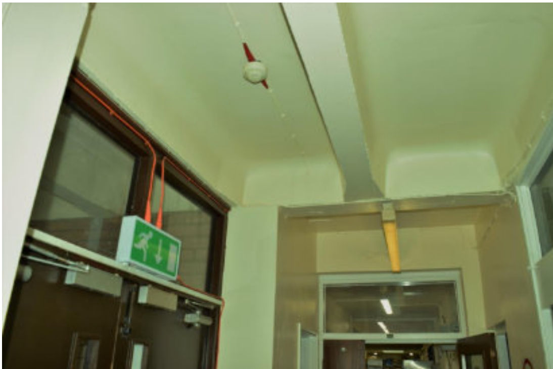
Figure 97 Service corridor NW end ceiling detail view to NW.
