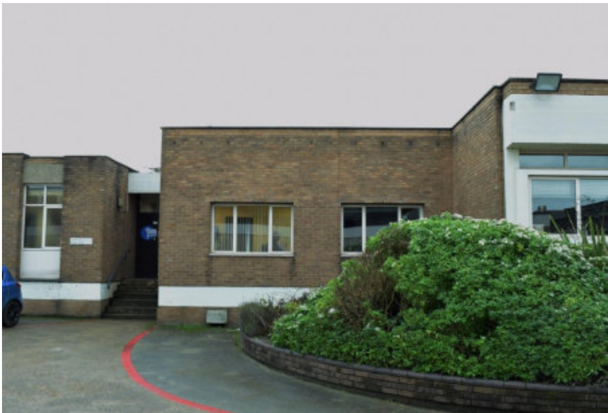
Figure 13 D block NE elevation Rooms D10 and D 12.
