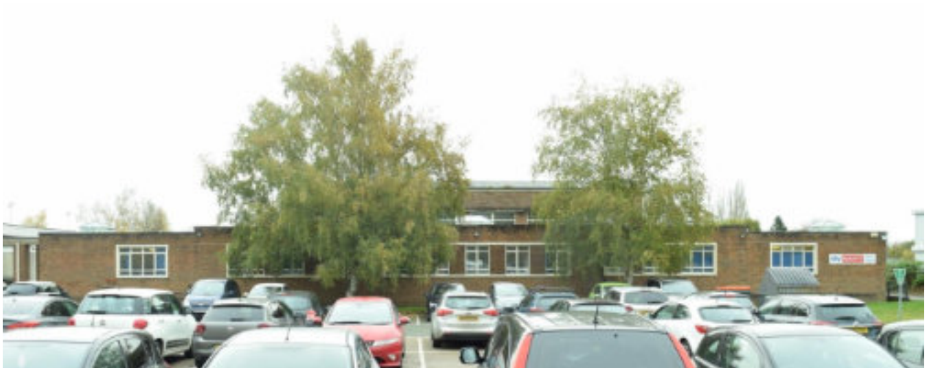
Figure 42 SU SW elevation from SW.
