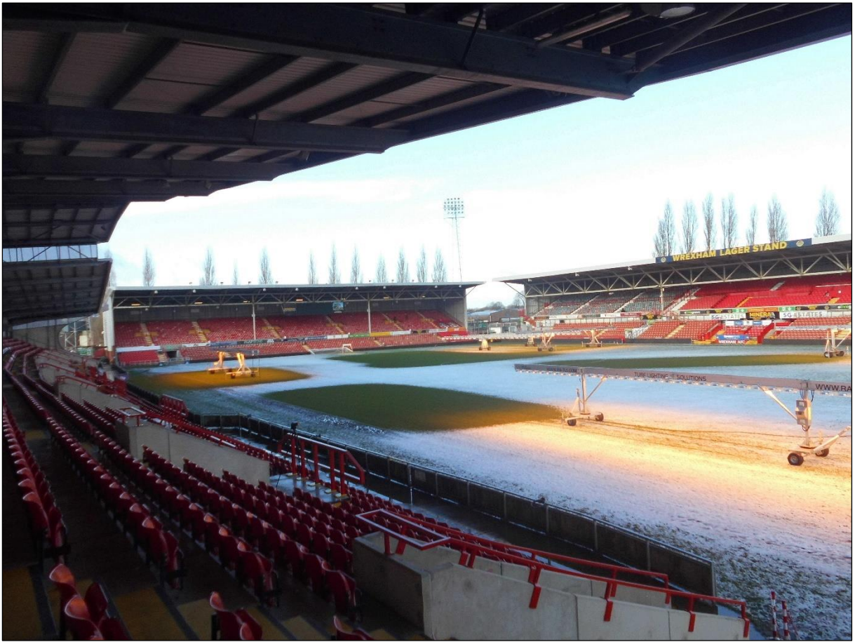
Plate 21: Floodlight A from stands, looking N
