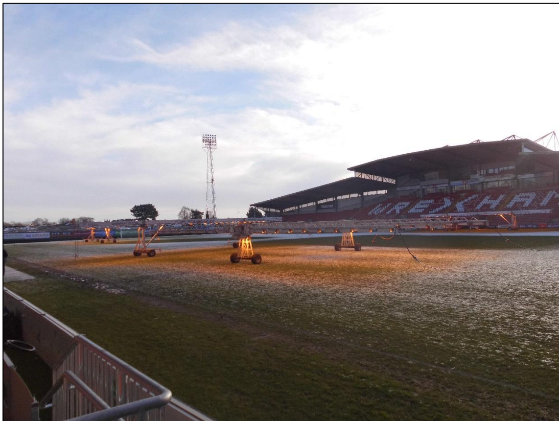
Plate 24: Floodlight C from stands, looking S.
