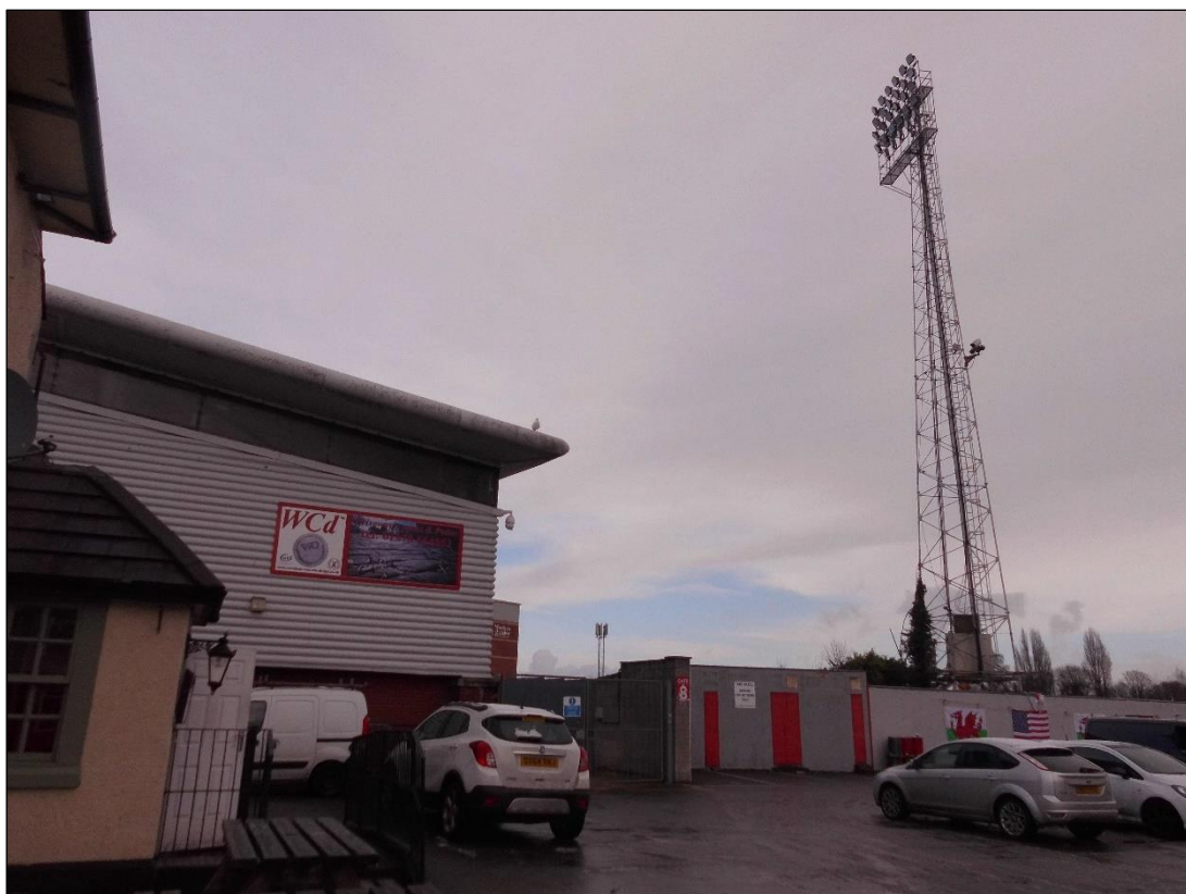
Plate 6: Floodlight C from The Turf pub car park, looking E.
