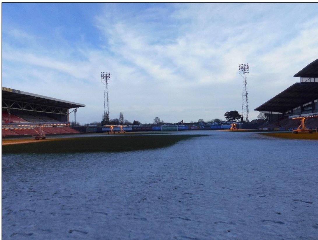
Plate 17: Floodlights C and D within stadium, looking SE.
