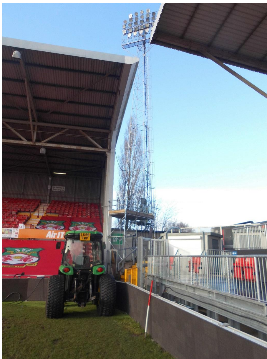
Plate 22: Floodlight A from within stadium, looking N. 1m scale.
