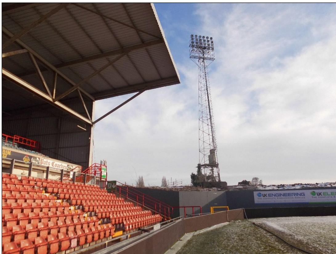
Plate 12: Floodlight D from within stadium by stands, looking SE.
