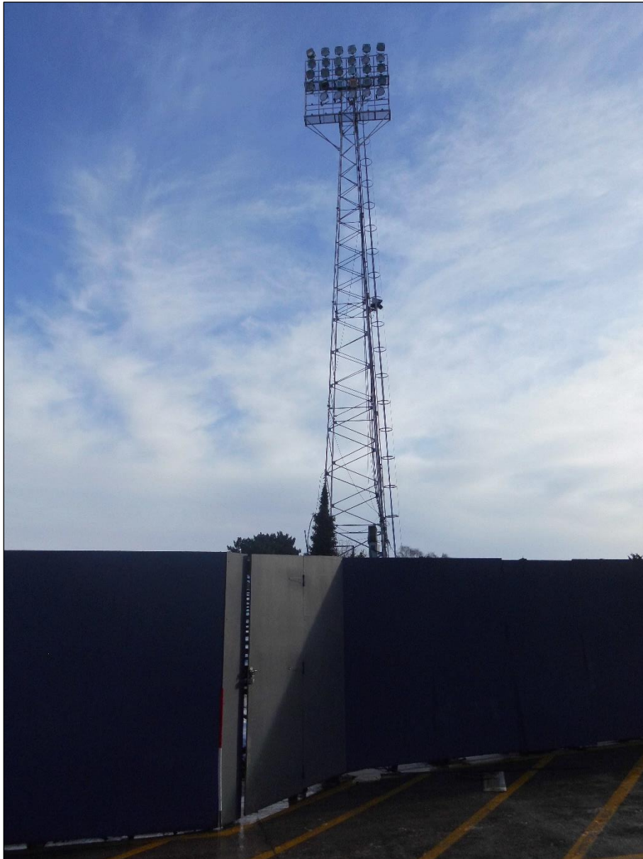
Plate 15: Floodlight C from within stadium, looking S. 1m scale.
