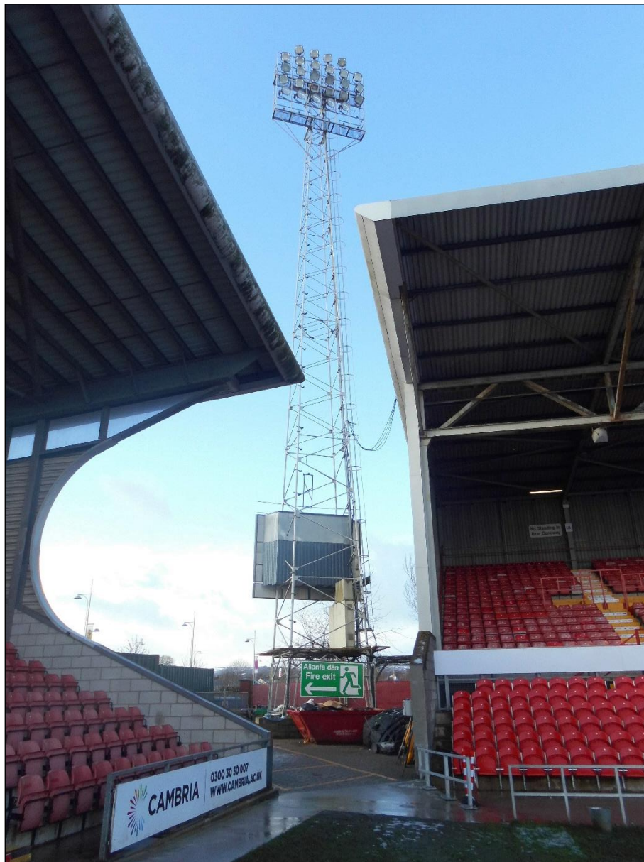
Plate 19: Floodlight B from within stadium, looking W
