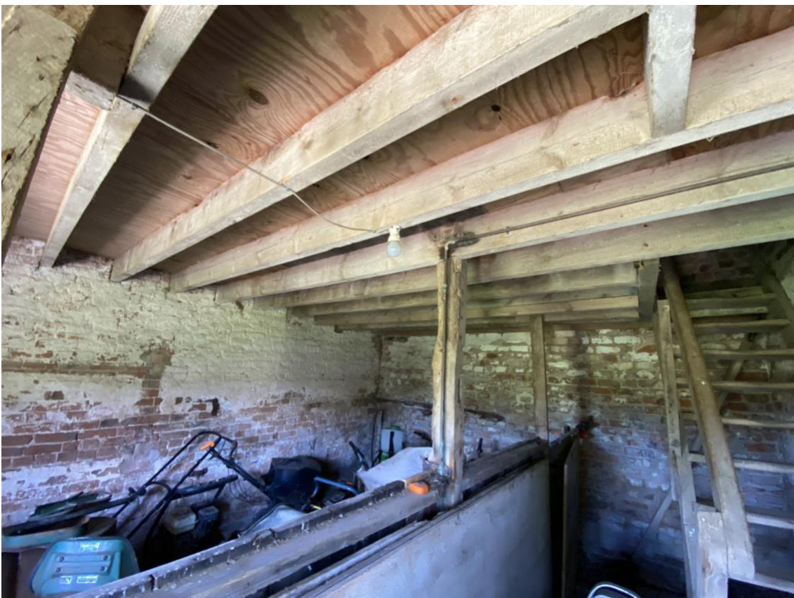
The ground floor of the building. No evidence of bats found within the ground floor
