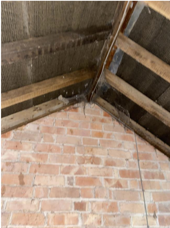
The roof liner is present beneath the roof slates within the building
