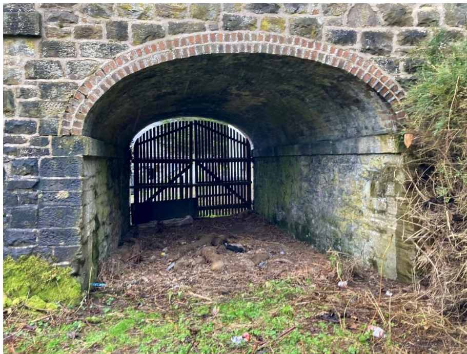
Figure 4: Bridge 31 on the east side of Trevor Basin
