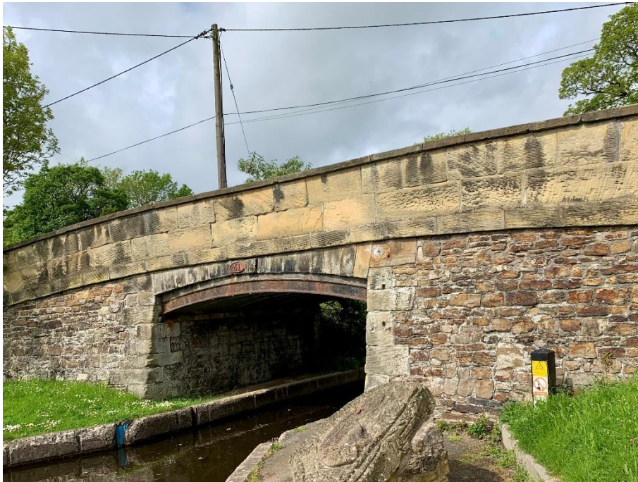
Figure 3: Bridge 31 on the east side of Trevor Basin.
