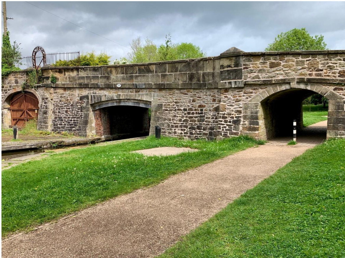
Figure 2: The view of the south elevation of Scotch Hall bridge.
