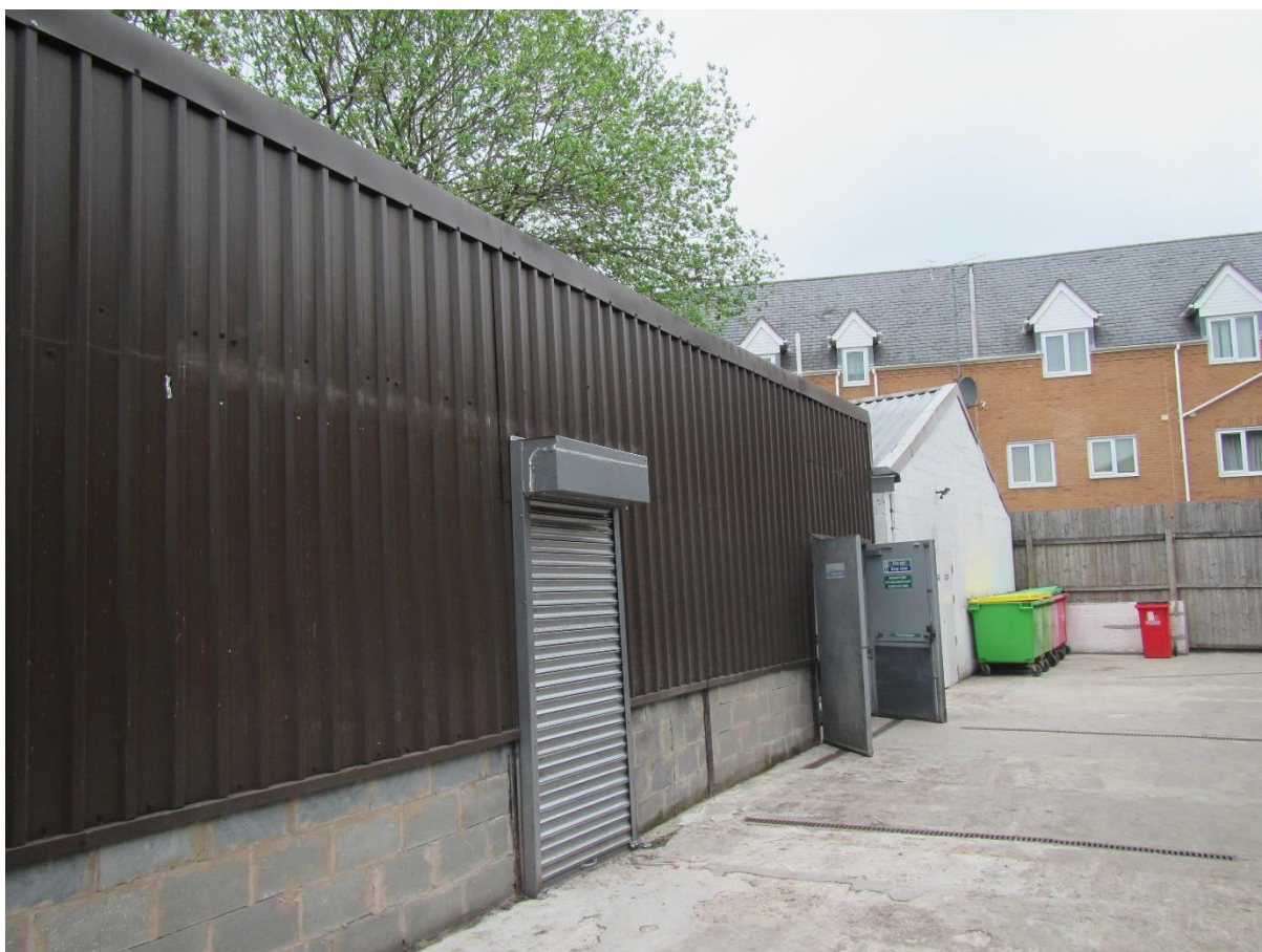
Photograph 1 – South-eastern aspect of the bakery and warehouse.
