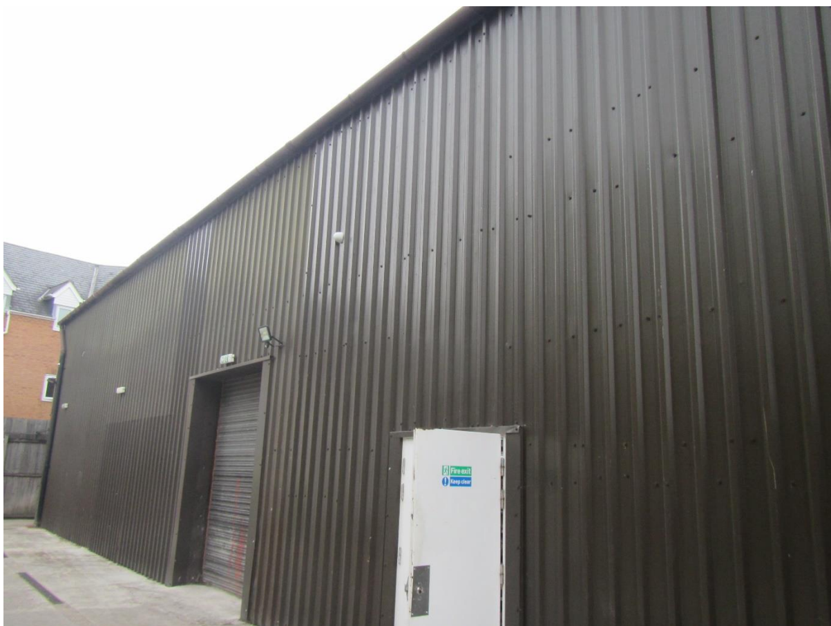
Photograph 13 – North-western aspect of the supermarket 'Chata Polska'.
