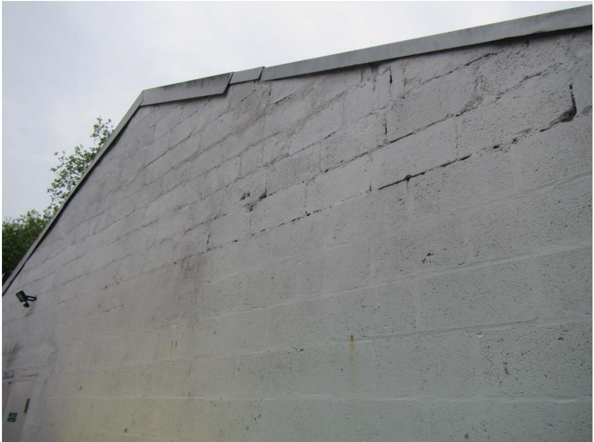
Photograph 3 – Lifted metal facias.
