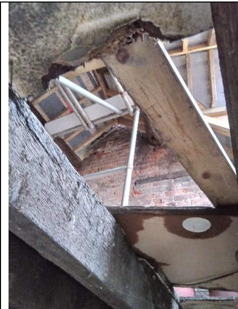
B1 – (interior loft space 3)
