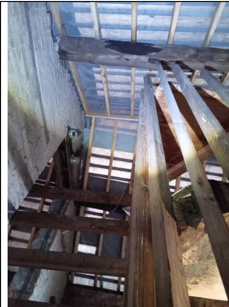
B1 – (interior loft space 2)
