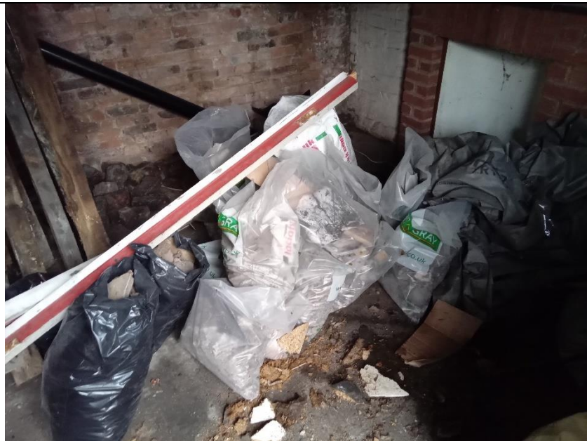
B1 – (interior loft space 3) (debris storage)
