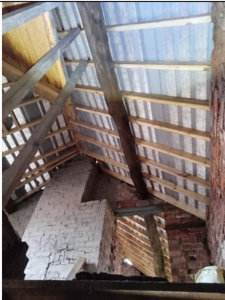
B1 – (interior loft space 2)
