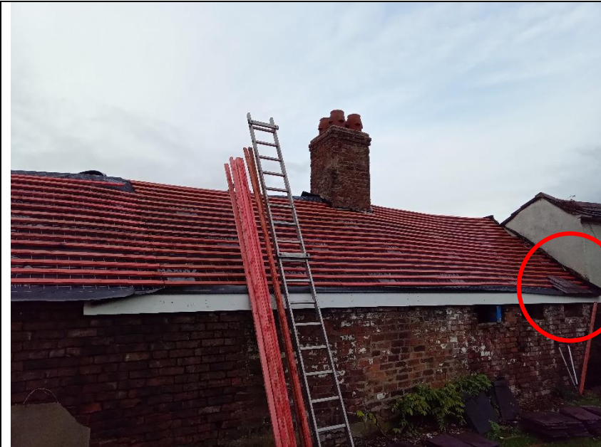
B1 – (western elevation) (few newly placed tiles)
