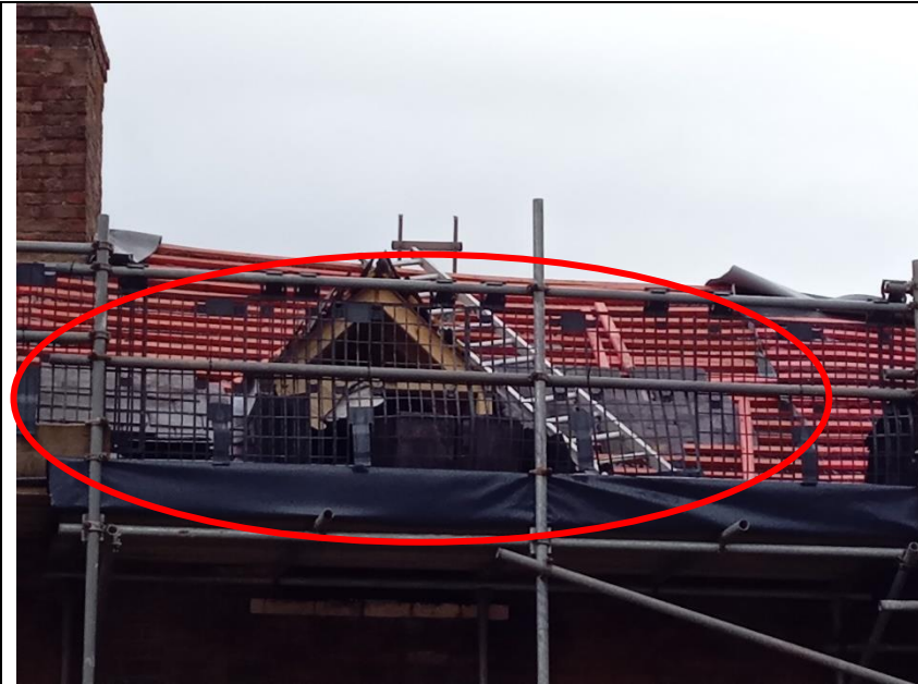
B1 – (eastern elevation) (few newly placed tiles)
