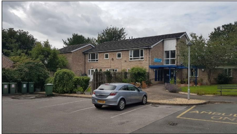
4. The existing building viewed from the car park
