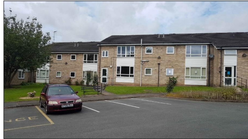
5. The existing building viewed from the car park
