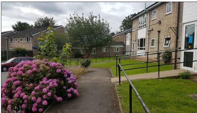
6. The existing building viewed from the car park
