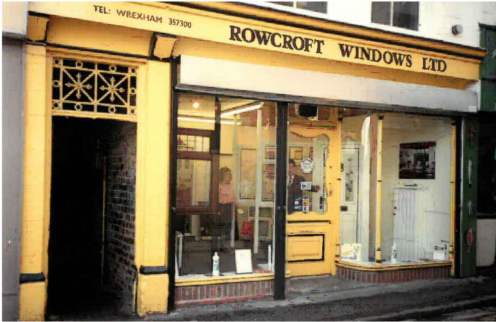
Historical Photograph 4 Henblas Street
