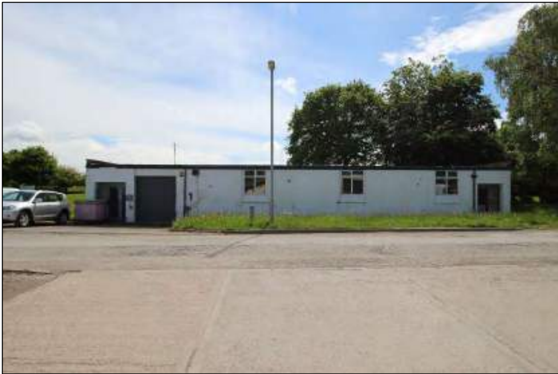
Plate 51: Front, north-west elevation of Building 6, looking south-east across access road
