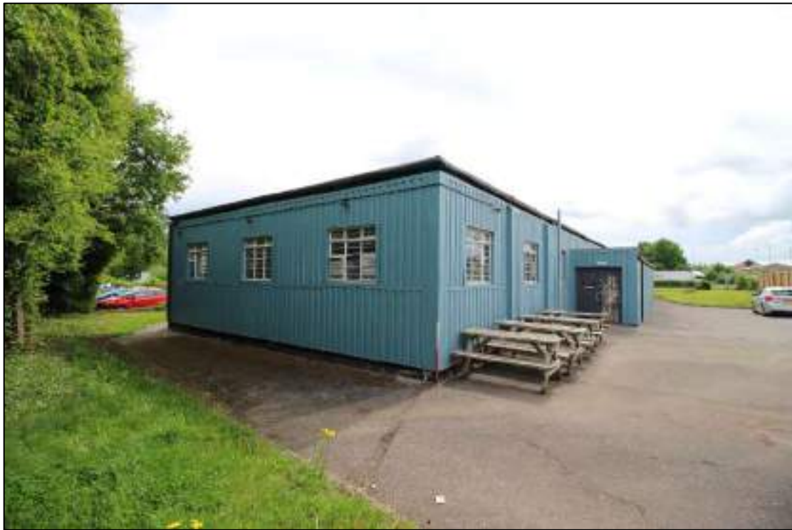
Plate 33: North-west end elevation of Building 3, looking east
