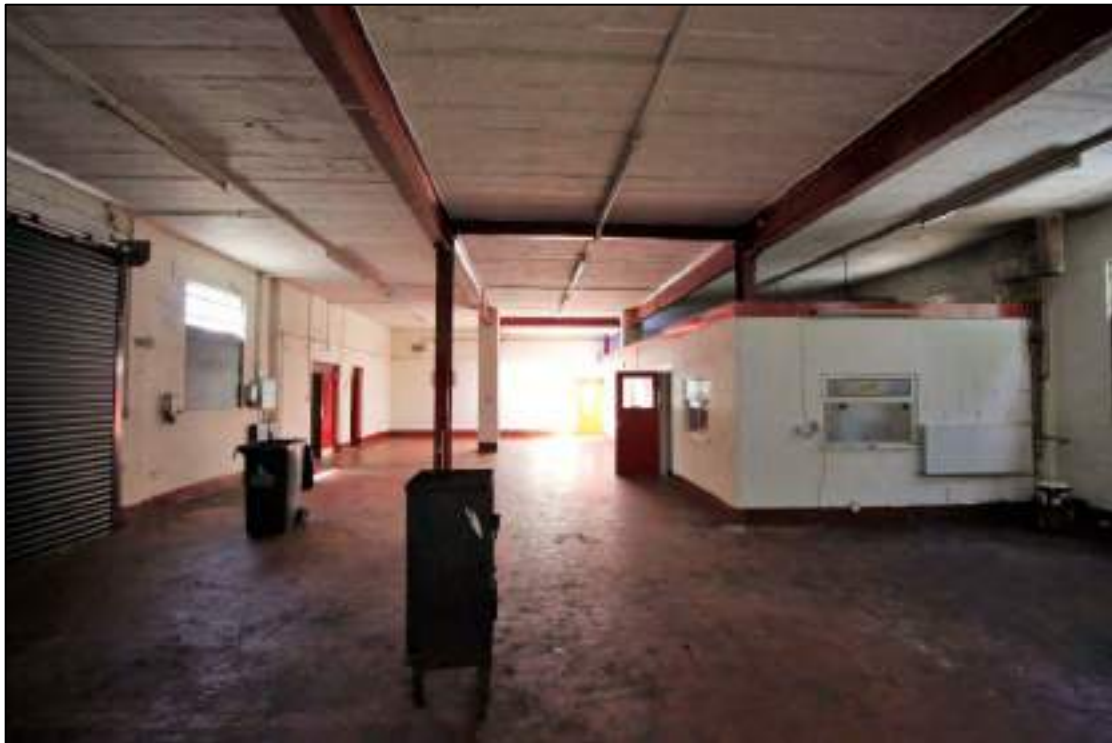
Plate 71: South-east half of Building 8, looking north-west toward cinder block partition wall
