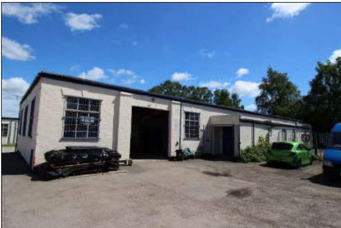
Plate 69: Vehicle entrance at north-west end of south-west elevation, looking east
