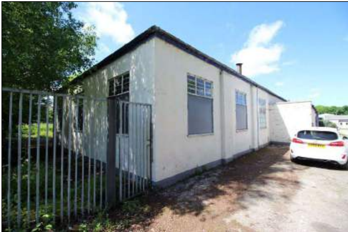
Plate 66: South-east elevation and south-east end of north-east elevation, looking west
