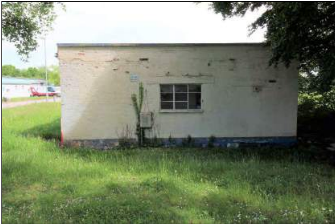
Plate 52: Remodelled openings with south-west elevation of Building 6
