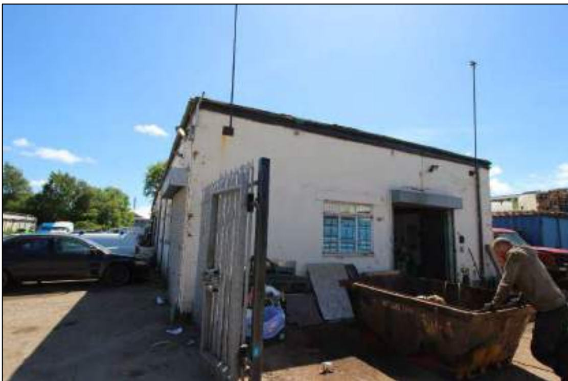
Plate 80: North-west elevation of Building 9, looking south-east
