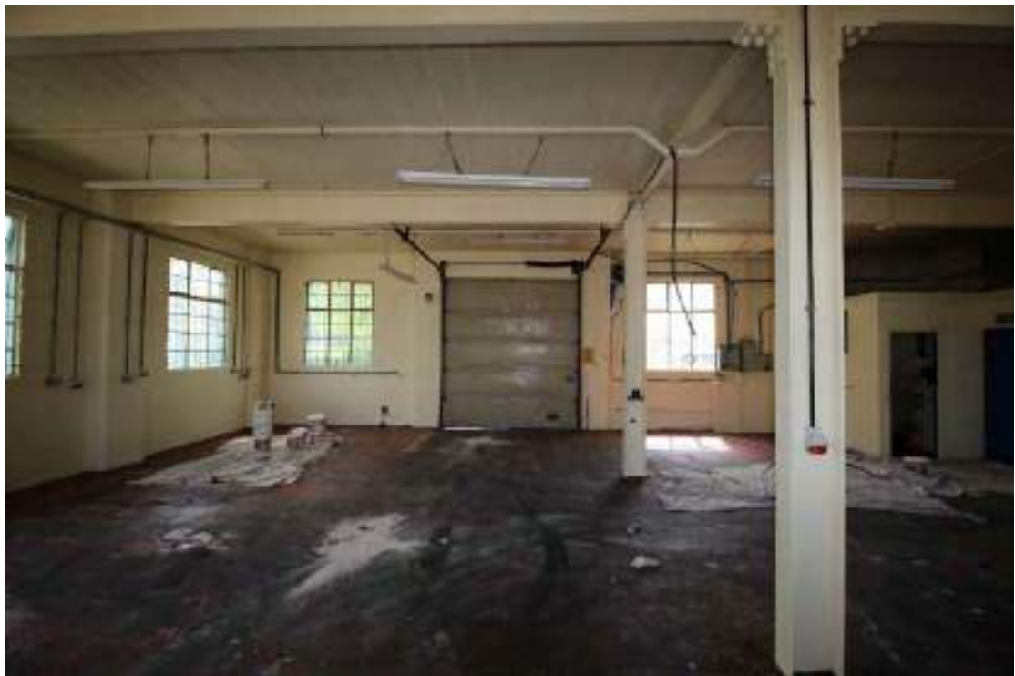
Plate 45: Detail of junctions between ceiling beams and columns, in north-east end of Building 5, looking south-east
