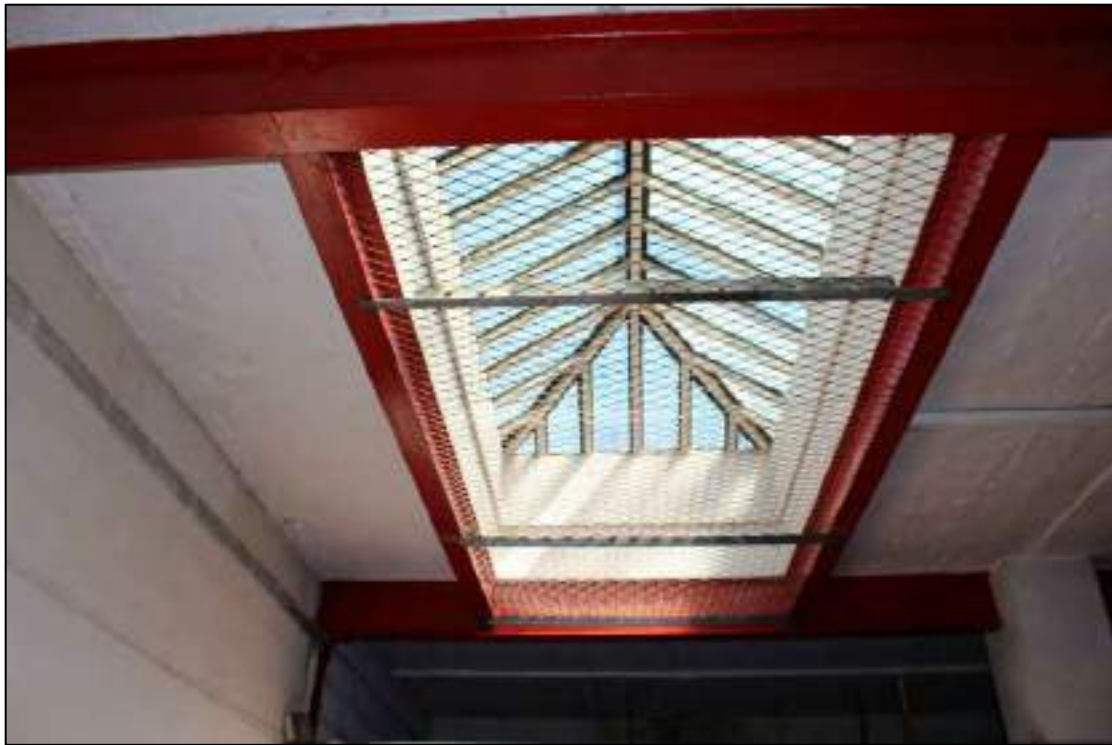
Plate 73: Detail of ridged skylight and surrounding beams, adjacent to centre wall
