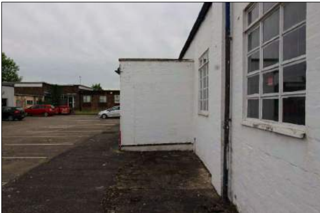
Plate 21: Infilled entrance at north-west end of lean-to on north-east side of Building 2, looking south-east
