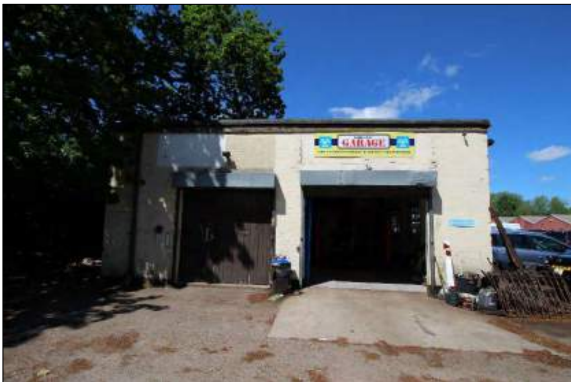
Plate 77: Vehicle entrances in south-east elevation of Building 9
