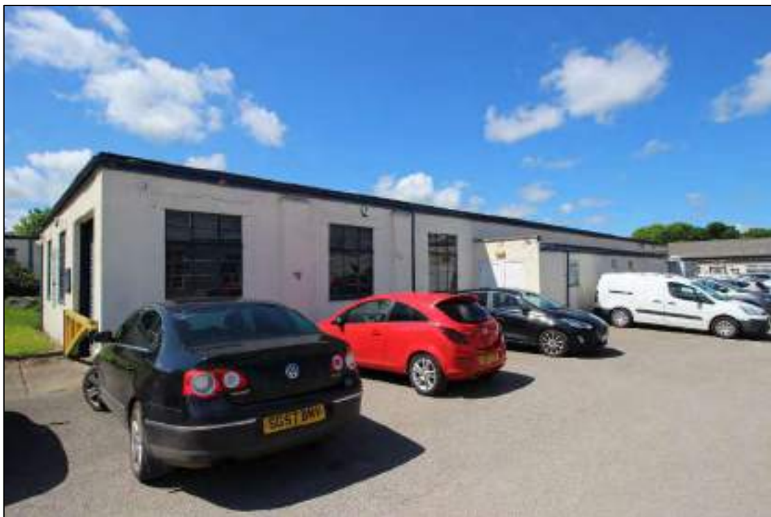
Plate 62: Rear north-east elevation of Building 7, looking west
