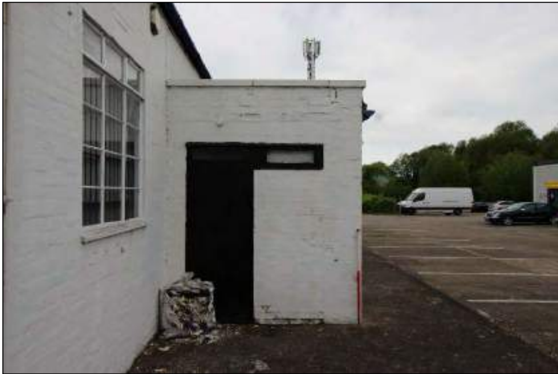
Plate 20: Remodelled entrance at south-east end of lean-to on north-east side of Building 2, looking north-west
