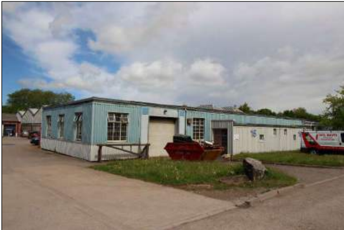
Plate 42: Oblique view of front, south-east elevation of Building 5, looking north
