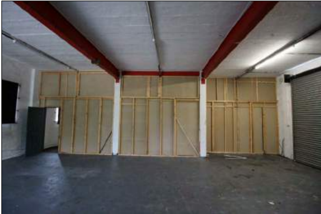
Plate 27: Interior of Building 2, spanned by steel I beams, looking south-east
