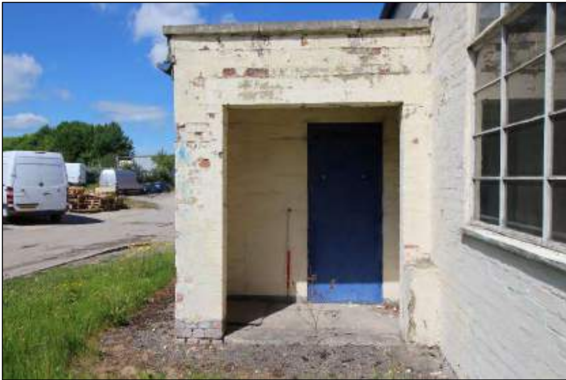
Plate 63: Remodelled doorway within porch at north-west end of rear, north-east lean-to
