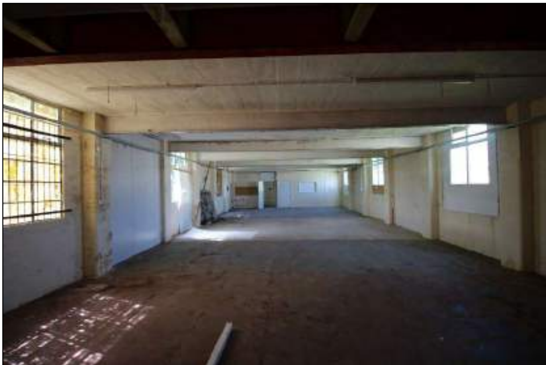
Plate 55: Interior of Building 6, looking south-west toward modern partition wall
