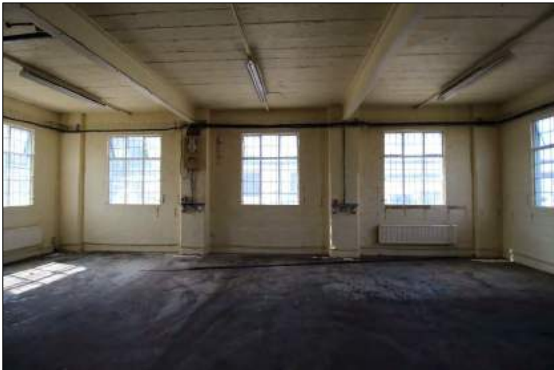
Plate 47: Windows within south-west end of Building 5, looking south-west
