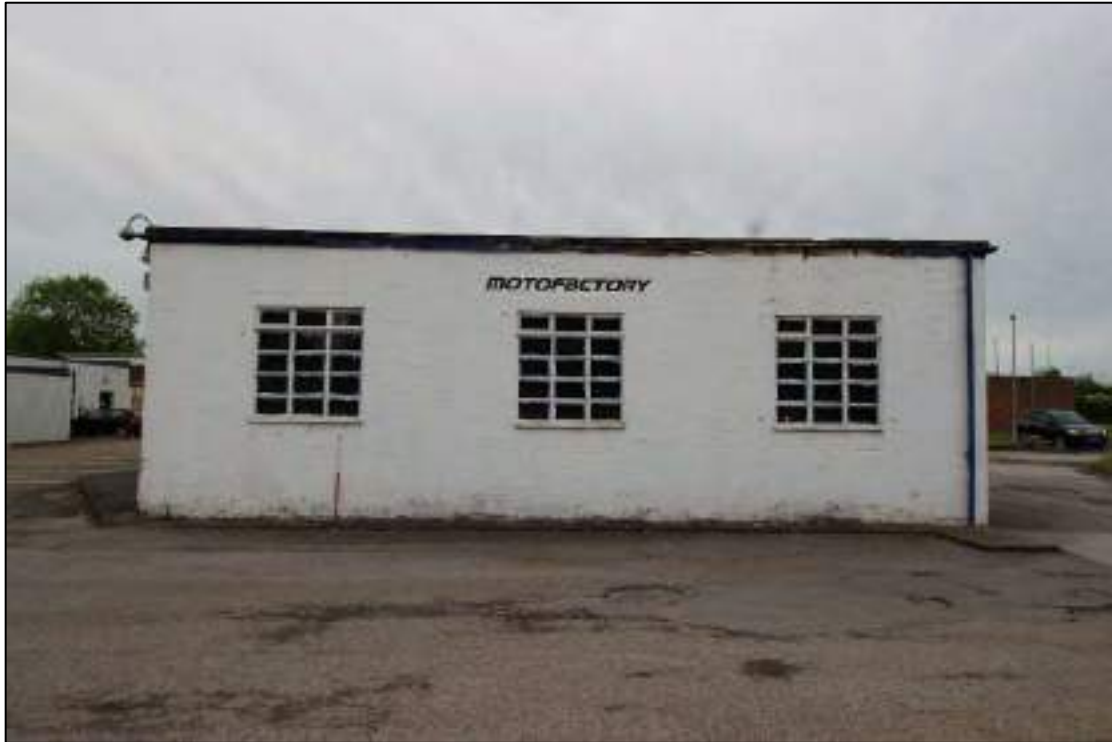
Plate 22: North-west elevation of Building 2, looking south-east
