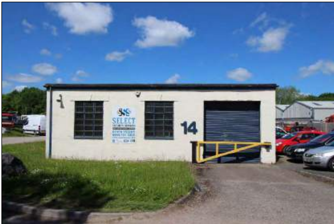
Plate 61: South-east elevation of Building 7, looking north-west
