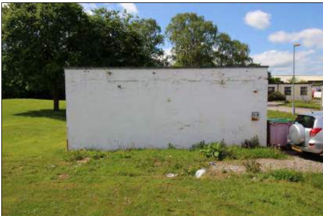
Plate 54: North-east elevation of Building 6
