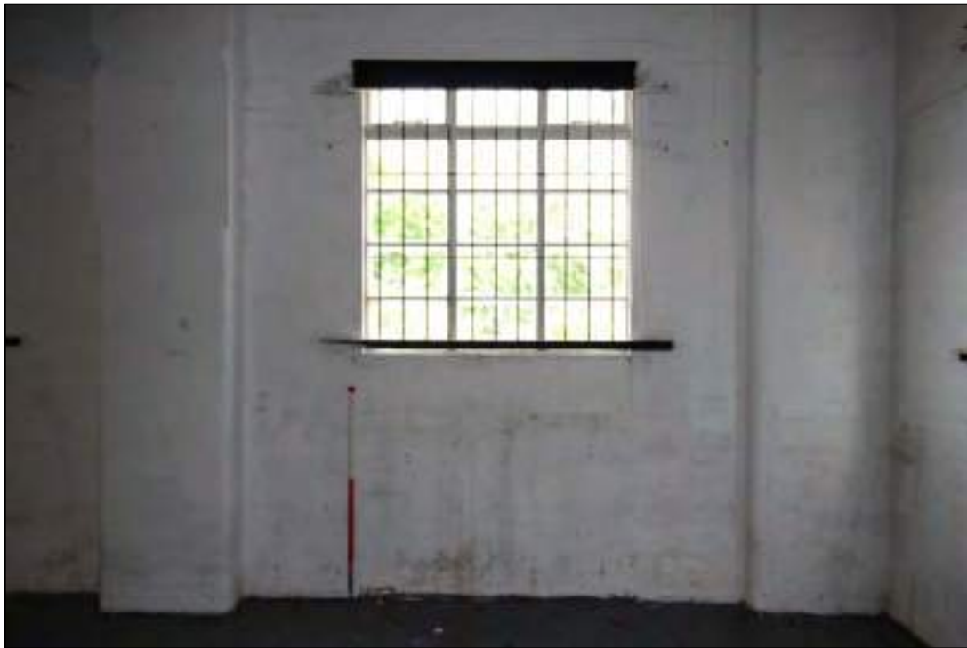
Plate 30: Detail of interior of window opening, within north-west wall of Building 2, looking north-west
