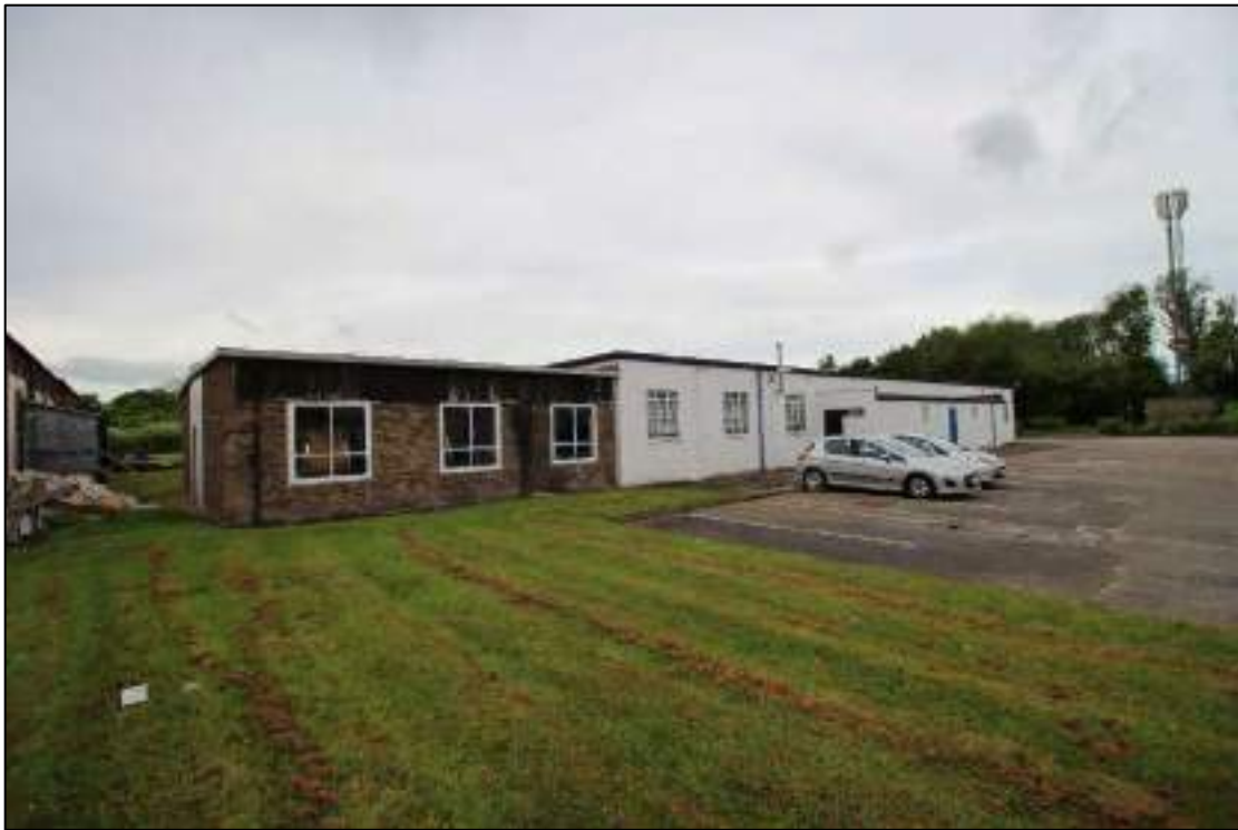
Plate 18: North-east elevation of Building 2 butted by modern extension, looking west
