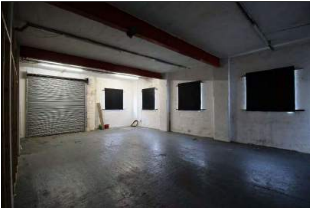
Plate 29: Window openings with the north-west, end wall and vehicle entrance within the south-west wall of Building 2, looking west
