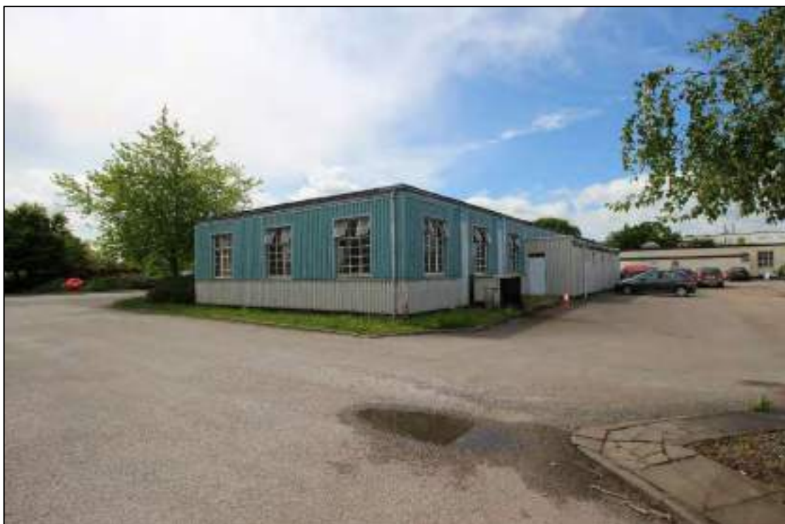
Plate: 43: North-east end elevation of Building 5, looking south
