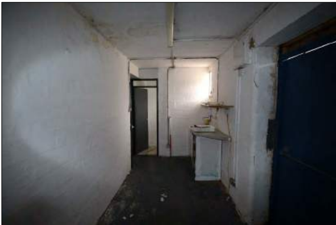
Plate 31: Interior of rear, north-east lean-to, looking north-west
