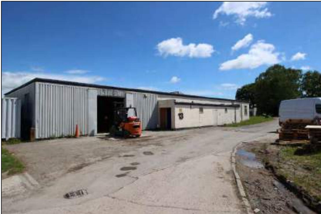
Plate 59: Oblique view of front, south-west elevation of Building 7, looking east
