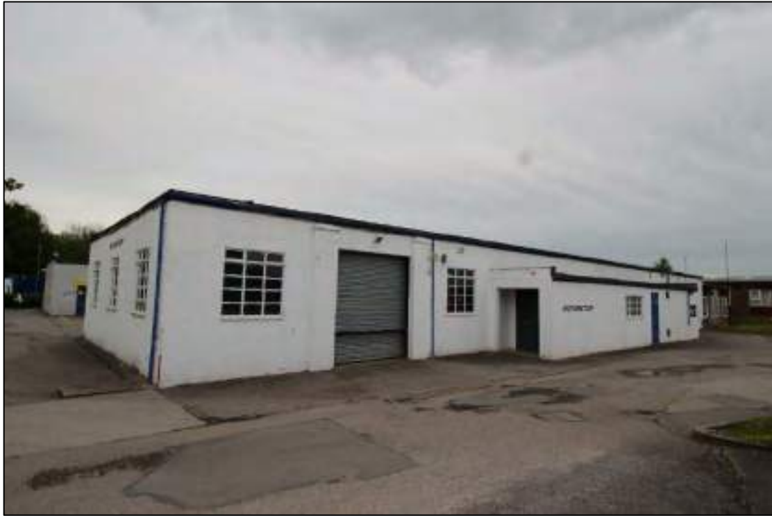
Plate 17: Principal south-west elevation of Building 2, looking east
