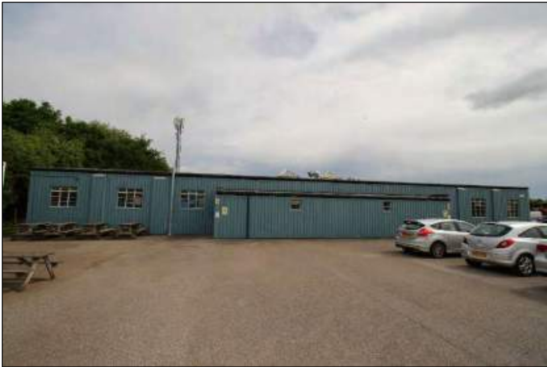
Plate 35: Rear south-west elevation of Building 3, looking north-east
