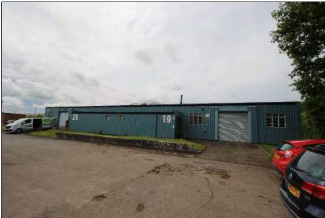
Plate 32: North-east elevation of Building 3, looking south-west
