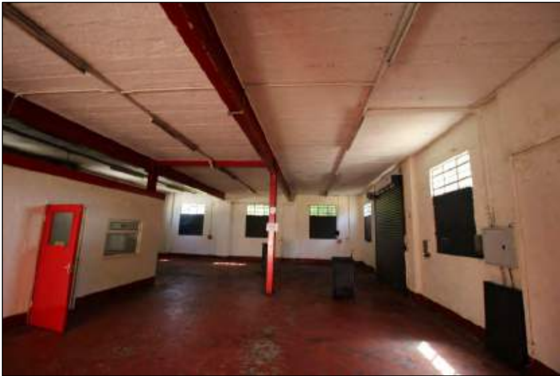
Plate 74: Interior of south-east half of Building 8, looking south-east
