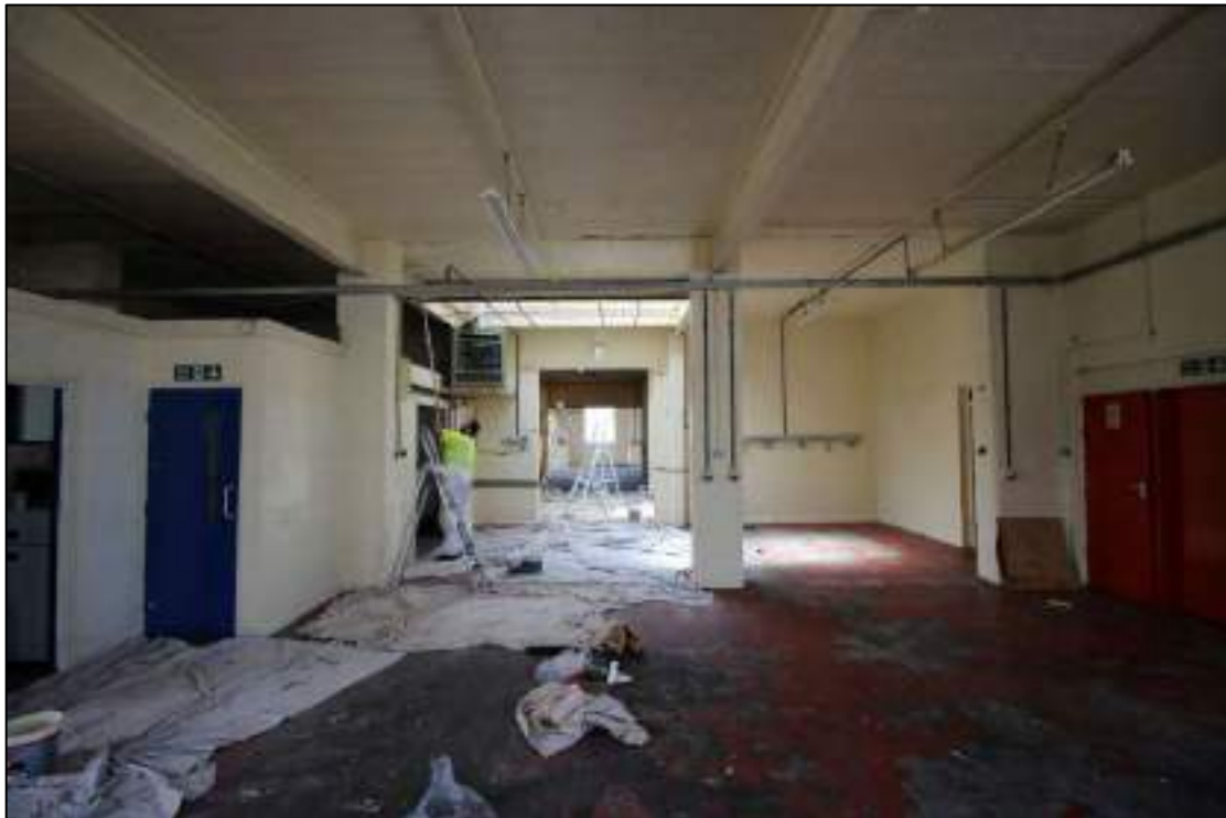
Plate 44: Interior of Building 5, looking north-east towards the centre wall
