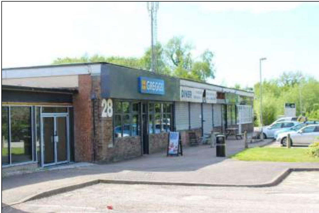
Plate 11: North-east elevation of Building 1, looking west.
