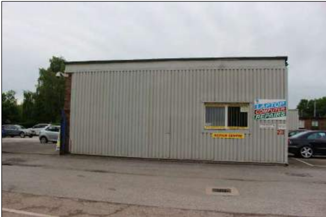
Plate 12: North-west end elevation of Building 1, looking south-east
