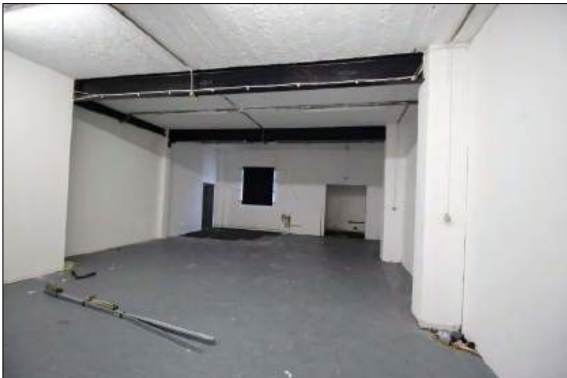
Plate 26: Central subdivision of north-west of Building 2, looking north-east
