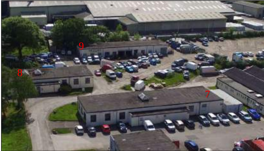
Plate 75: Recent UAV photograph of Building 9 (indicated) at south-west boundary of Site, looking south-west
