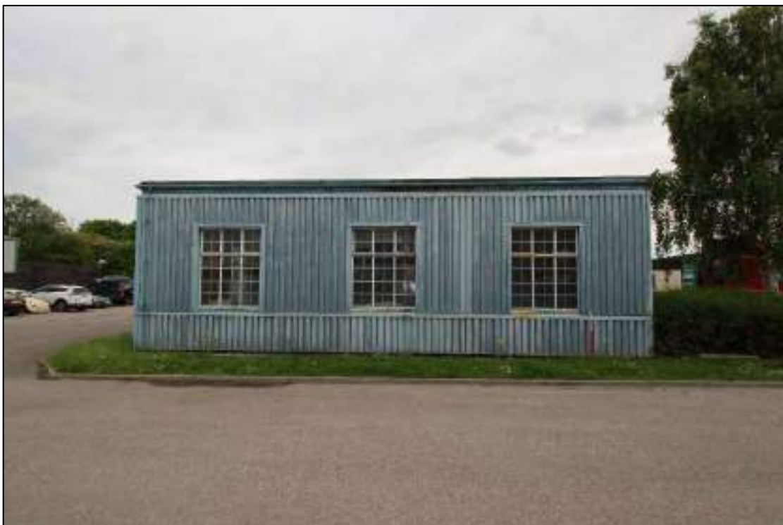
Plate 40: South-west elevation of Building 4, looking north-east
