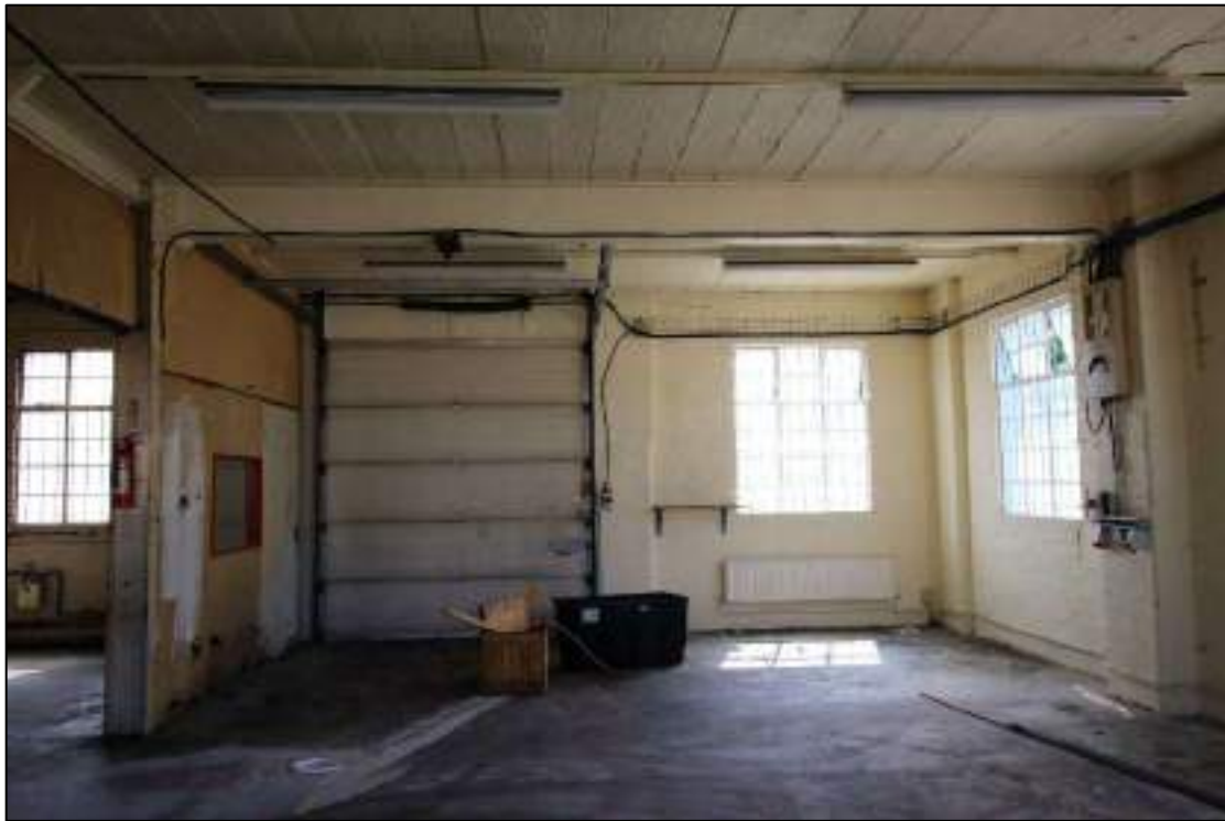
Plate 48: Vehicle entrance at south-west end of front, south-east wall with hanger clamp attached to ceiling beam, looking south-east
