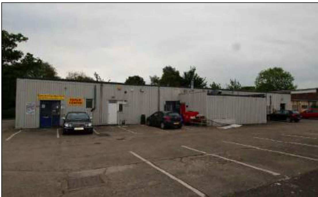
Plate 13: Rear, south-west elevation of Building 1, looking north-east
