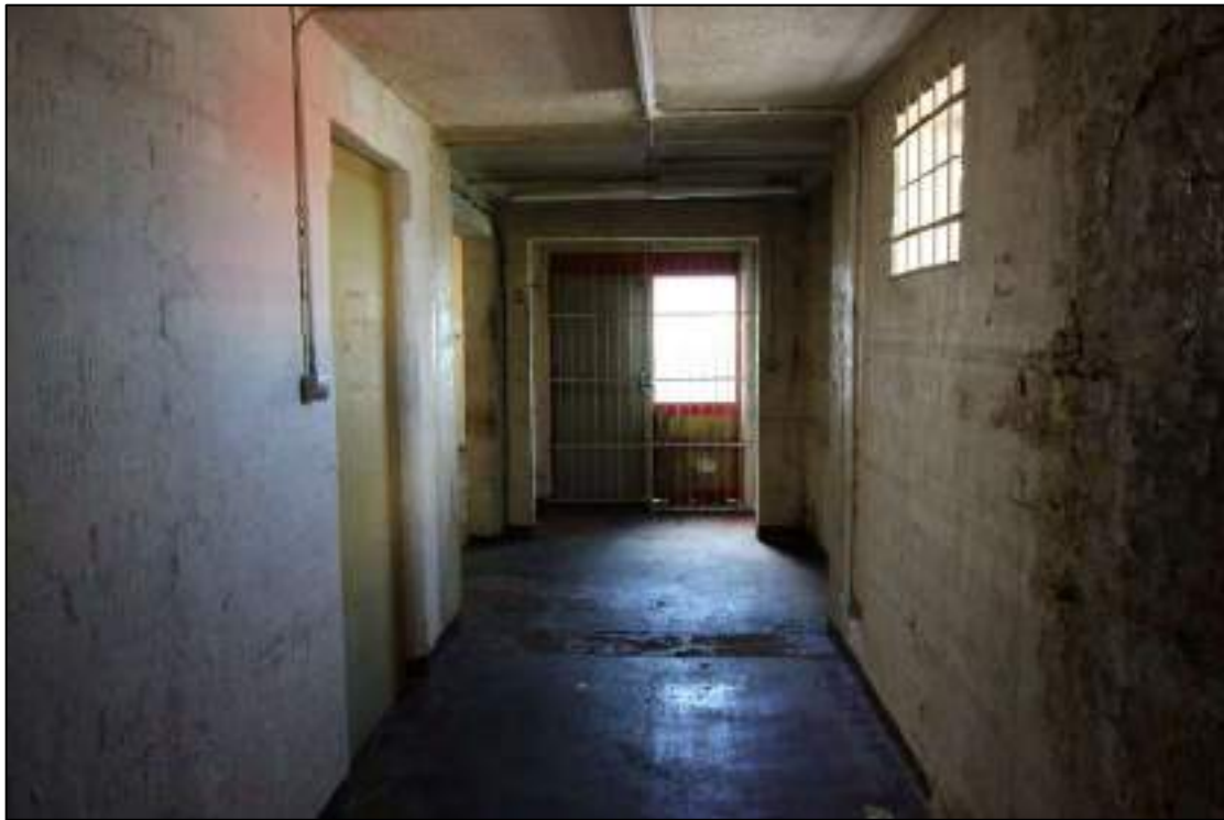
Plate 49: Interior of rear lean-to, looking south-west towards double doorway
