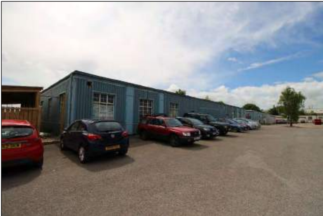
Plate 39: Oblique view of north-east end elevation and rear, north-west elevation of Building 4
