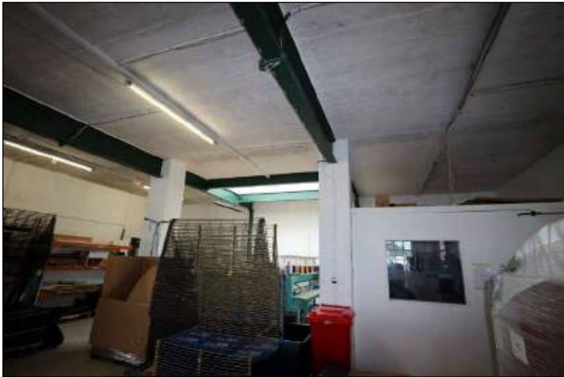
Plate 70: Interior of north-west half of Building 8, looking south-east toward centre division and skylight
