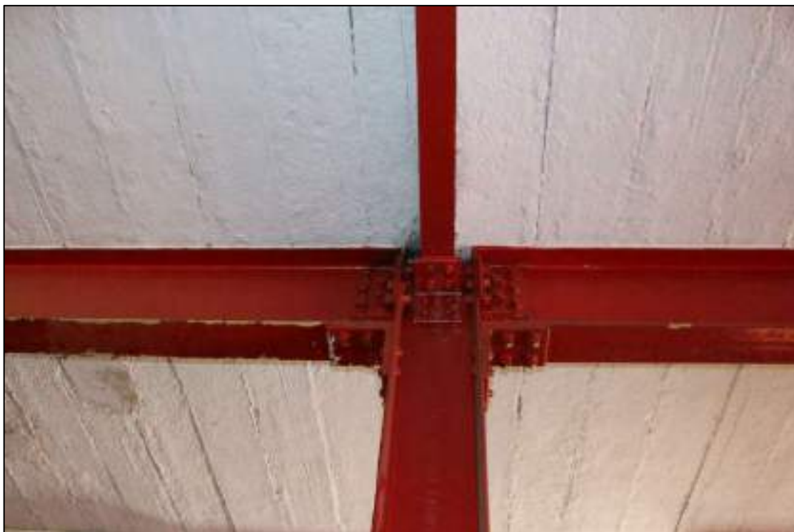
Plate 72: Detail of bolted angle brackets between steel columns and beams
