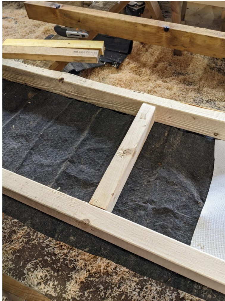
Figure 4.1. Mock up of new timbers to be added to sandwich the bitumen hessian lining
