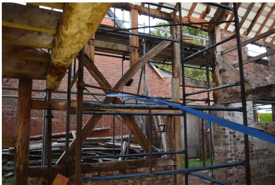
Figure 3.3. View from interior through eastern elevation (Aug 2021)
