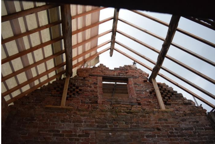
Figure 3.4. Southern gable end (Aug 2021)
