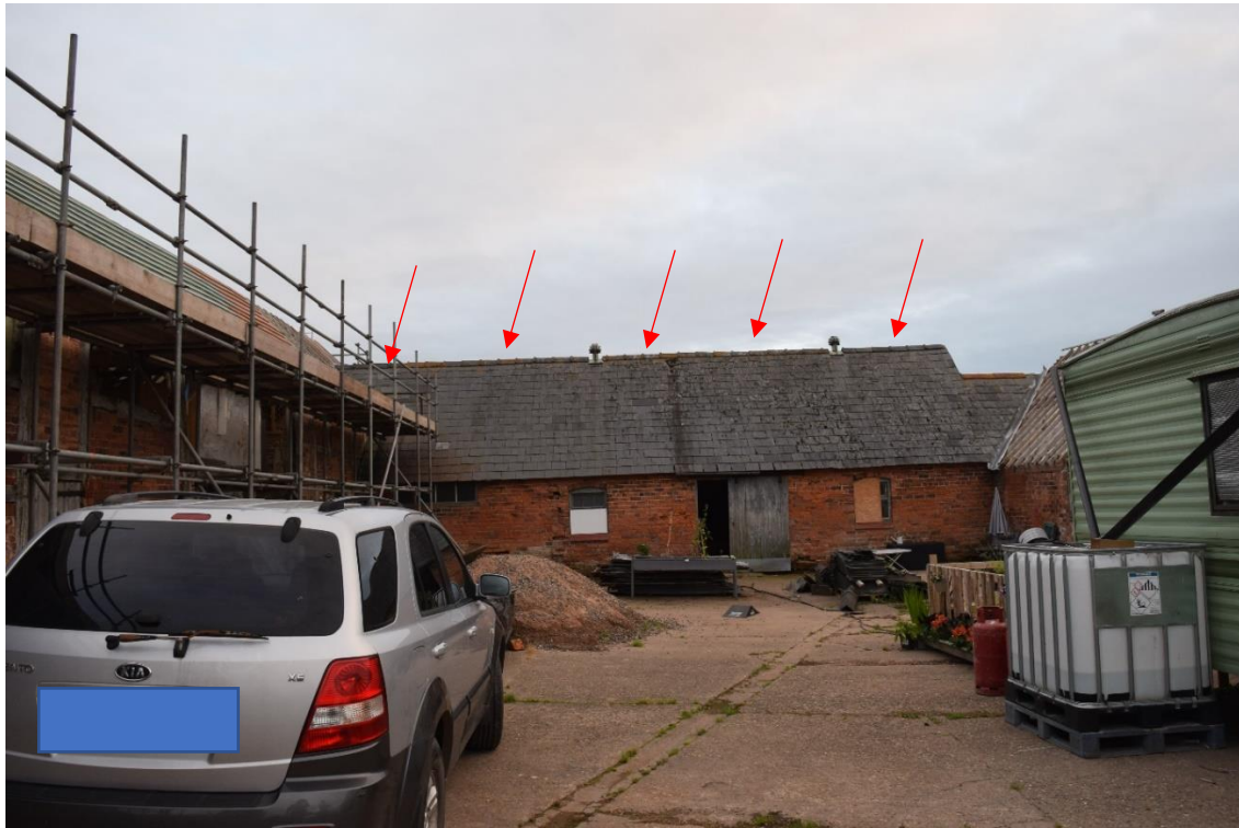
Figure 4.8. Showing approximate positions of bat access under ridge tiles on 1.2
