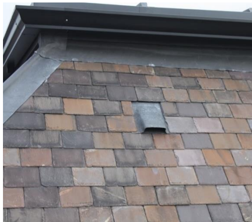
Figure 4.3. Bat access in slate roof constructed from lead.
