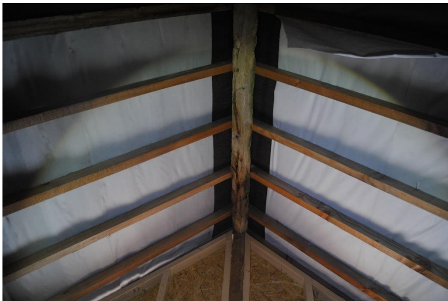
Figure 3.7. View of bitumen hessian along ridge placed above the breathable membrane.
