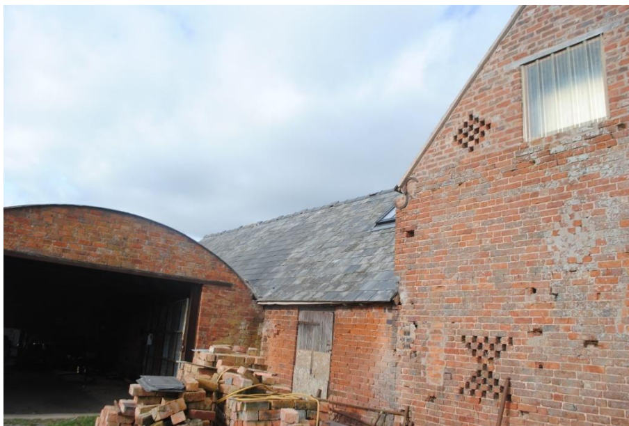
Figure 3.13. View of ridge tiles with vents (Feb 2023)
