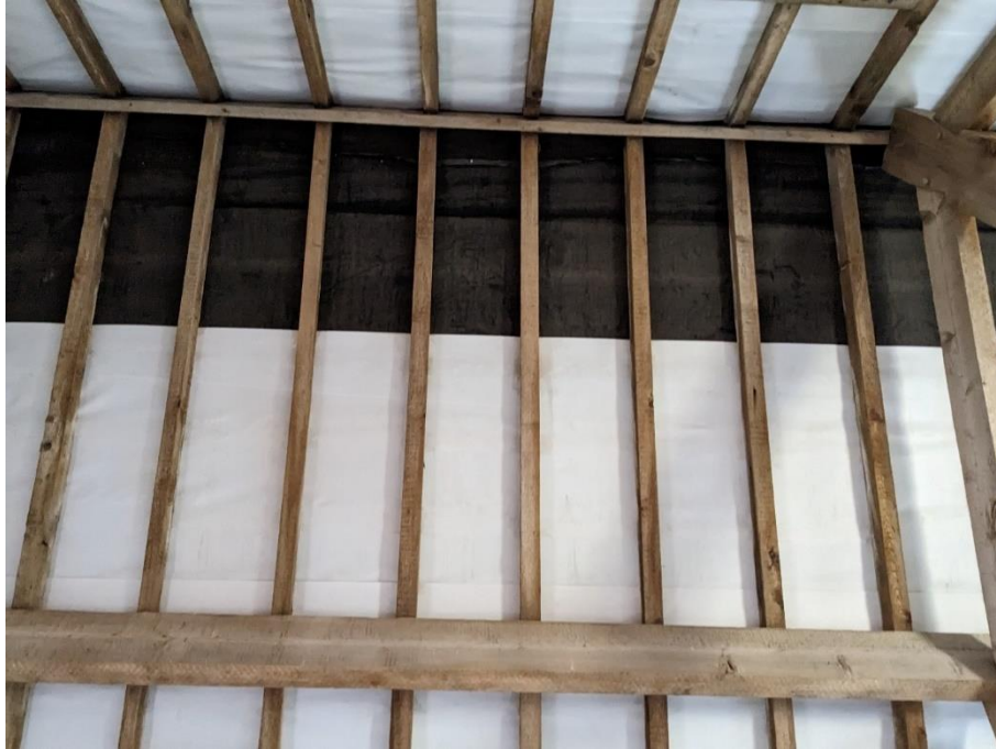
photo showing the existing roof with the BRM (white) and the Bitumen (grey / black)
