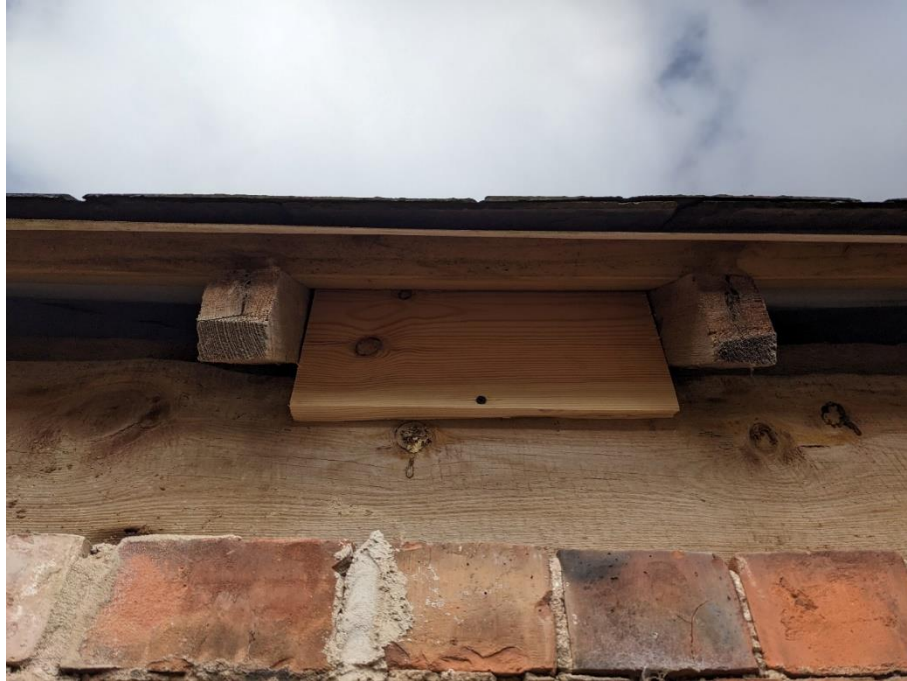
Figure 4.2. Mock up showing bat access to the bottom of the roof being inhibited
