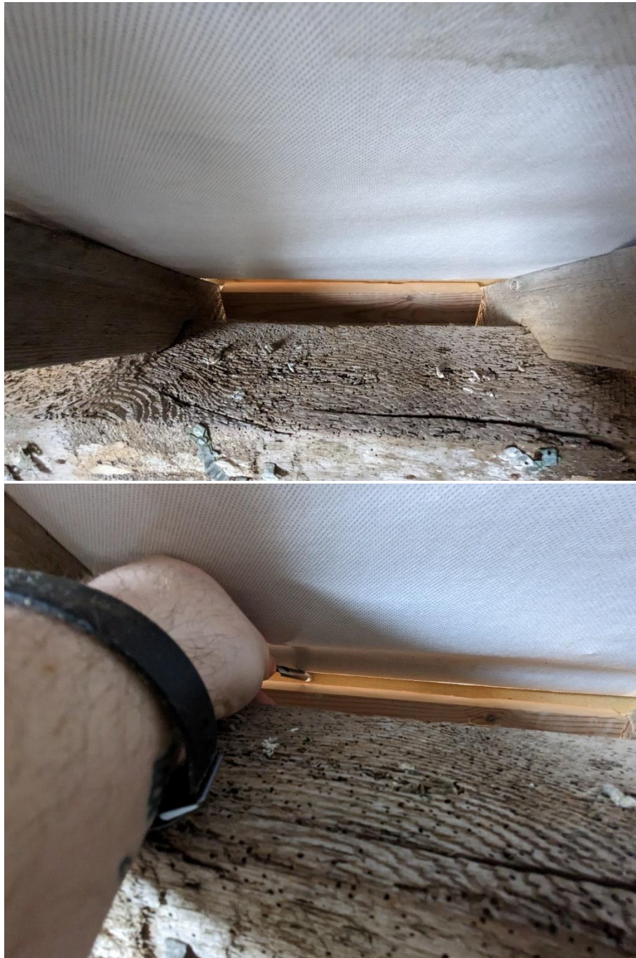
Showing that an 8mm drill bit cannot get through the gap.
