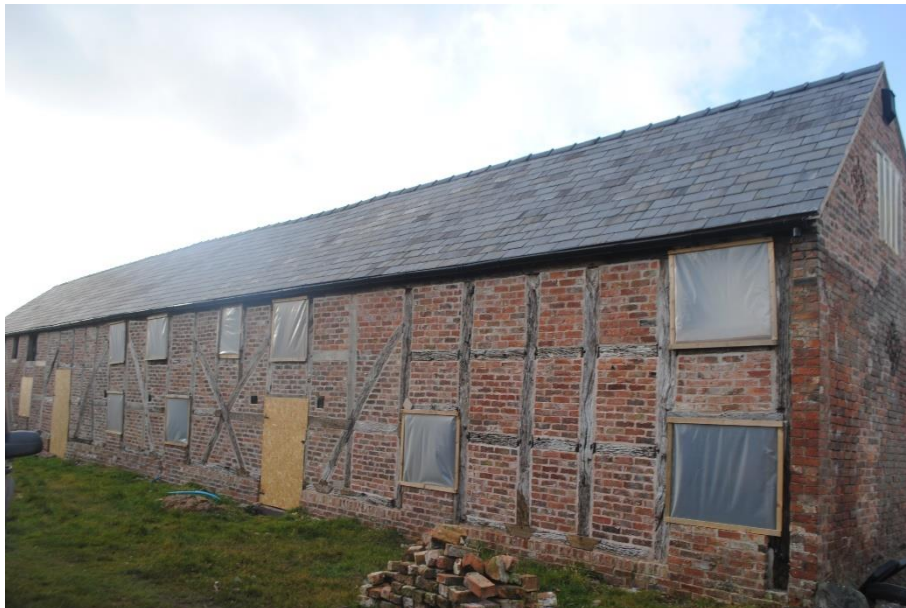
Figure 3.5. Barn 1.1 in February 2023
