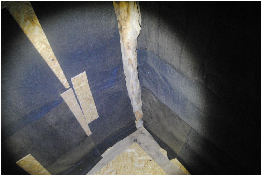
Figure 3.20. Void left for bats in Barn 2.
