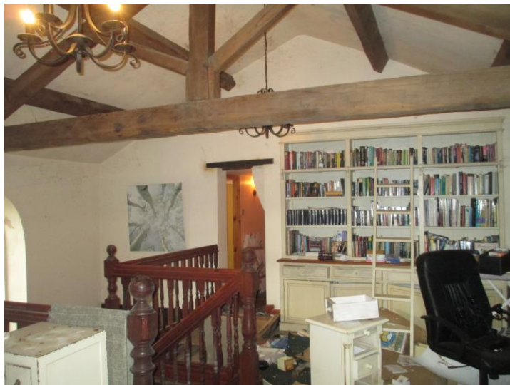
Image 14: Existing trusses to be maintained.
