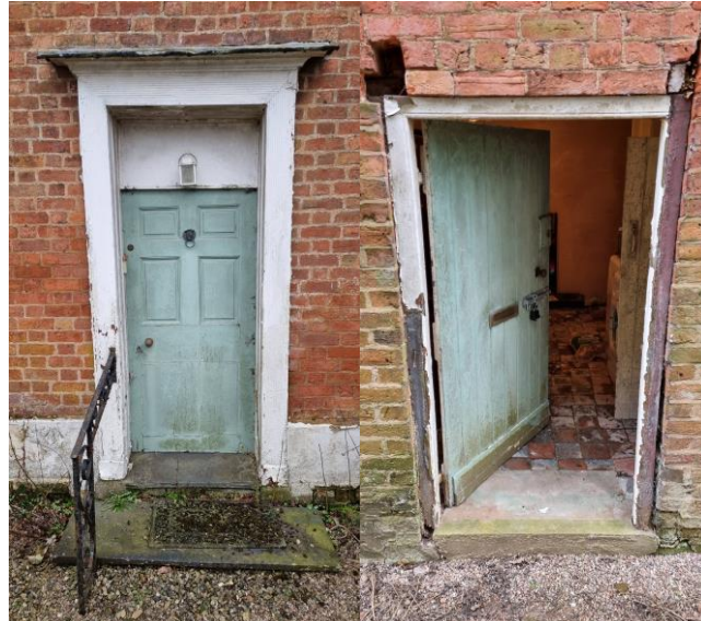
Image 07: Existing front and side door.
