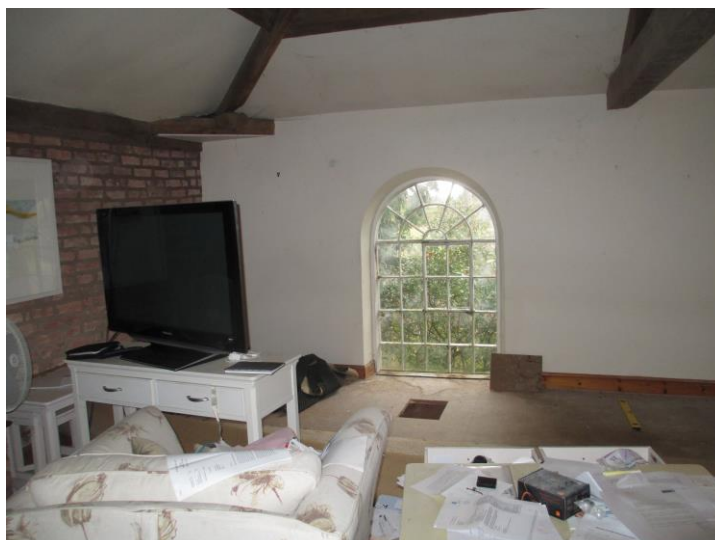
Image 15: Existing first floor visually cutting chapel windows in half.
