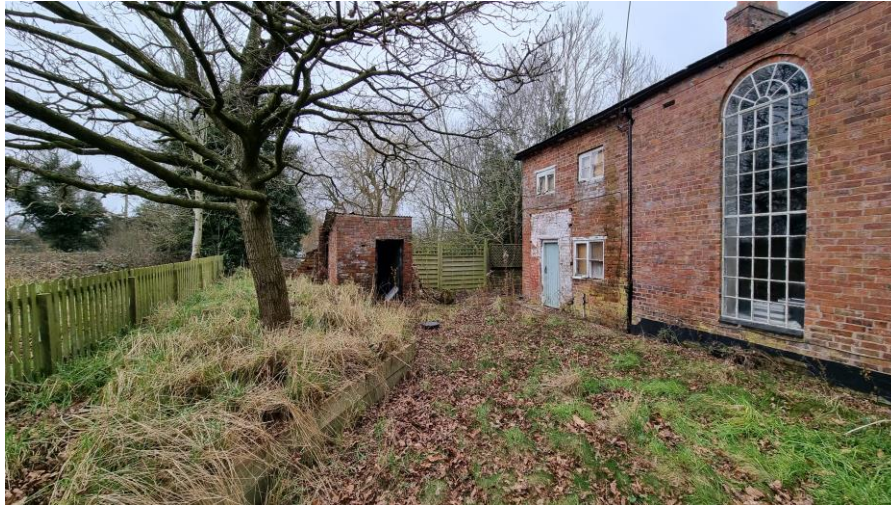
Image 06: Showing existing brick shed at the rear of the property, and overgrown garden.
