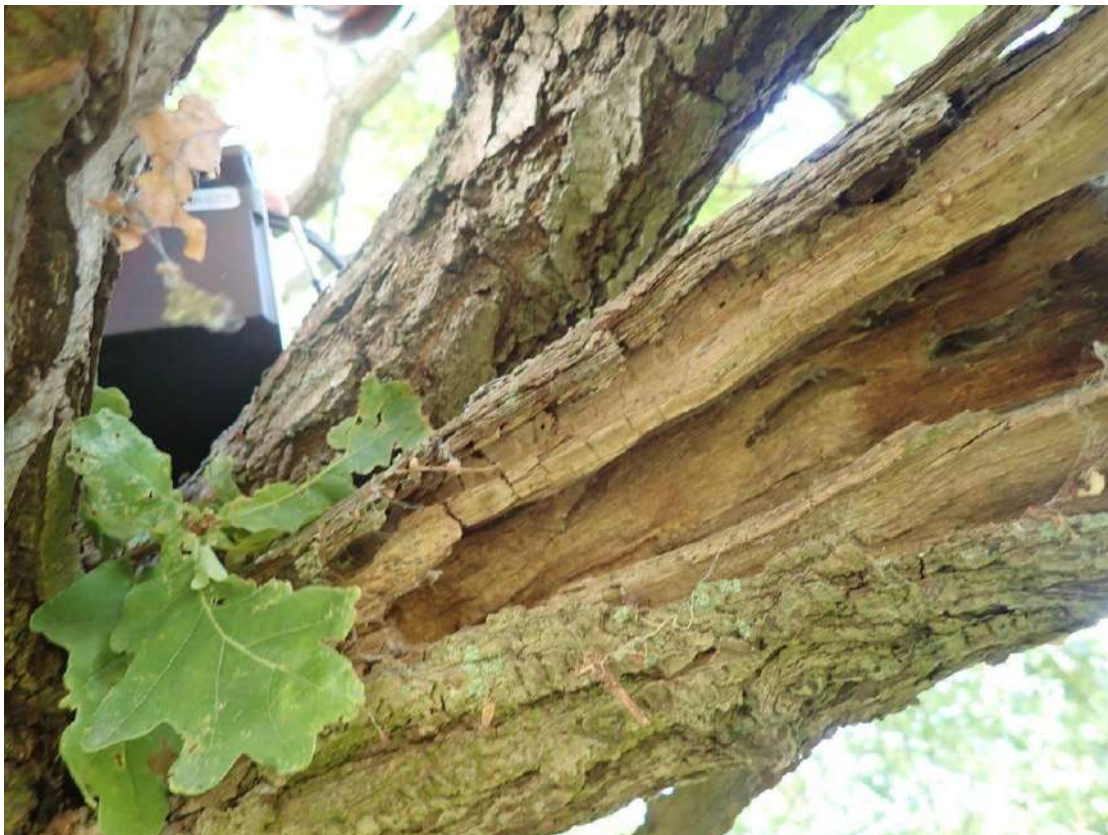
Photograph 36 – T10 showing hazard beam (T10.16).
