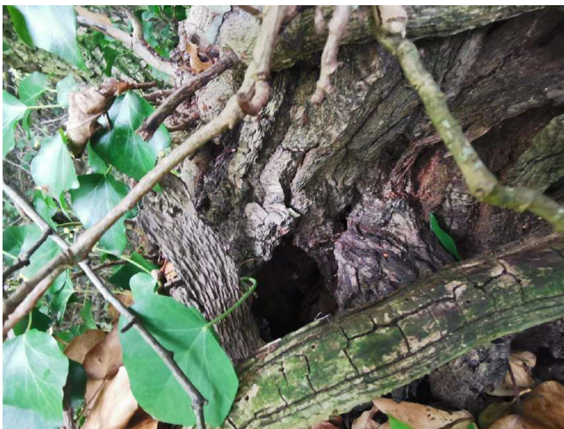
Photograph 17 – T7 showing branch cavity (T7.4).
