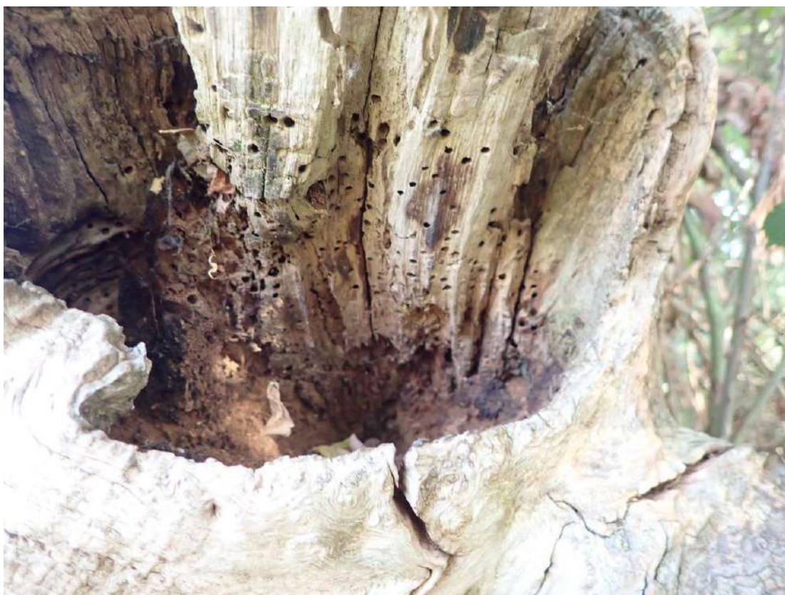
Photograph 5 – T1 showing rot-hole (T1.4).
