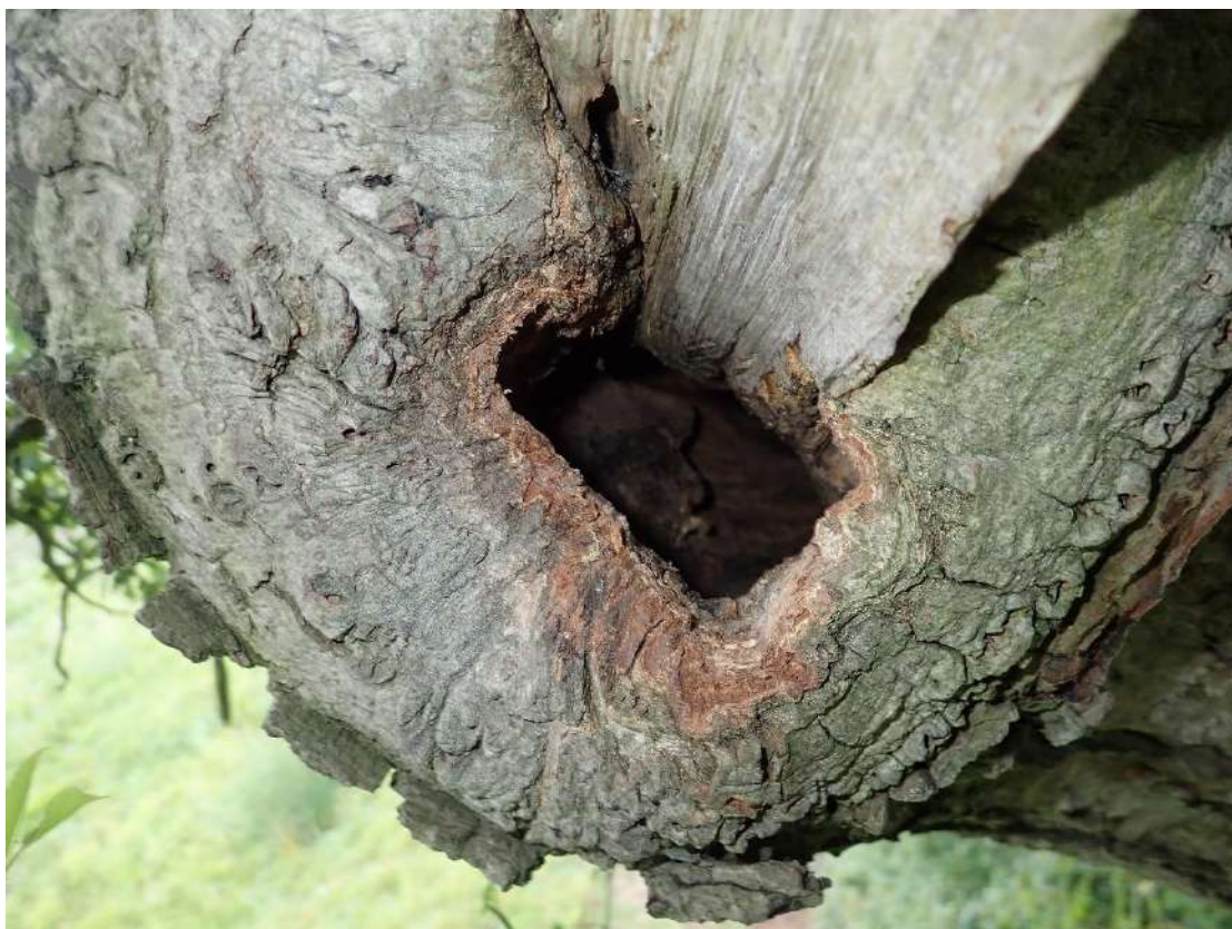
Photograph 14 – T6 showing tear-out (T6.4)
