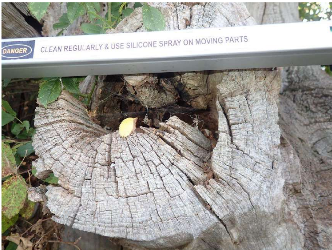
Photograph 4 – T1 showing rot-hole (T1.3).
