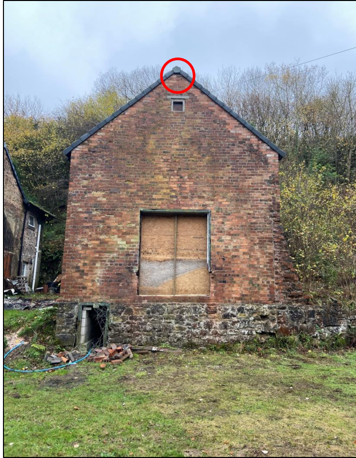
Figure 5.3 – Visual aid – Emergence point beneath at apex of the northern gable, from which a single Common Pipistrelle emerged during the Dusk Survey on 31/08/2022
