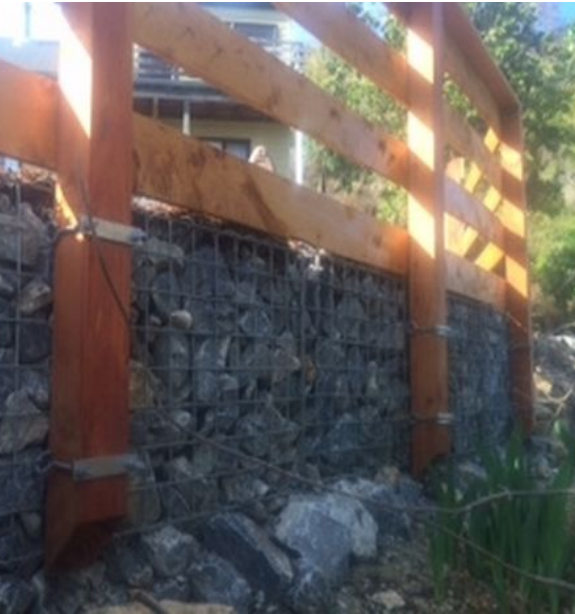
Post and rail fence above gabion baskets.
