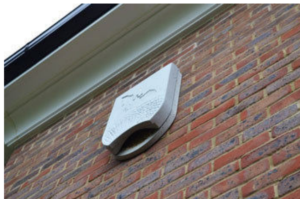
Figure 12: Schwegler (1WQ) bat box fitted to wall.
