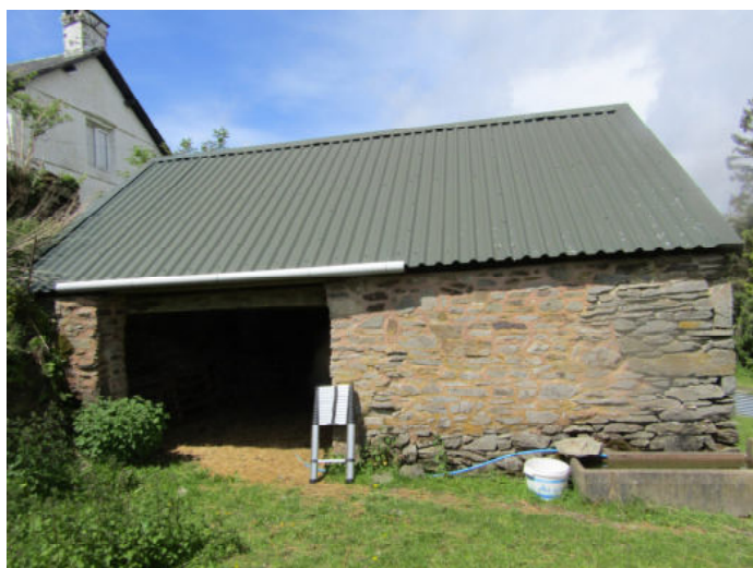
Photo 3: East elevation of barn.
