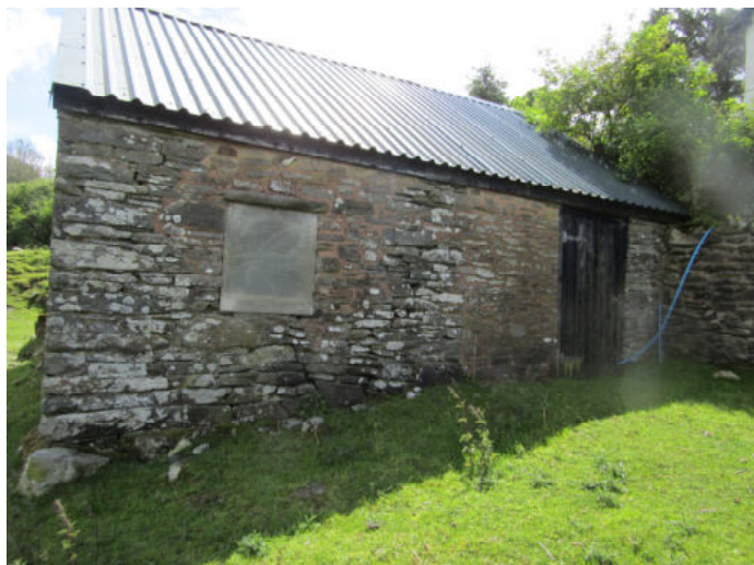
Photo 1: Galvanised roofing sheets on roof.
