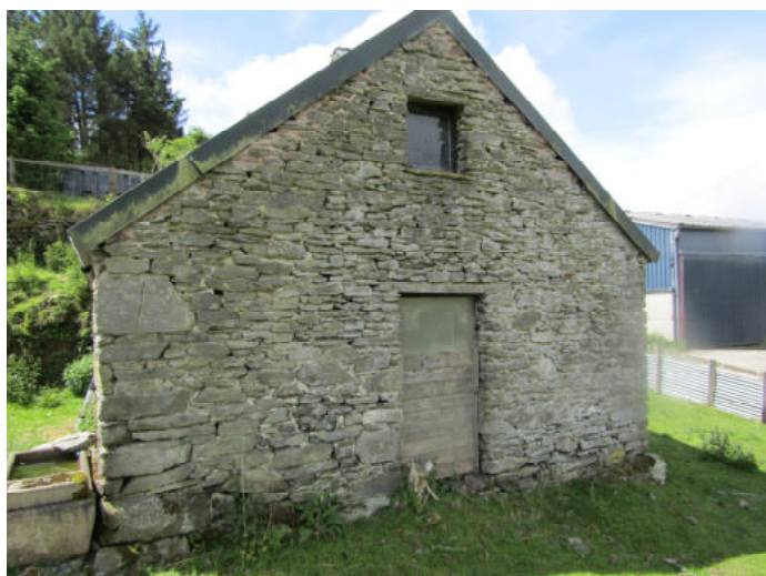
Photo 2: North gable-end of barn.
