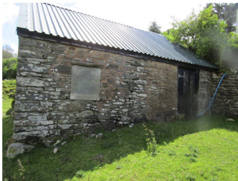
Barn at Hen Hafod.
