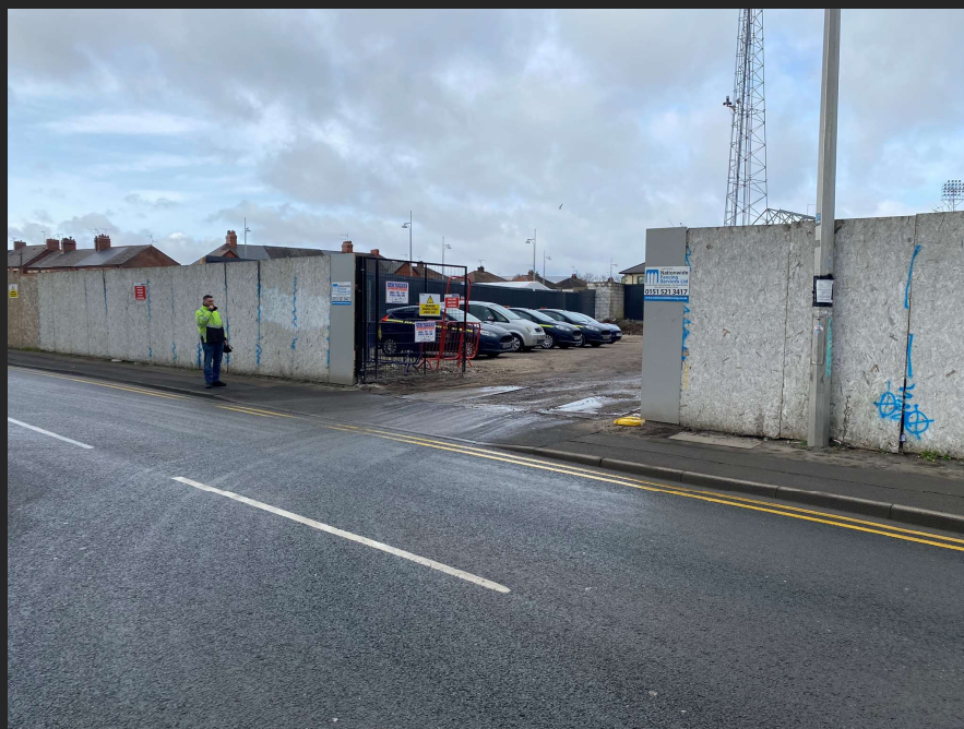
Crispin Lane Entrance through Hoarding – 5m wide
