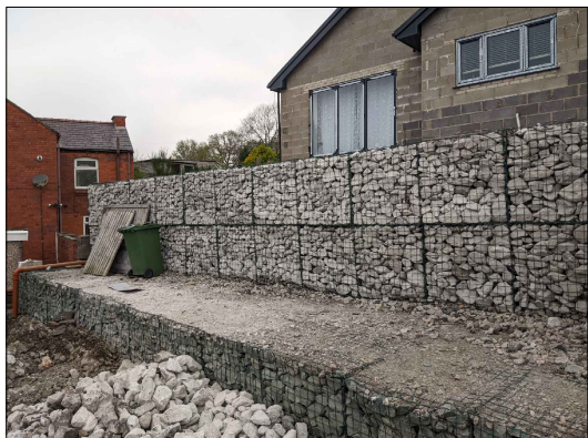
Ref 2 - Gabion Baskets
