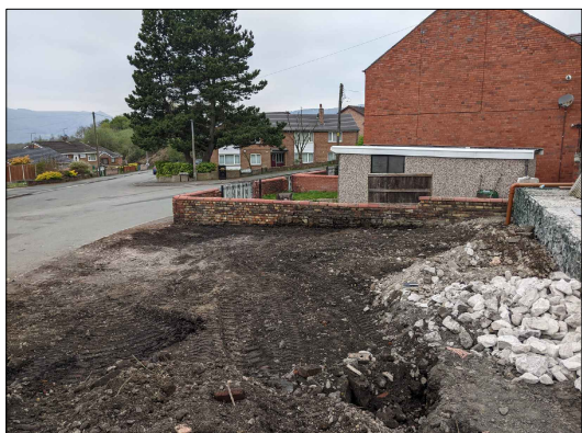
Ref 3 - Existing Boundary Wall (to remain)
