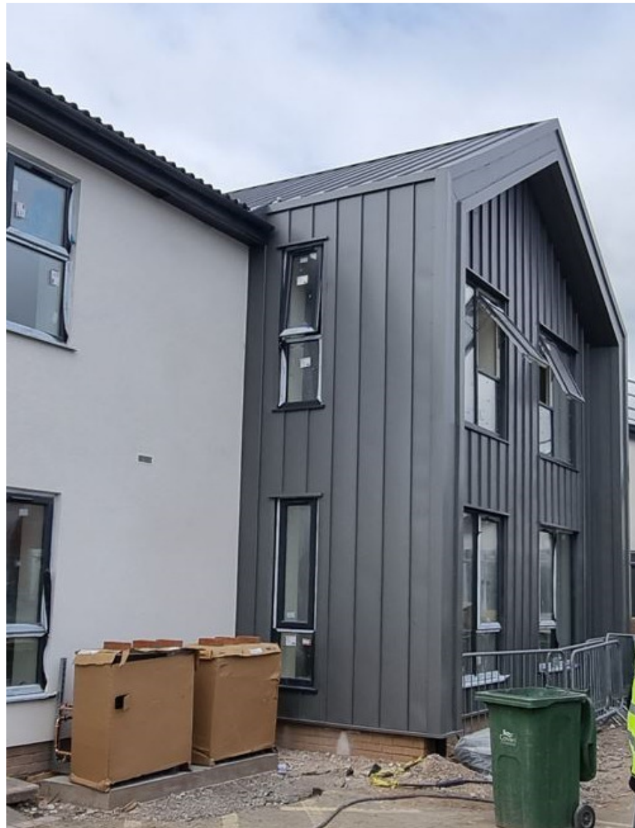
Plinth, cladding and render
