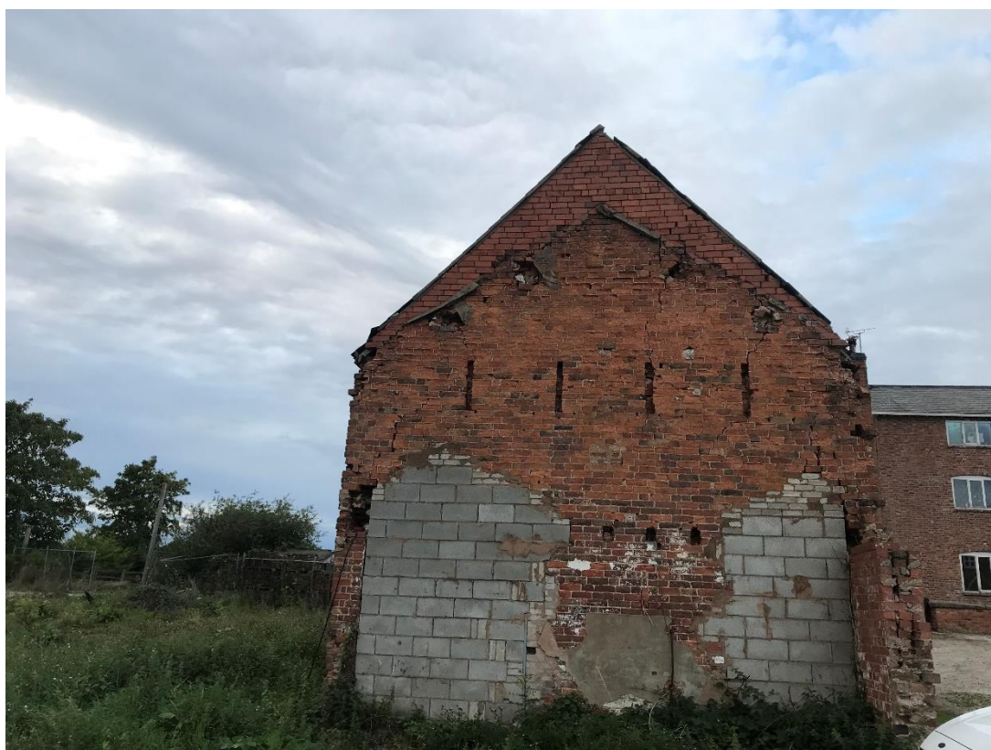
Plate 2 – Southern elevation of the barn
