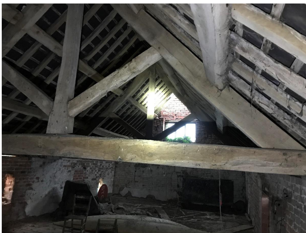
Plate 4 – Character of the loft of the barn, showing roofing timbers and empty window frame at the northern gable
