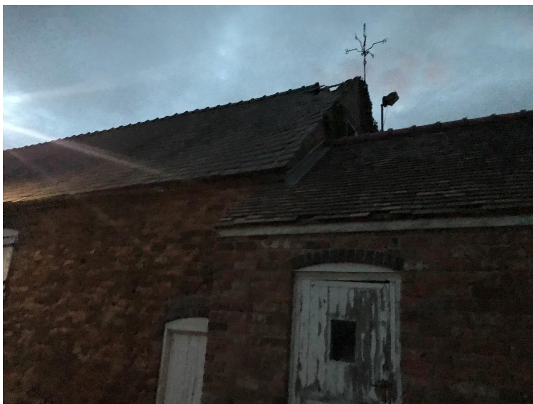
Plate 6 – Northern gable of the barn
