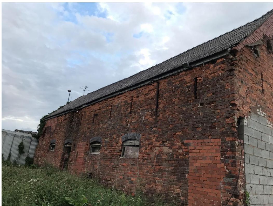
Plate 3 – Western elevation of the barn
