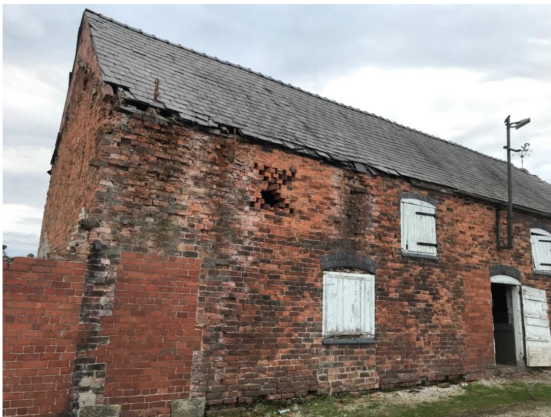
Plate 1 – The Barn at Middle Sontley Farm, as viewed from the south-east
