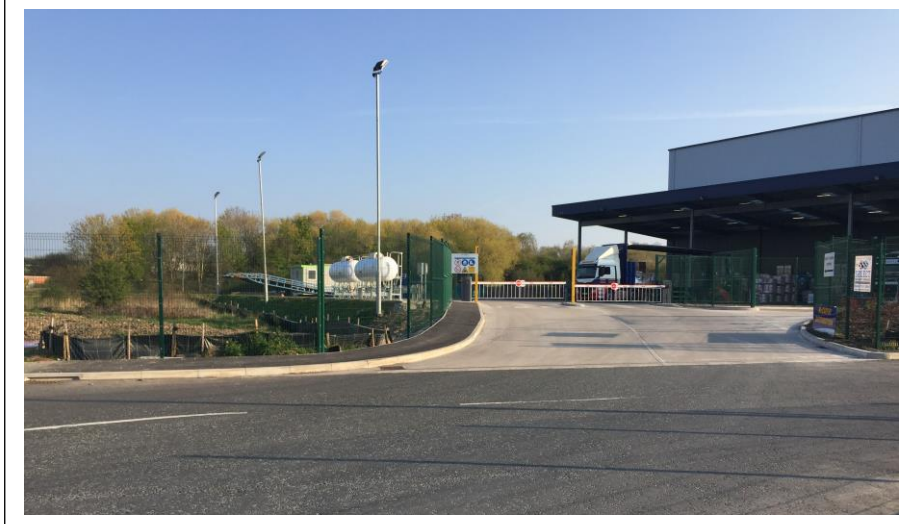
1 – General elevation of site from Abbey Road.
