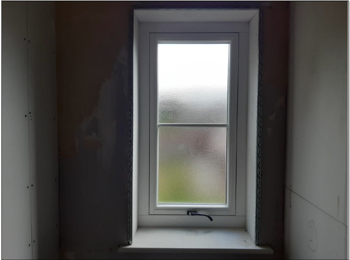
Additional North-West Facing Window
