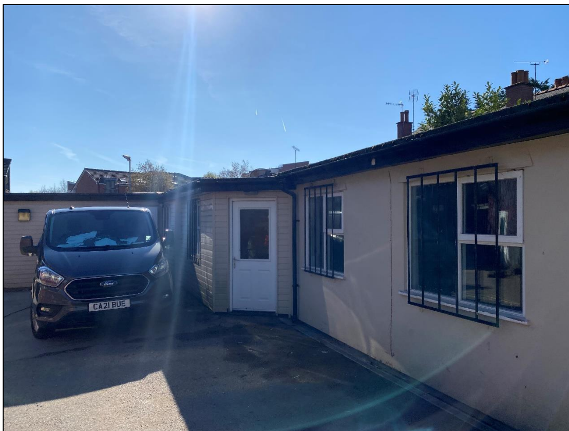
Plate 11 – Northern elevation of B4
