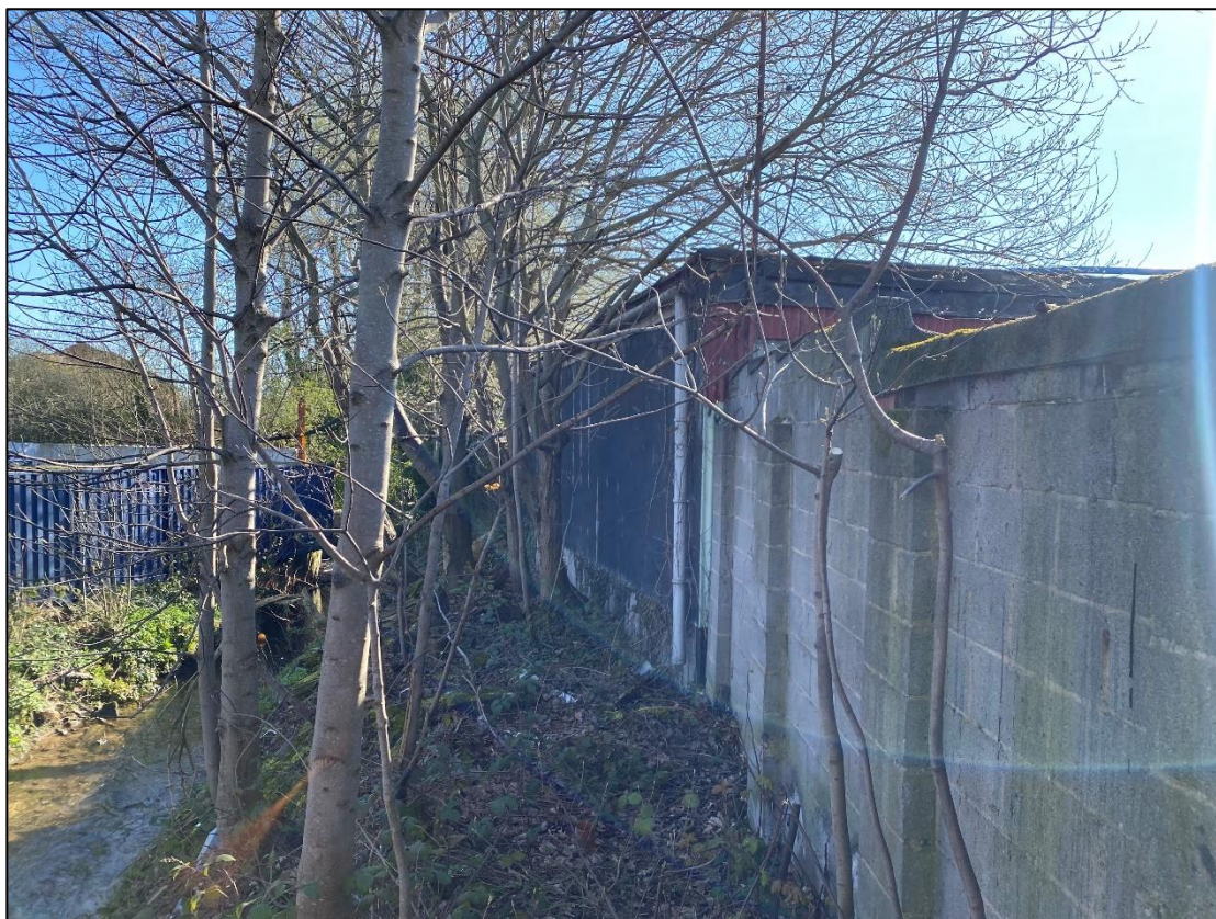
Plate 10 – Rear elevations of B2 and B3 and tree line along the river Gwenfro
