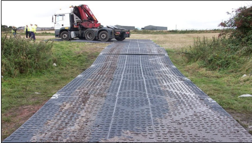
P1 – Example of ground guards used for plant access within RPA of trees
