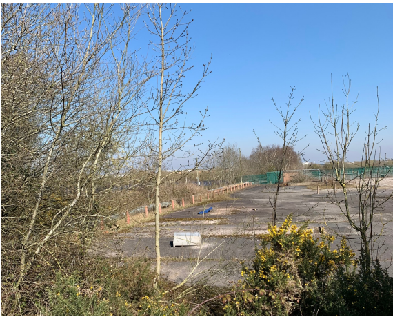
Former gasometer - Exterior Image
