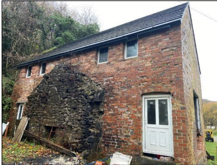
Figure 7.1 - Exterior of the Barn from the East
