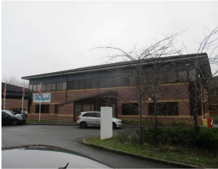
Front elevation of Unit G, Yale Business Centre
