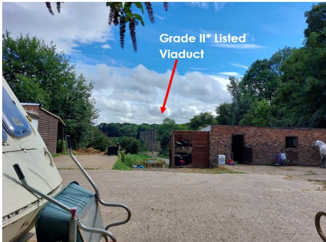
Figure 7. Photograph taking from the front door of the current building, demonstrating the distance from the Grade II* Listed Viaduct.
