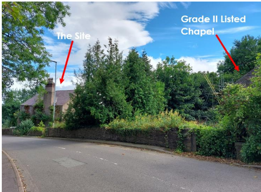
Figure 6. Photograph taken on Newbridge Road showing how the two buildings cannot be seen from one another. The photograph also shows how the current buildings condition impacts the road negatively.
