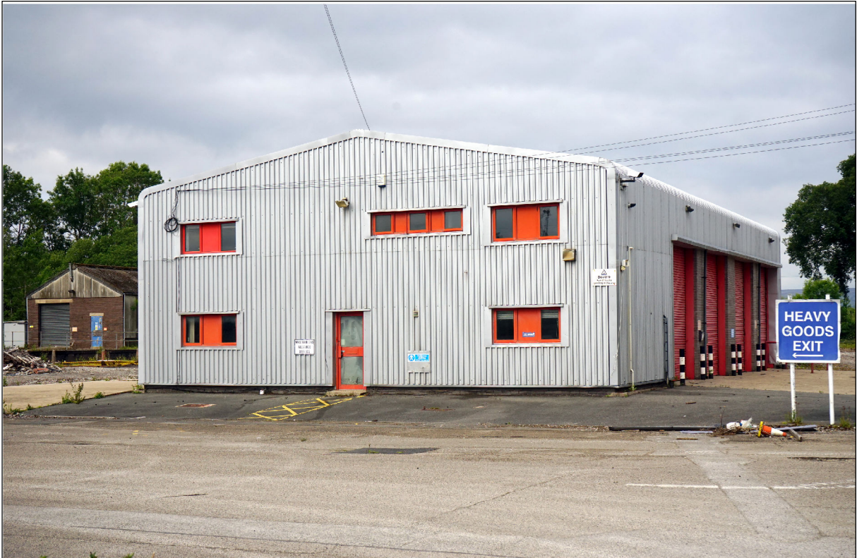
Plate 13) Modern depot building, facing southwest
