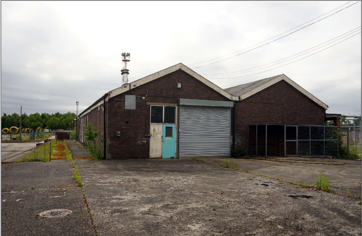
Plate 7) View of the west elevation of ROF Marchwiel Case Store 28/233B, facing southeast
