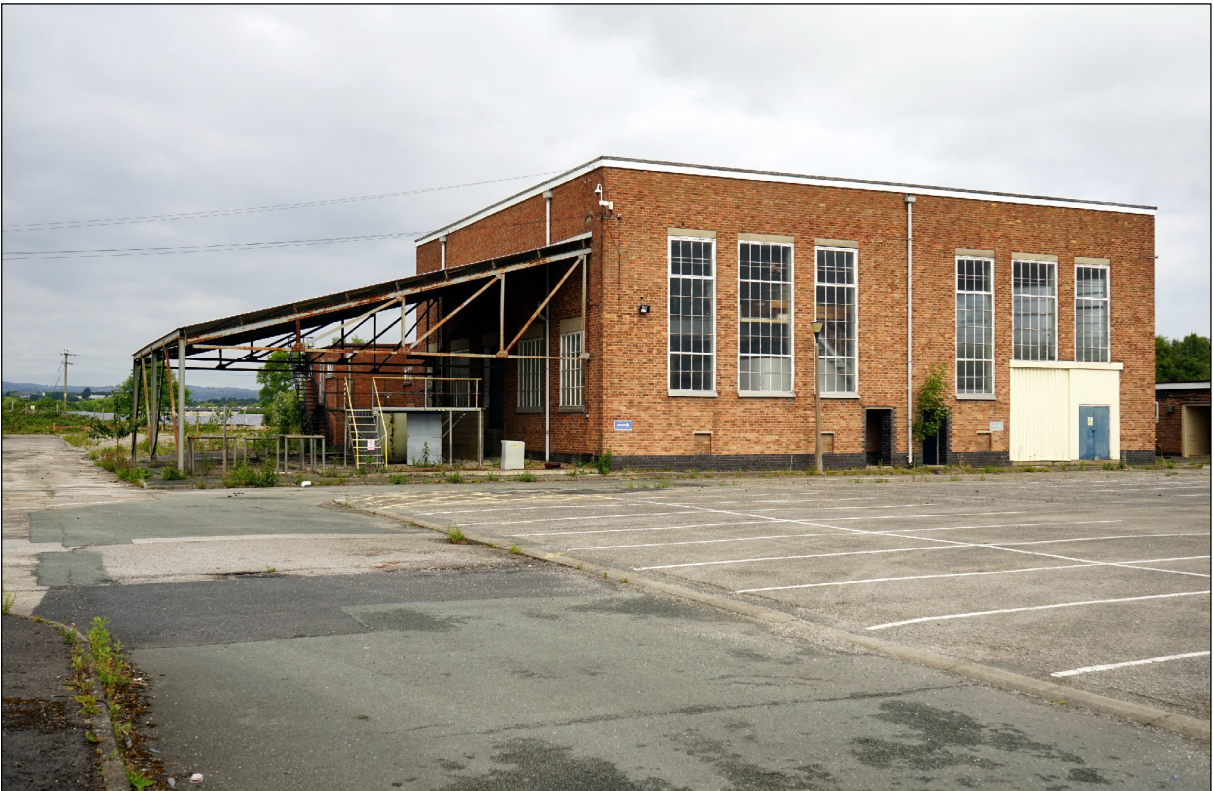
Plate 8) Maelor Works Plant Building, facing northwest
