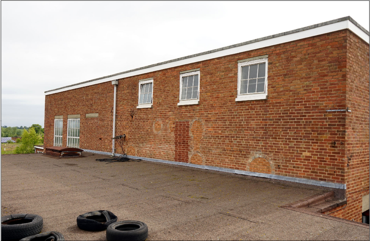
Plate 9) View of the rear first-floor elevation of the Maelor Works Plant Building, facing northeast
