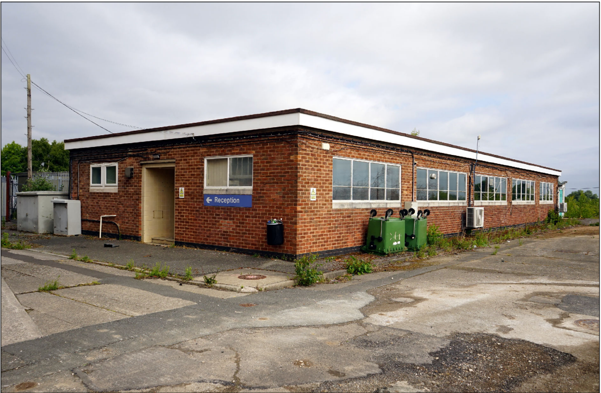
Plate 10) Maelor Works Administrative Building, facing northwest
