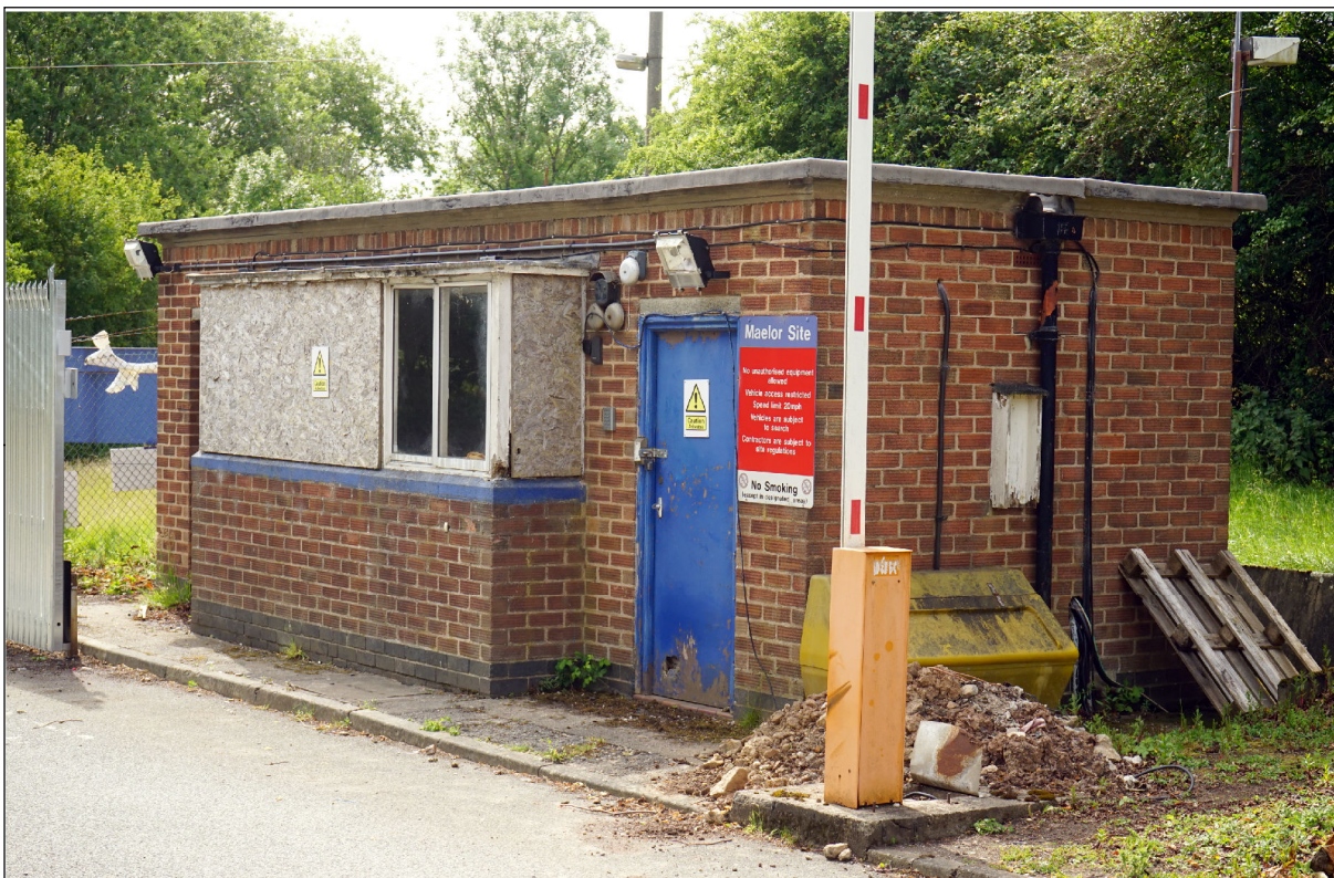
Plate 11) Maelor Works guard room located on the main access road, facing southeast
