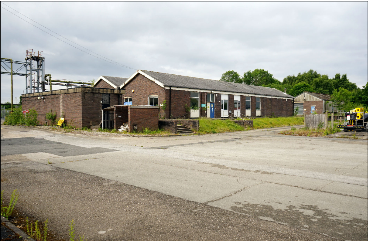
Plate 6) ROF Marchwiell Case Store 28/223B with modern ancillary structure, facing southwest
