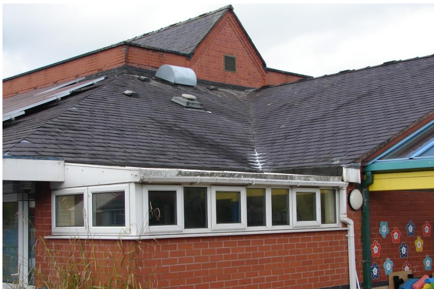
Northeast gable end.
