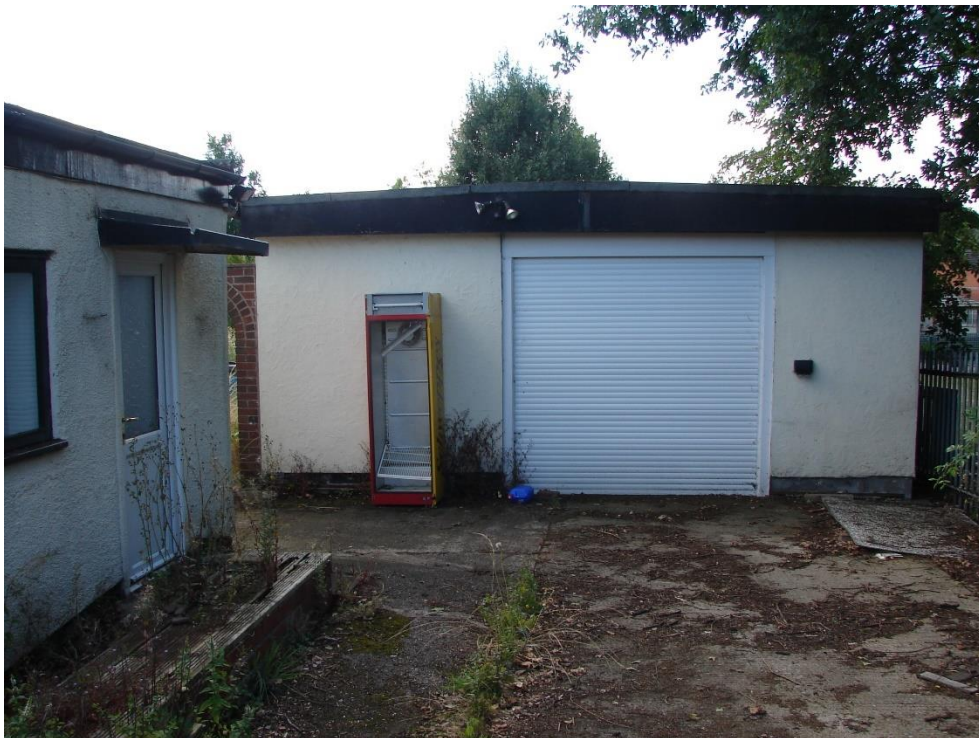
The northern elevation of the garage ( Target Note 10 ).
