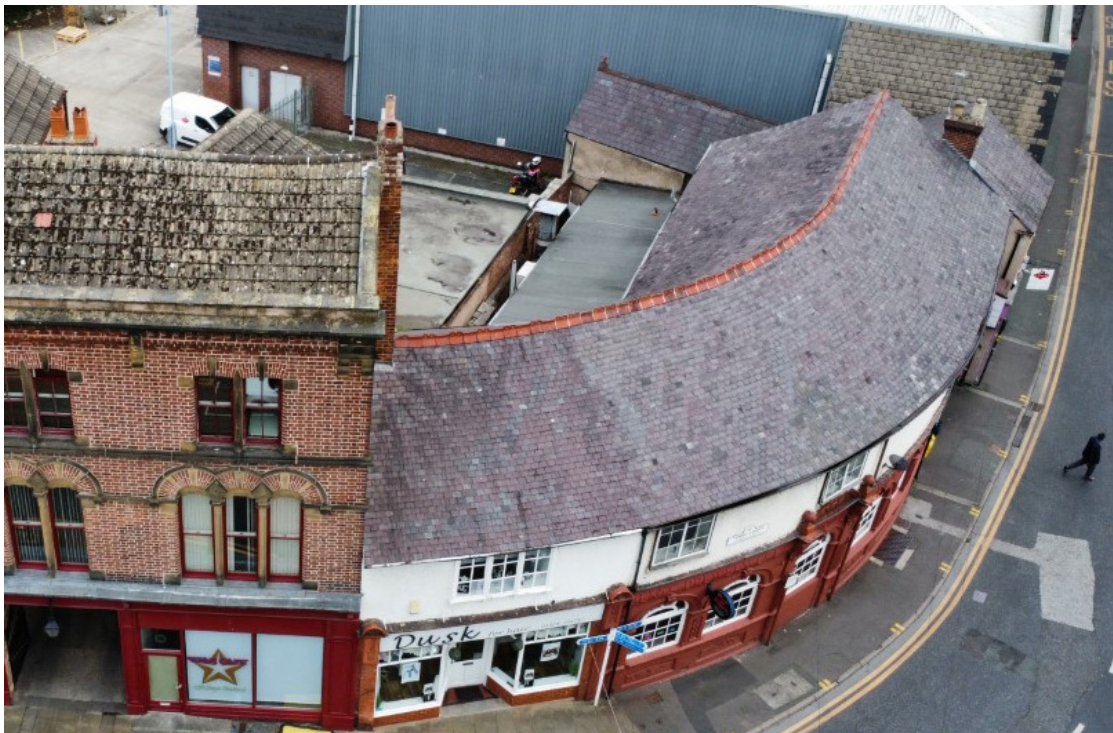
Drone photograph from the north west looking south east across the front elevation of the building.
