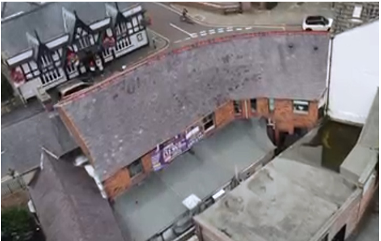
Aerial view of the rear facing roof slope post-development.
