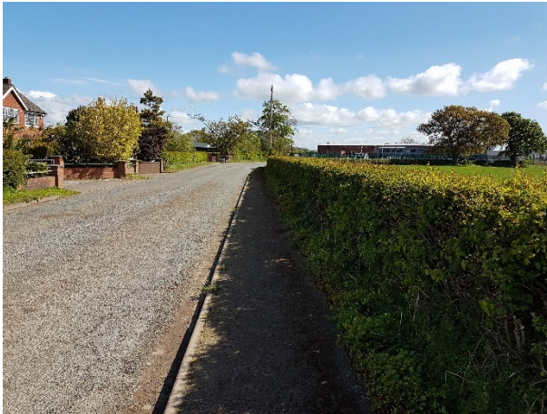
Figure 4.2: Footway on Pickhill Lane
