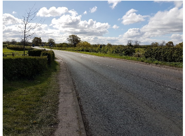
Figure 4.3: Footway on A525
