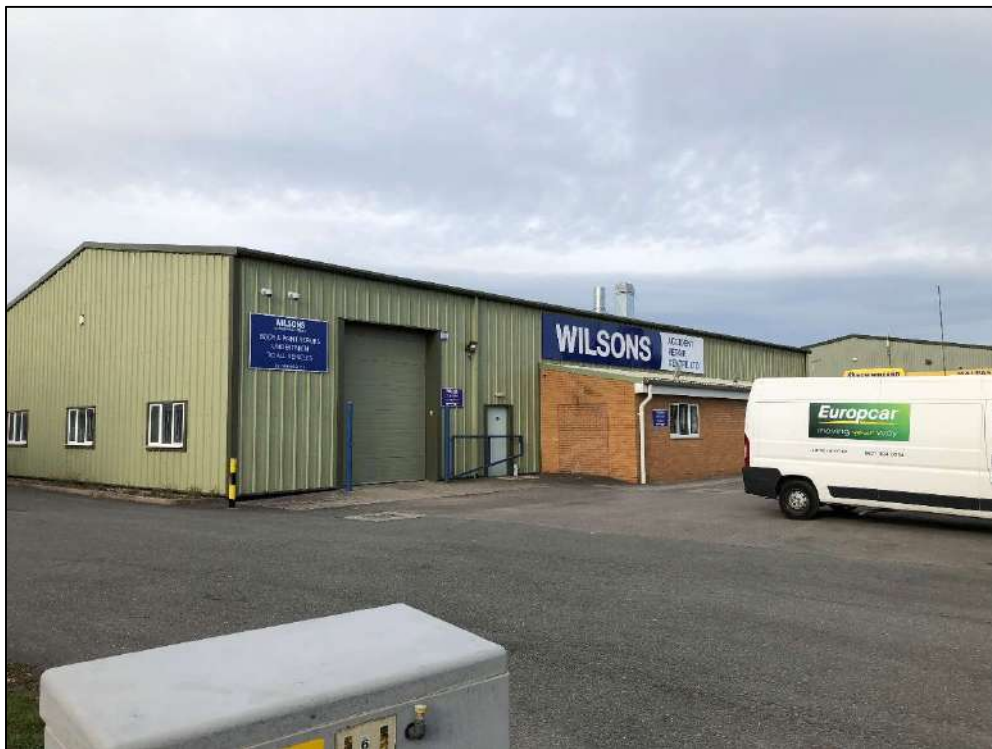
Plate 23: View north west showing the industrial unit operated by Wilsons Accident and Repair Centre.
