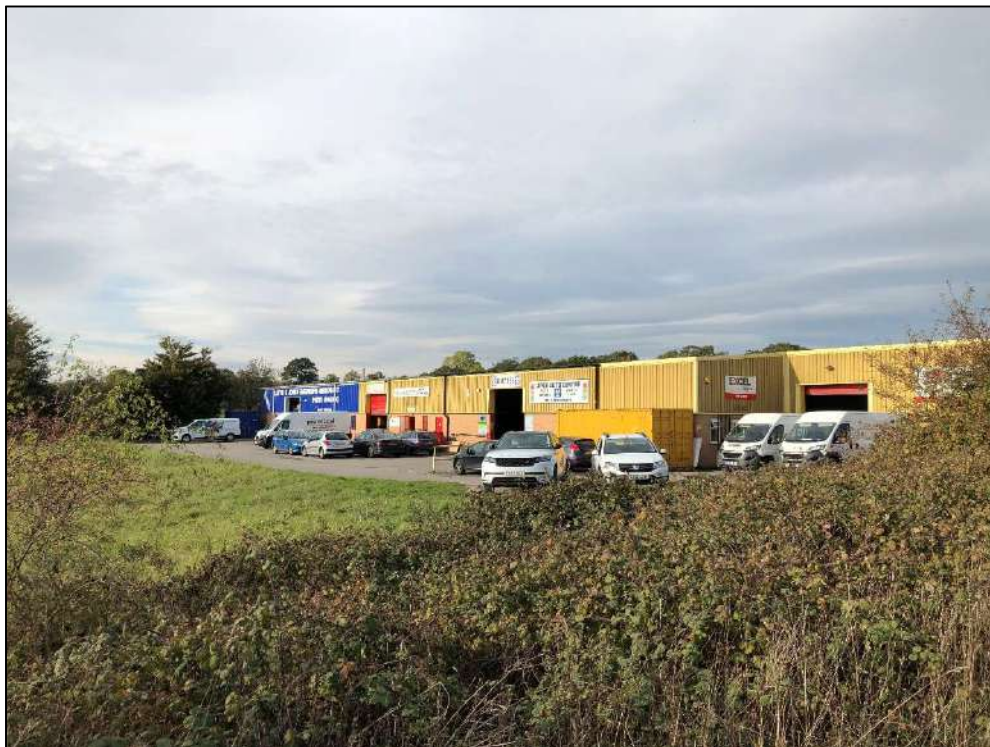
Plate 19: View north east showing the industrial unit to the south west of the site.
