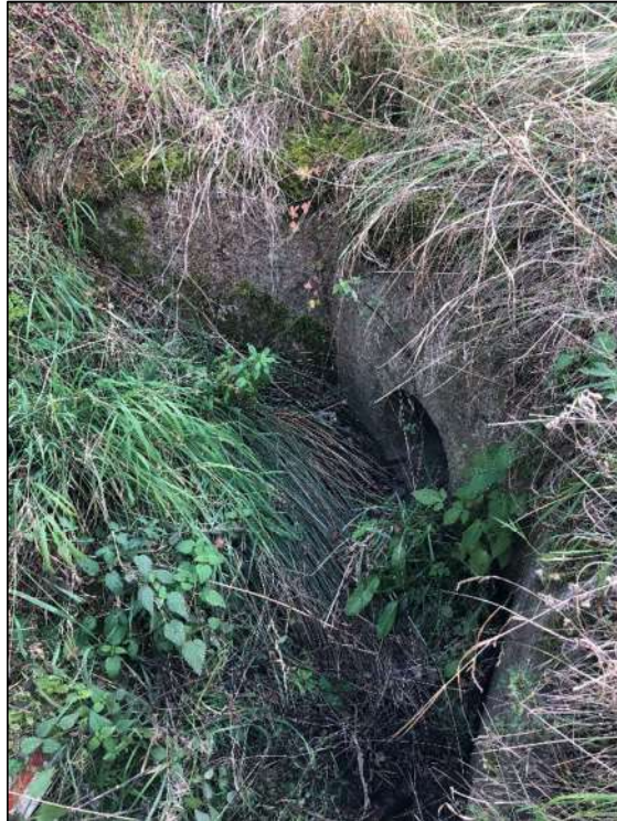
Plate 17: View showing the culvert adjacent to the sites southernmost section.
