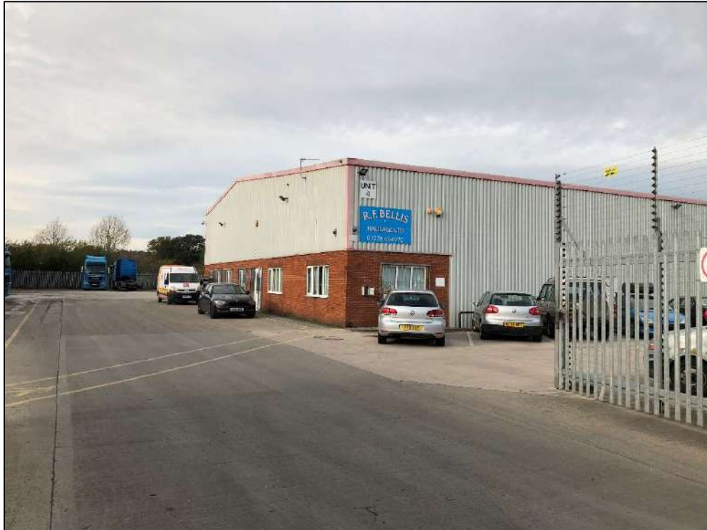
Plate 22: View west showing industrial warehouse being operated by R.F. Bellis Haulage Ltd.
