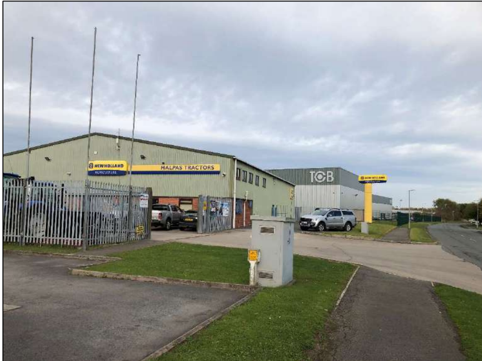
Plate 24: View north west the industrial unit operated by Malpas Tractors beyond which lies the large warehouse operated by Tension Control Bolts Ltd.
