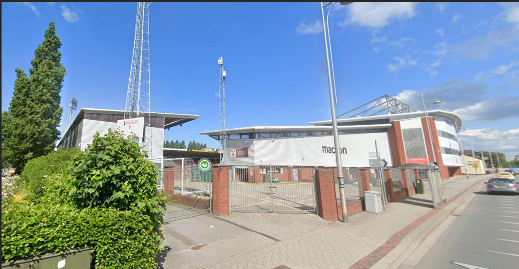
The entrance to the yard/car park for the for the first column base to be completed.
