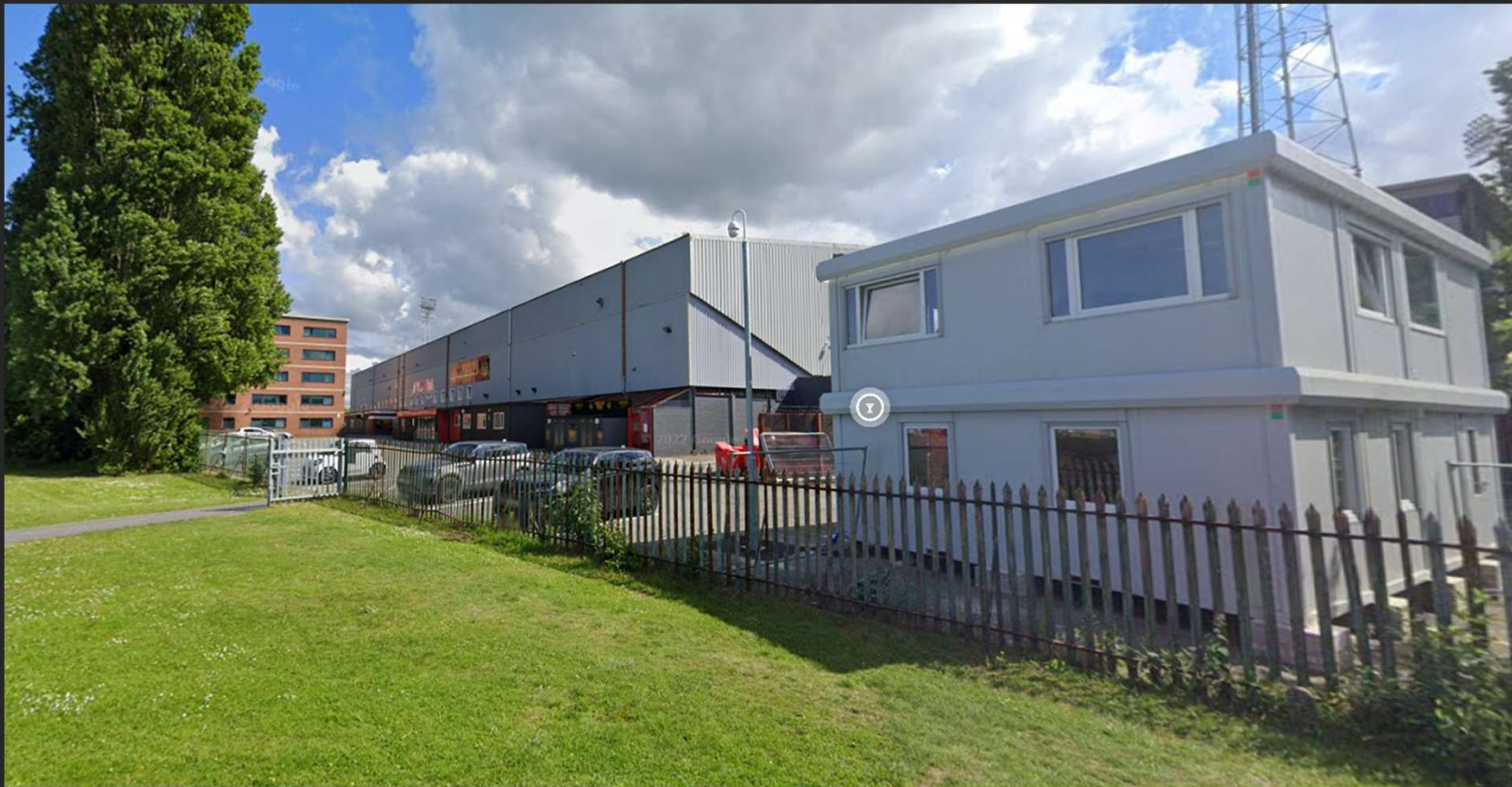
A view of the club car park and additional club offices
