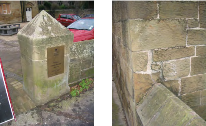
Plate 38 & Plate 39 Entrance Pillar, which has been reduced in height. Evidence of the original (1896) wall height on the Court No. 2 Entrance.
