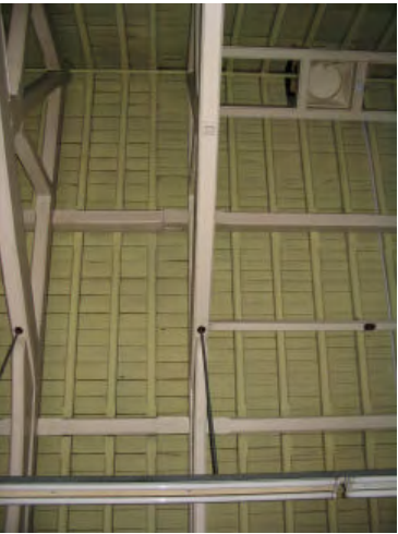
Plate 8 The difference in boarding sizes illustrates the original extent of the Regimental Store. The 1857 boarding being much wider
