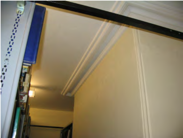
Plate 19 Original (c.1896) corning and moulding to chimney breast. The modern ductwork can be seen in the rear of the photograph.
