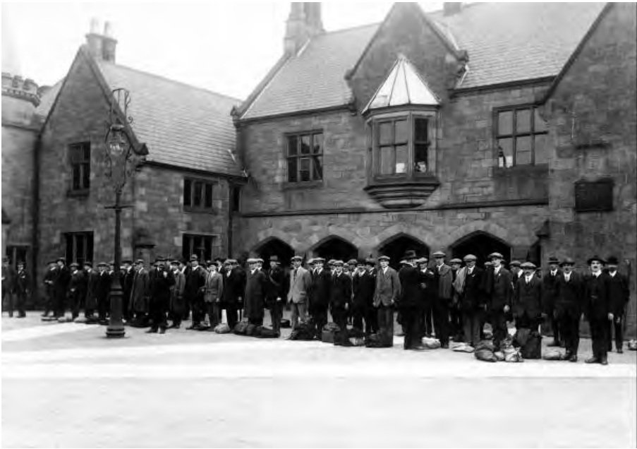
Plate 35 The entrance front c.1914. This view has changed remarkably little. The diamond pattern casements have been replaced largely in single panes and many of the hopper and pivot lights still survive today.
