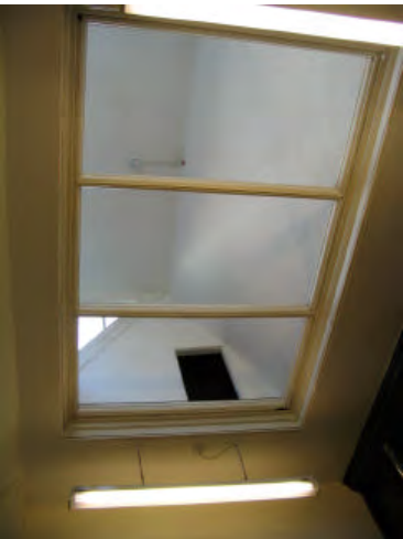
Plate 15 Lay-light showing framing for glass panels.
