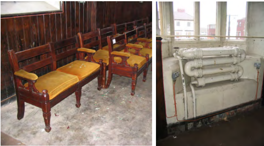
Plate 23 & Plate 24 Court room furniture stored in Court 1. To the right, 19 th century heating pipes to the oriel window.
