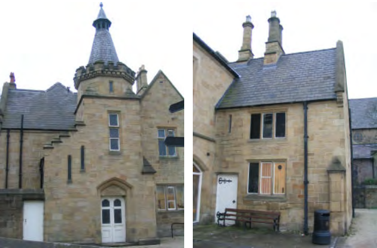
Plate 31 & Plate 32 Entrance to Court 2 (1896) and blank window to F23. Tooling is visible behind the central pane as noted in the text.
