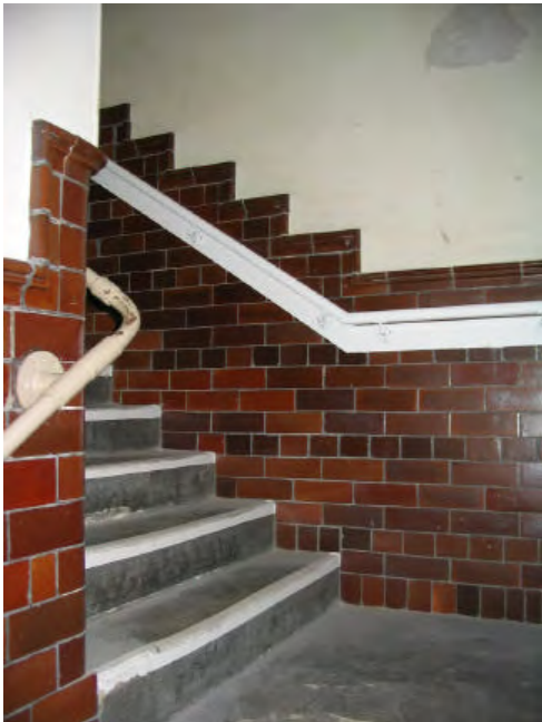
Plate 20 Glazed brickwork, original and modern handrails to G40.
