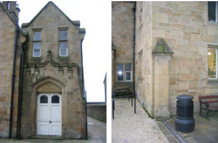
Plate 33 & Plate 34 Entrance to Court No.1 showing the more restrained detailing. To the right, the piers which were to form a boundary with railings to the front of the building, but there is no evidence it was installed beyond these piers.
