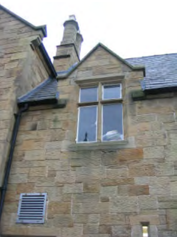
Plate 9 Dormer window added c.1917
