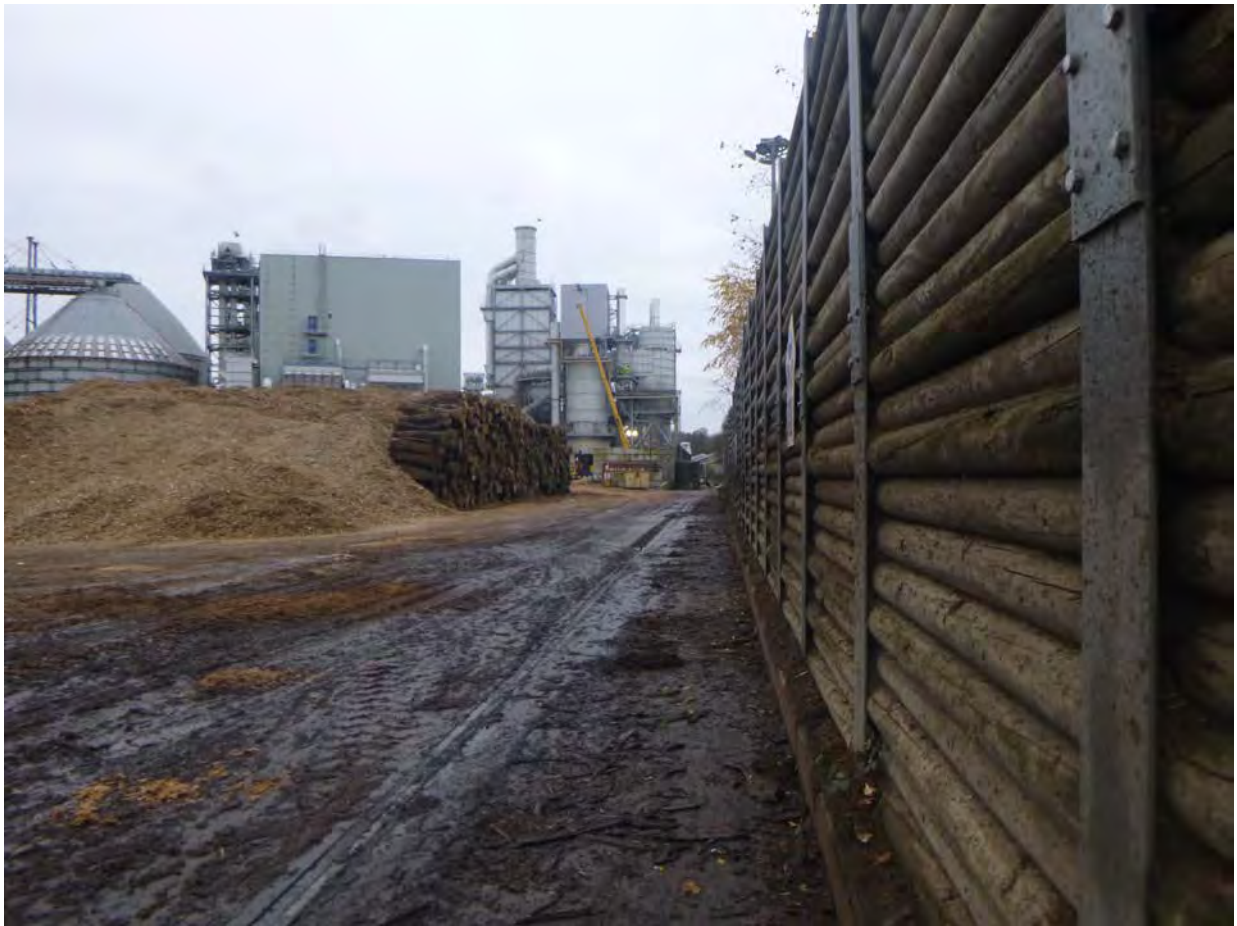
Plate 3. Existing silos and chip preparation building
